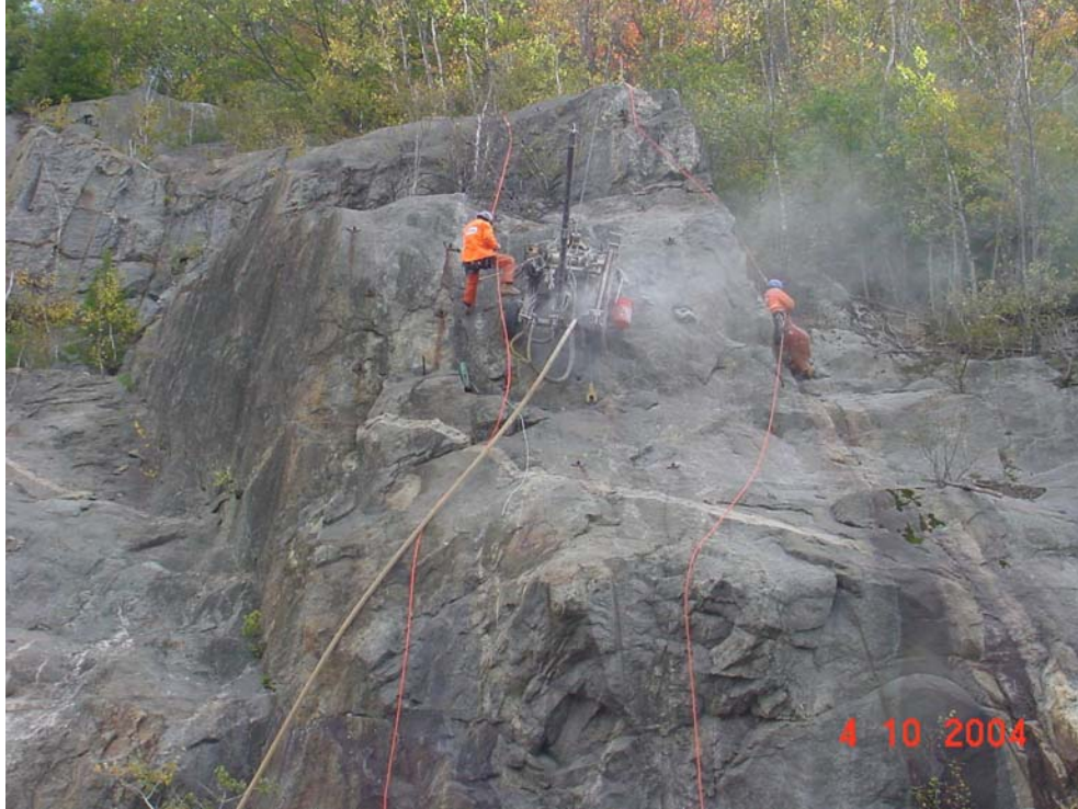
Figure 5. Drilling replacement holes for rock reinforcement
