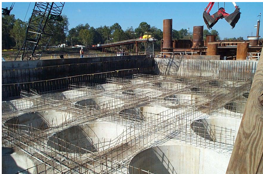
Clamming in between lifts of concrete at Pier 37
