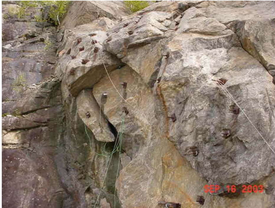
Figure 3. Pre-stressed, resin grouted rock bolts, center section
