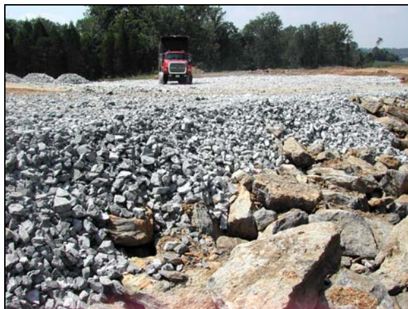
Figure 13. Same sinkhole with full treatment of graded rock embankment. Truck is on subgrade of roadway.
