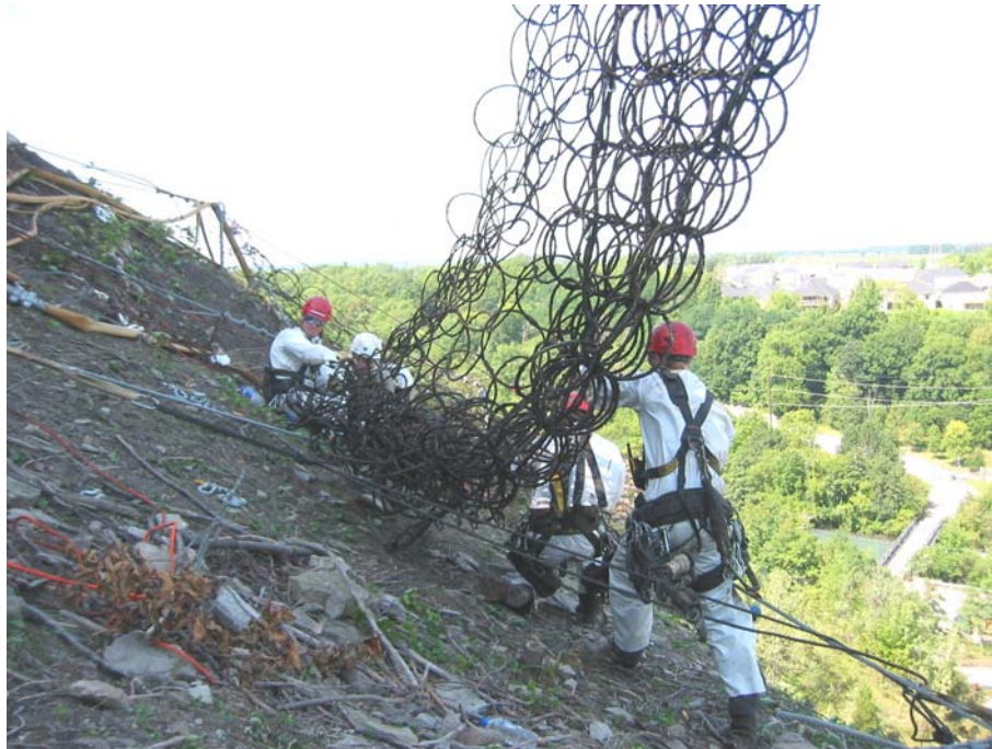
Figure 13. Ring net panel hanging from helicopter while ground crew attaches end of net to anchor cable.
