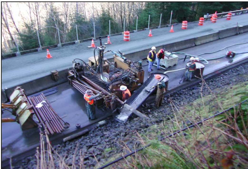
Figure 9c: Installation of horizontal drains and recently completed soldier-pile wall on an unstable slope above the Bogachiel River along SR 101 on the Olympic Peninsula.
