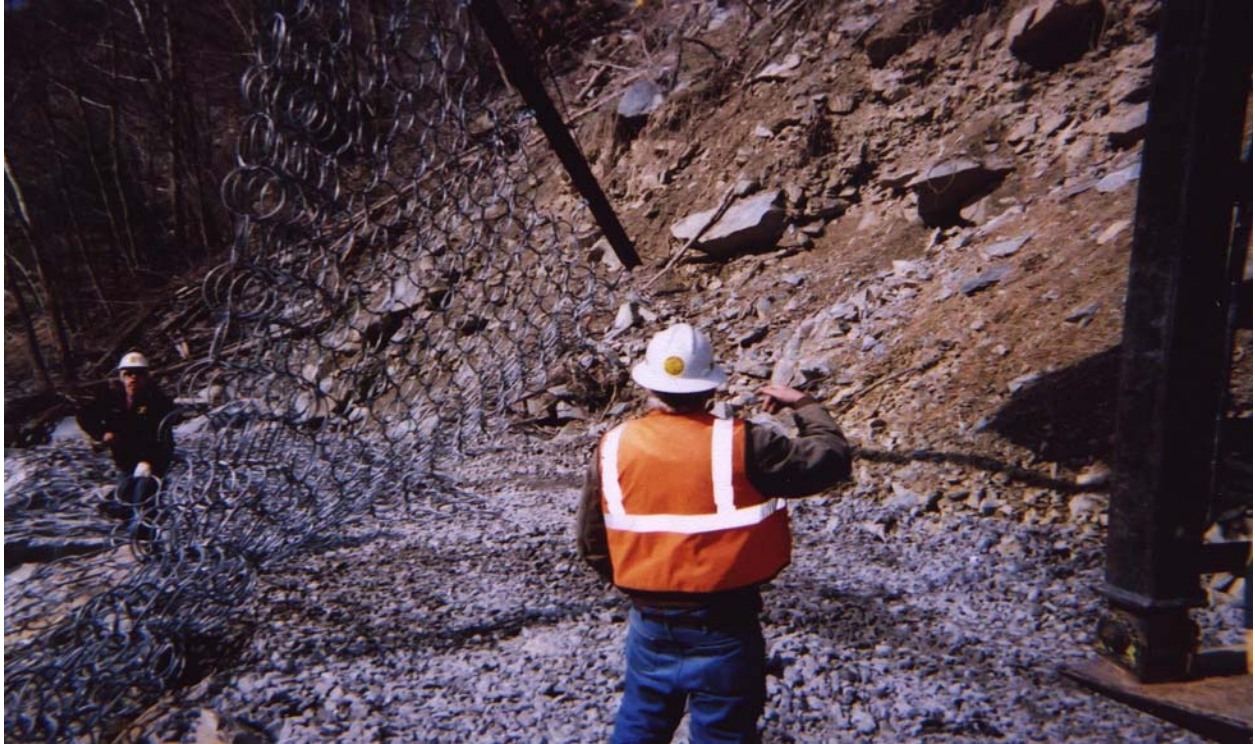
VIEW OF RING NET BEING POSITIONED
