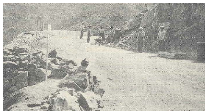
Figure 2. 1937 stone retaining wall construction (Clements 2003)
