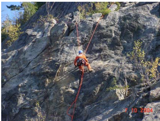
Figure 6. Hand scaling
