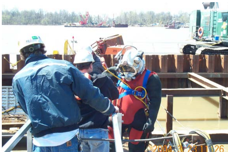
Diver Prepared to Enter Pier 38 Caisson
