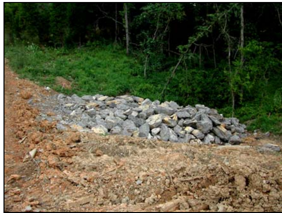
Figure 9. Same sinkhole with graded rock fill in lower lift of embankment.
