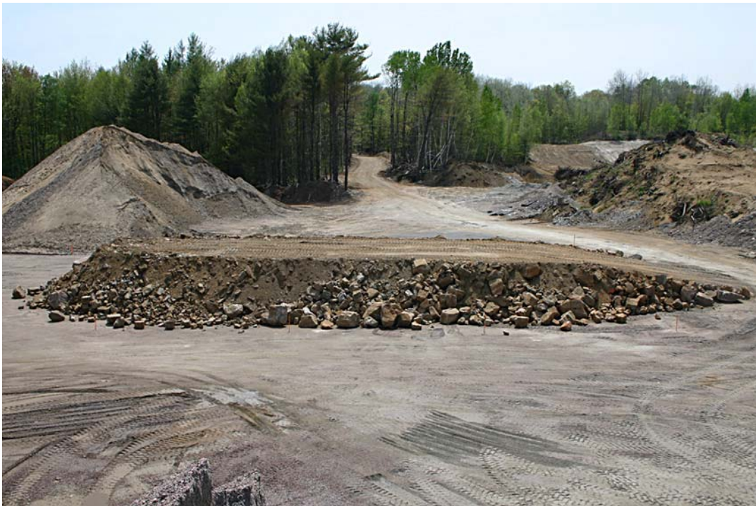
Figure 4. Partially constructed embankment at the Minden site.
