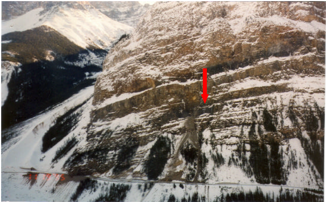
Figure 5: Rock fall November 17, 1995 – An estimated 3,200 to 4,000 cubic yards fell behind the lock-block wall under construction.
