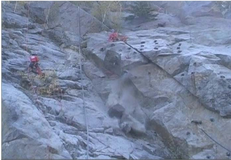
Figure 8. Splitting the detached block with the Boulder Buster™ device.
