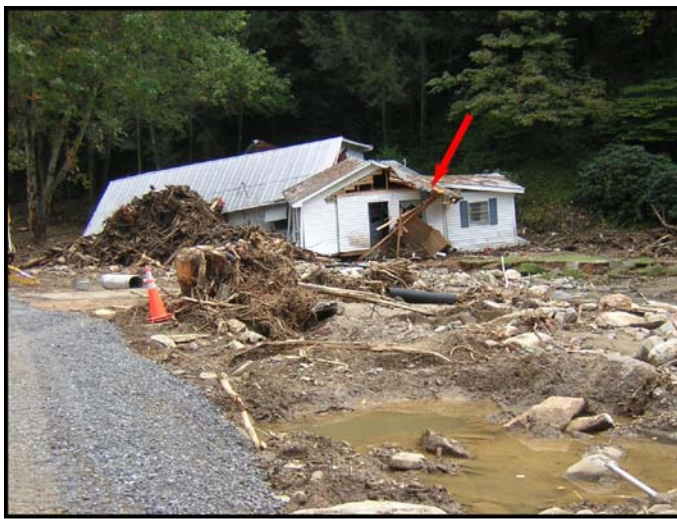
Figure 6. Photographs showing damage in the Peeks Creek community. Above, house indicated by arrow was moved 500 feet downstream by the debris flow. It stopped when it collided with the house on left. Right, contorted vehicle is all that remains at this location. Three people were killed here, and one was severely injured.
