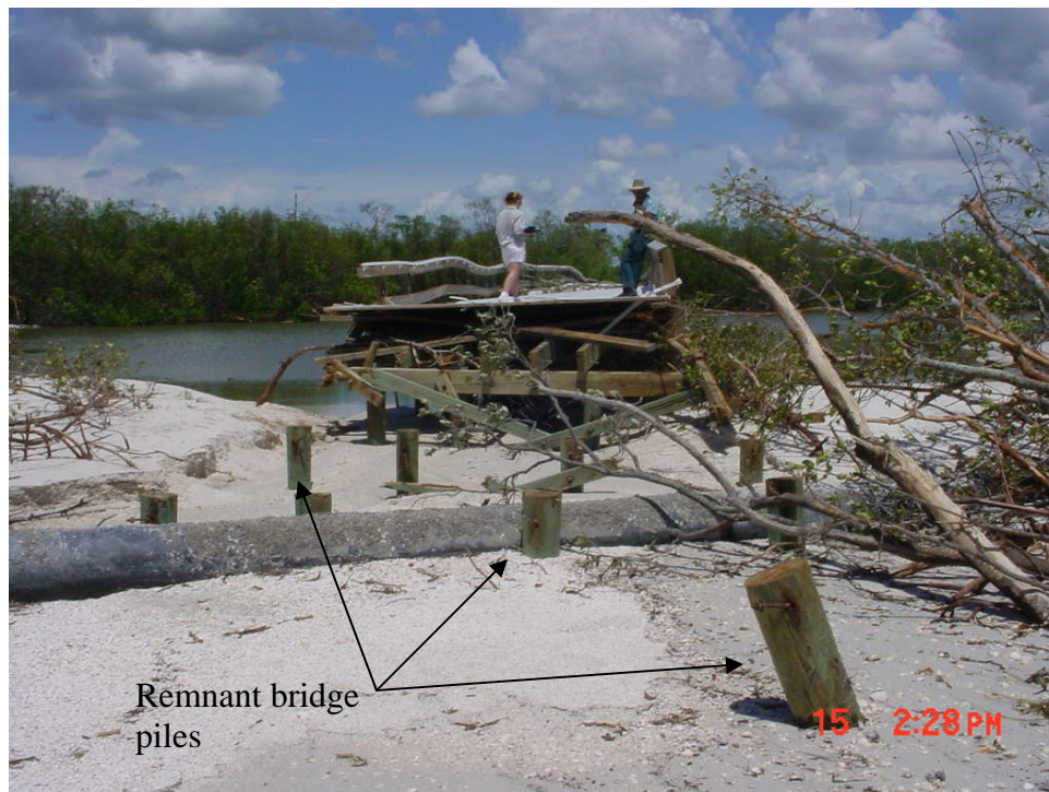
Figure 7: Wooden bridge damaged by hurricanes, Lovers Key, Lee County, FL. (Photo courtesy of Rob Neal, Lee County)
