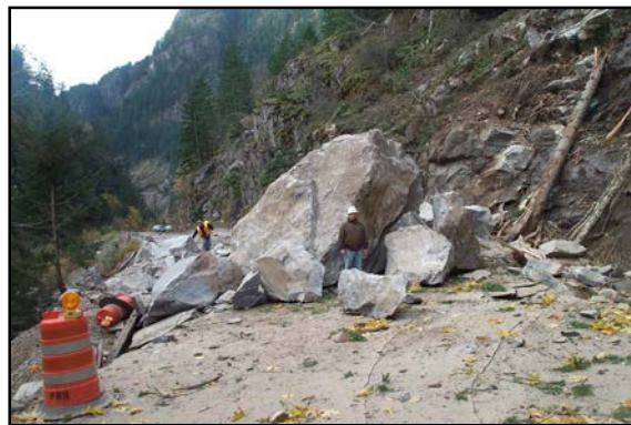
Figure 4: Rockslide at Falls Creek overtopping catchment area and highway along SR 20 North Cascades, Washington.
