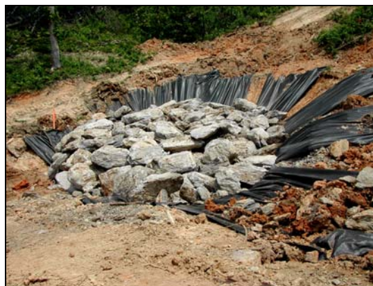
Figure 7. Typical sinkhole with graded rock placed onto the geofabric.
