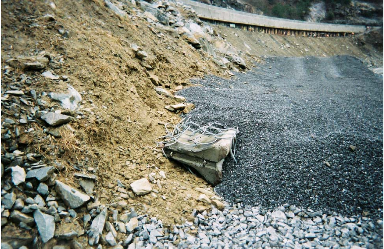
VIEW OF CONCRETE BARRIER WITH RING NET WRAPPED AROUND IT
