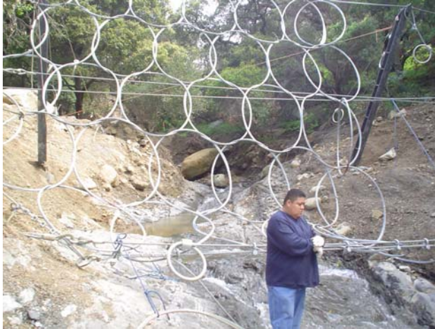
Fig. 21 - Whale net barrier in construction.
