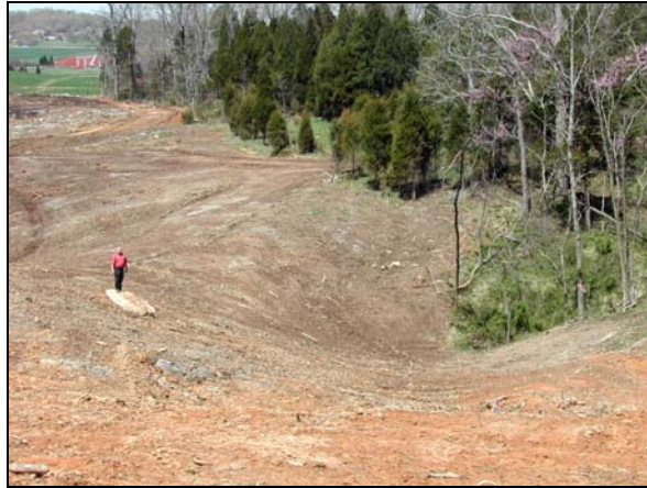
Figure 11. Typical sinkhole on SR 66 project, before treatment.
