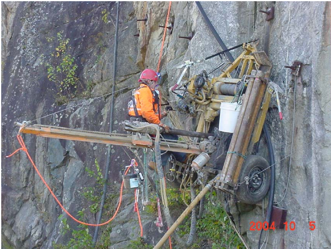
Figure 10. Air track drill with winch mounted on wagon
