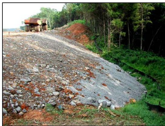
Figure 10. Same sinkhole with choker stone lift on top of larger graded rock material and common fill material placed on top of choker stone material. The choker stone aids in filtering runoff as it enters the sinkhole basin.
