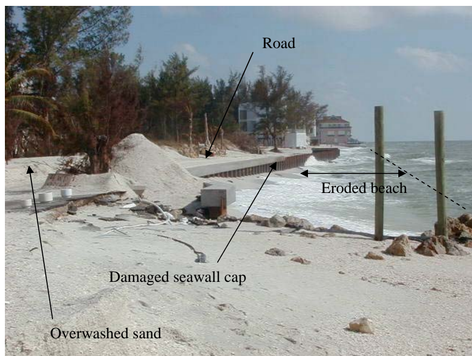
Figure 3: Seawall damage and eroded beach, Siesta Key, Sarasota County, FL. (Photo Courtesy of FDEP, 2004d)
