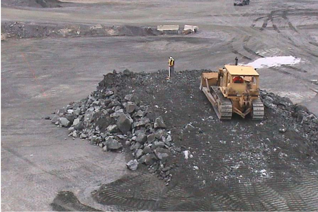
Figure 3. Building the embankment access ramp at the Parry Sound site.
