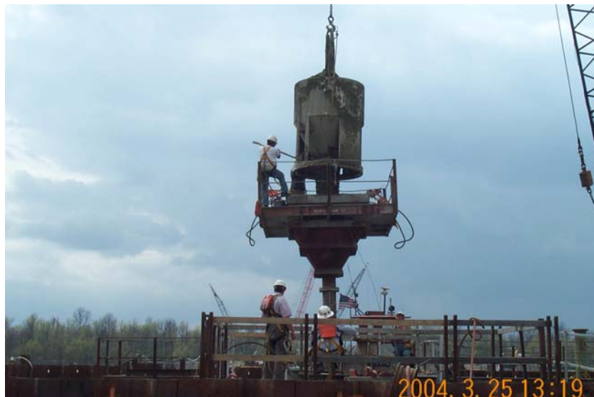
Placement of Seal Concrete
