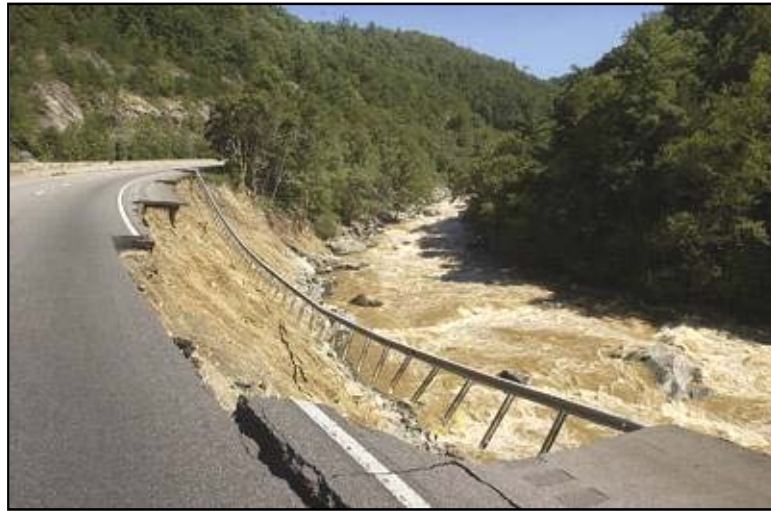
Figure 5 – Section of I-40 collapsing in September 2004 due to erosion of embankment by floodwaters in the Pigeon River from Hurricane Ivan.
