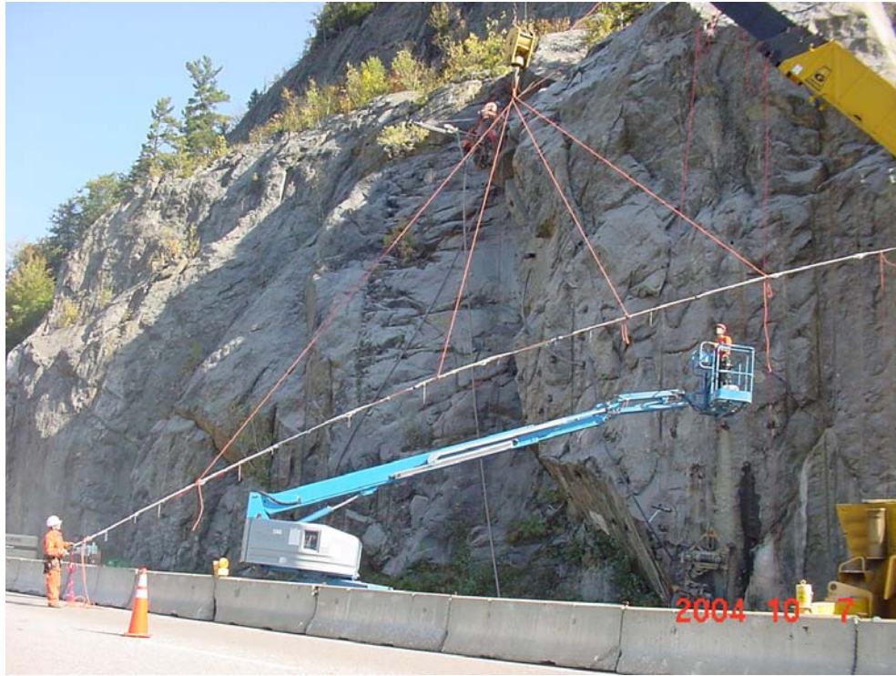
Figure 11. Installing 60-foot long steel tendon
