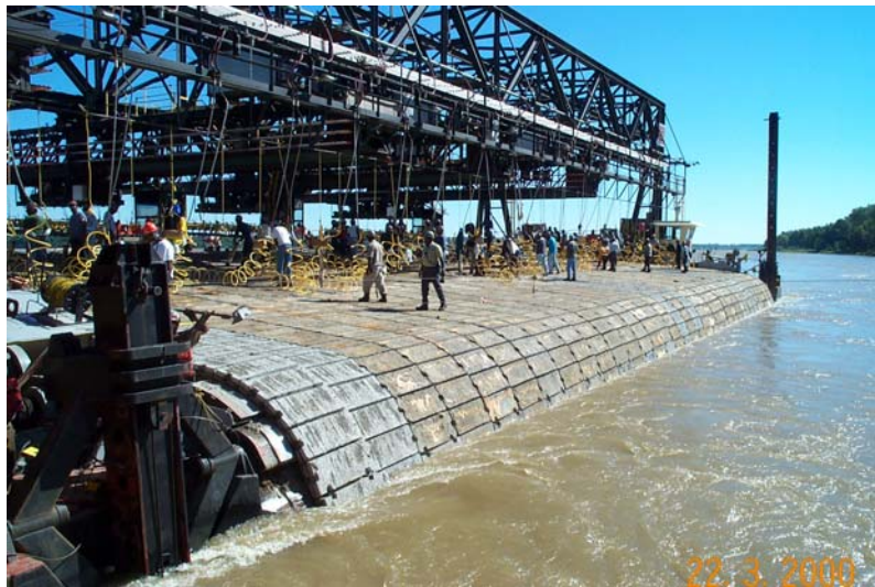
Installing Articulated Concrete Mattress Scour Protection
