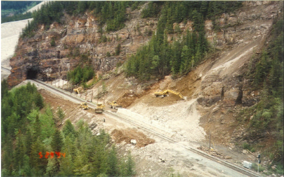
Figure 4: Rock fall May 26, 1994 – An estimated 3,200 cubic yards fell. Most was retained behind the existing 10 foot high lock-block wall. Cleanup took 26 hours.
