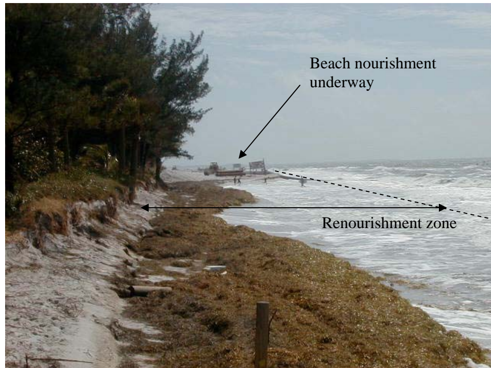
Figure 2: Beach Nourishment on Treasure Island, Pinellas County, FL (FDEP, 2004c).
