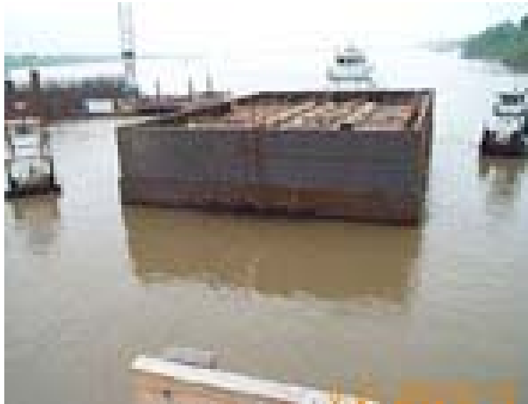
Float-in of Cutting Edge
