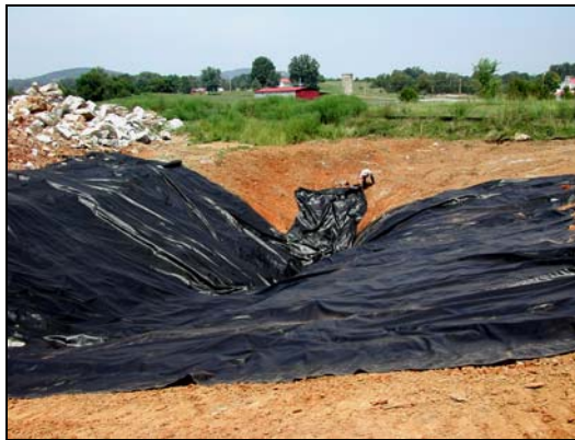
Figure 6. Placing the geofabric (geotextile) liner into the sinkhole (note man bending over in upper center of photo).
