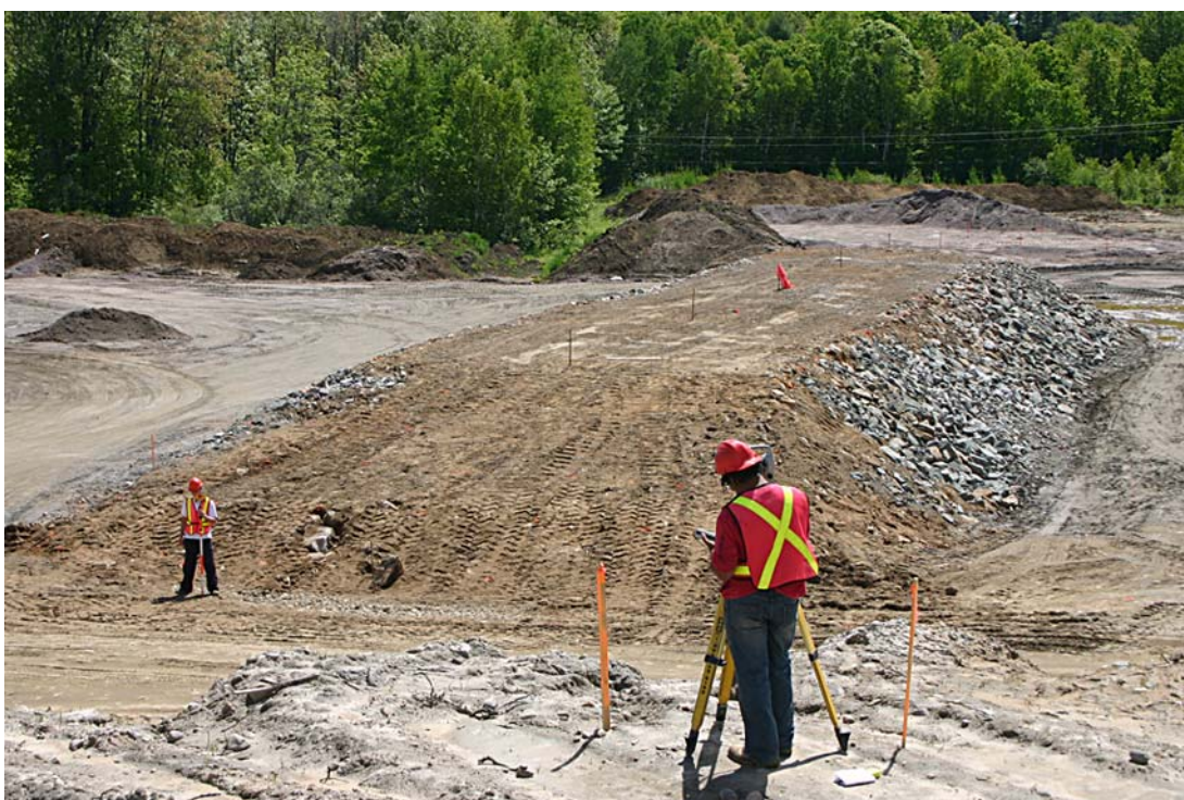
Figure 6. Surveying the embankment at Minden to determine volume of the fill.
