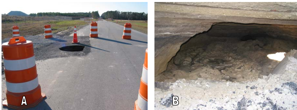
Figure 1. A- Sinkhole on Duffy Field Road that developed in December 2003, view west. B- Below ground view of sinkhole illustrating its lateral extent. The sinkhole is developed in Unit B of the Castle Hayne Limestone; overburden is at the top of the photo. Note the roadway asphalt.
