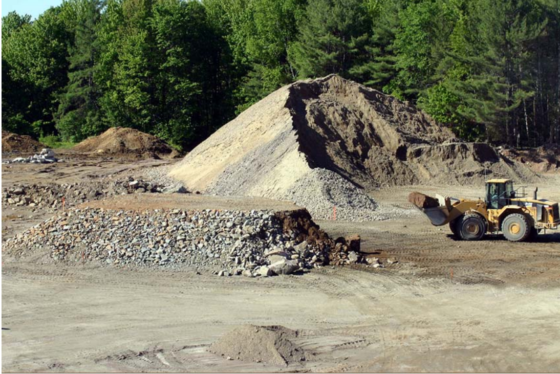
Figure 7. Removal and weighing materials at the Minden site to determine mass of the fill.
