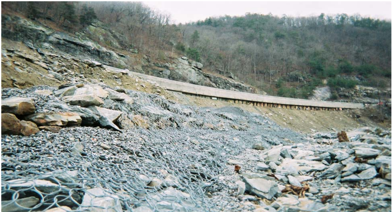
VIEW OF PARTIALLY COMPLETED TOE SCOUR SYSTEM AT SLIDE AREA 2
