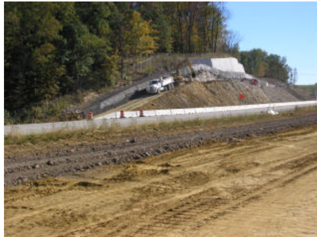
Photograph 3. Showing the Upper Soil Nail Wall and the Rock Nail Stabilization
