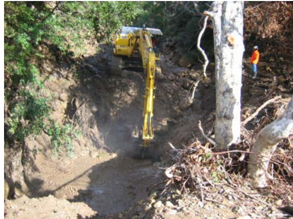
Fig. 17 – Cleanout of channel before whale net install. (Courtesy Duffy).
