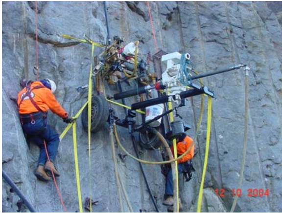
Figure 15. Over-coring (Janod Contractors)
