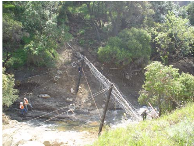
Fig. 20 - Whale net barrier side profile.
