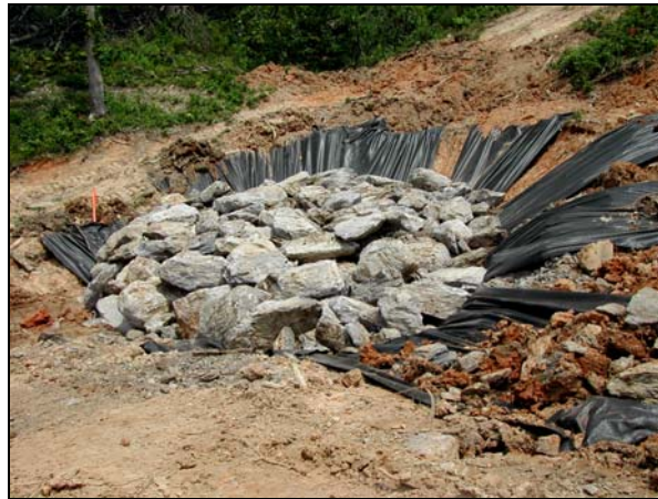
Figure 12. Same sinkhole with geofabric and graded rock fill material.
