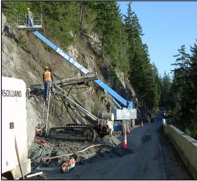
Figure 9a: WSDOT conducting an emergency repair of an unstable slope problem along SR 11 Chuckanut Drive in south Whatcom County, Washington.
