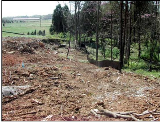
Figure 8. Typical sinkhole on SR 66 project, before placing graded rock embankment .
