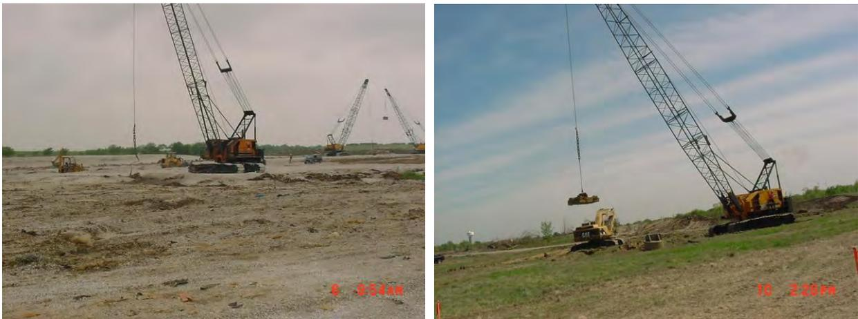
**Figure 18 – Deep Dynamic Compaction (Ironing Pass on right)**
