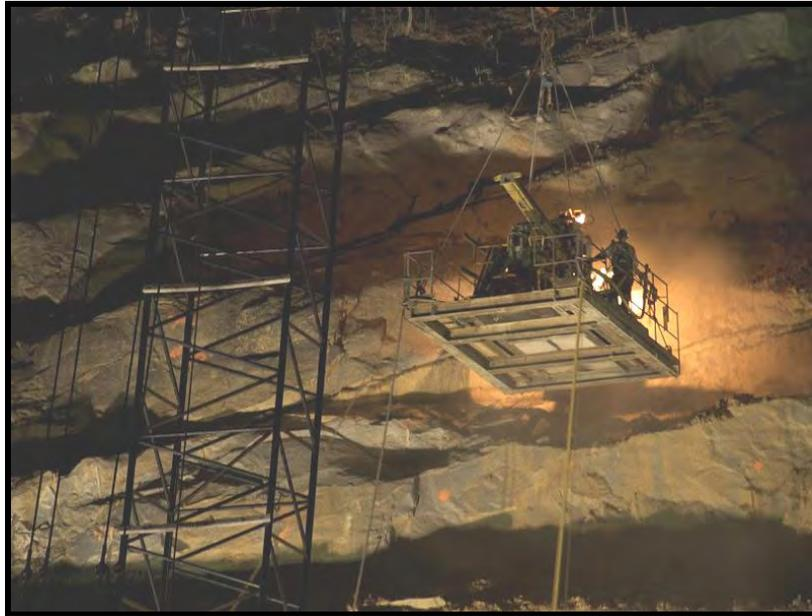
**Figure 12 – Night Drilling Pattern Rock Bolts Using Electric Drill Suspended by 275-Ton Crane.**
