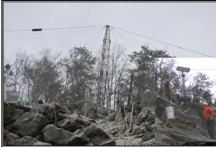
**Figure 11 - Tyrolean Hoist System, Inset - Moving a Jack**
