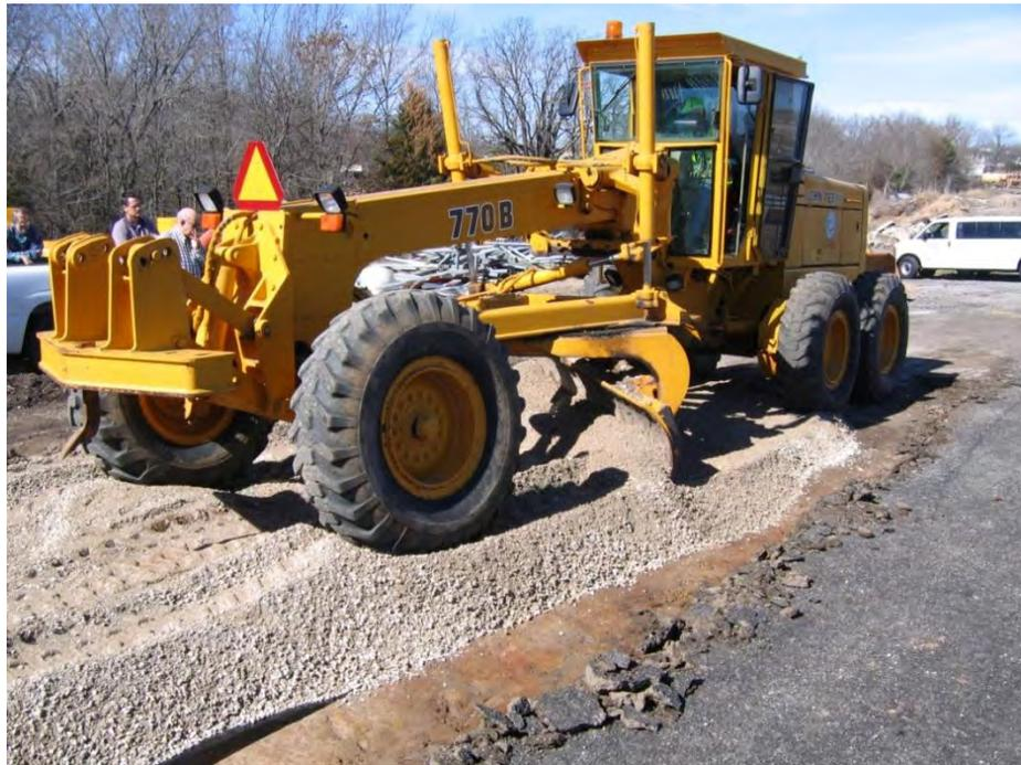
**Figure 6 – Blading the aggregate across the membrane**
