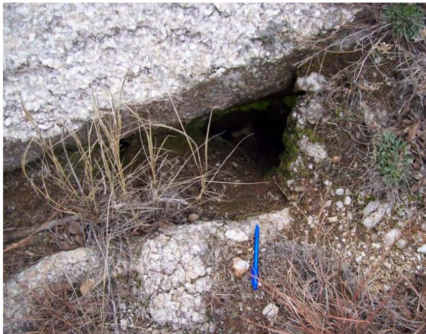
**Figure 2, Small Surface Void in Cut Section of HW-412**
