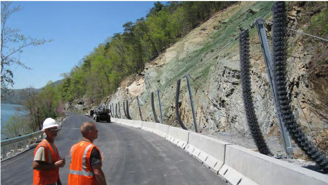
**Figure 6: Ongoing Installation of GBE Rockfall Barrier, Ocoee, TN**
