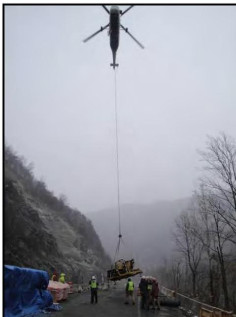
**Figure 9 - CH-53 Lifting Grout Plant**
