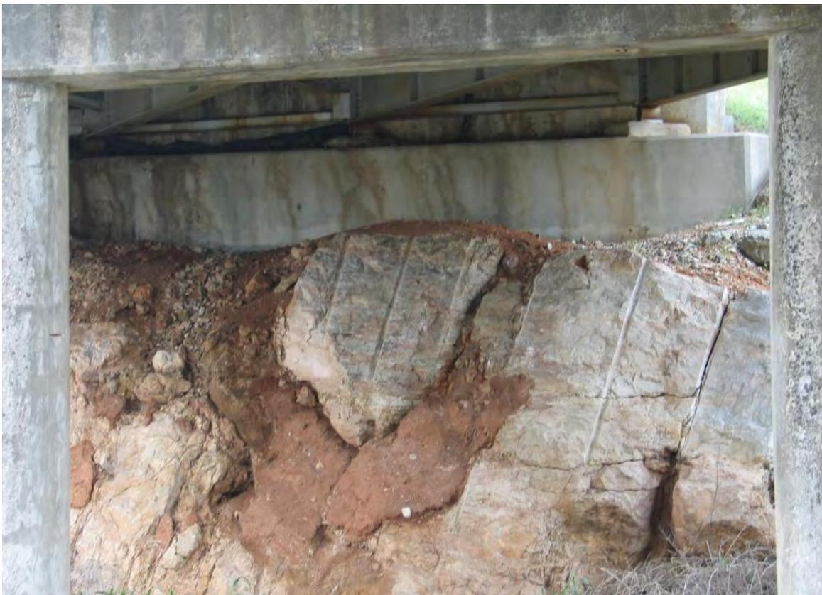
Fig. 3. South bridge abutment of northbound I-35 bridge over U.S. Highway 77, and blocks of Royer Dolomite filled in with red, clay-rich sediment.
