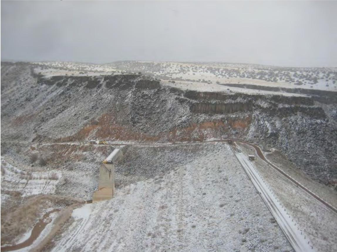
**Figure 5: Installed GBE Rockfall Barrier, Jemez Dam, NM**
