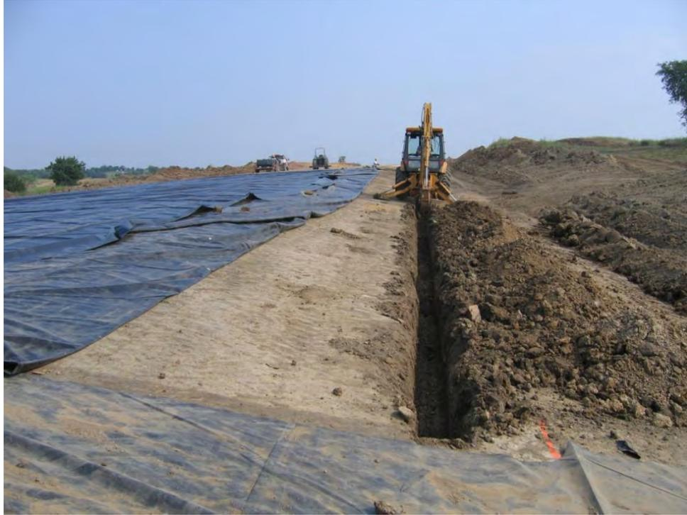
**Figure 12 – Trenching for pipe underdrain**
