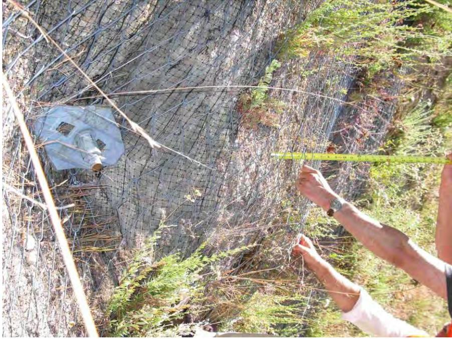
**Figure 5.** Non-uniform pressure between two short distances nails using high performance single-twist mesh.
