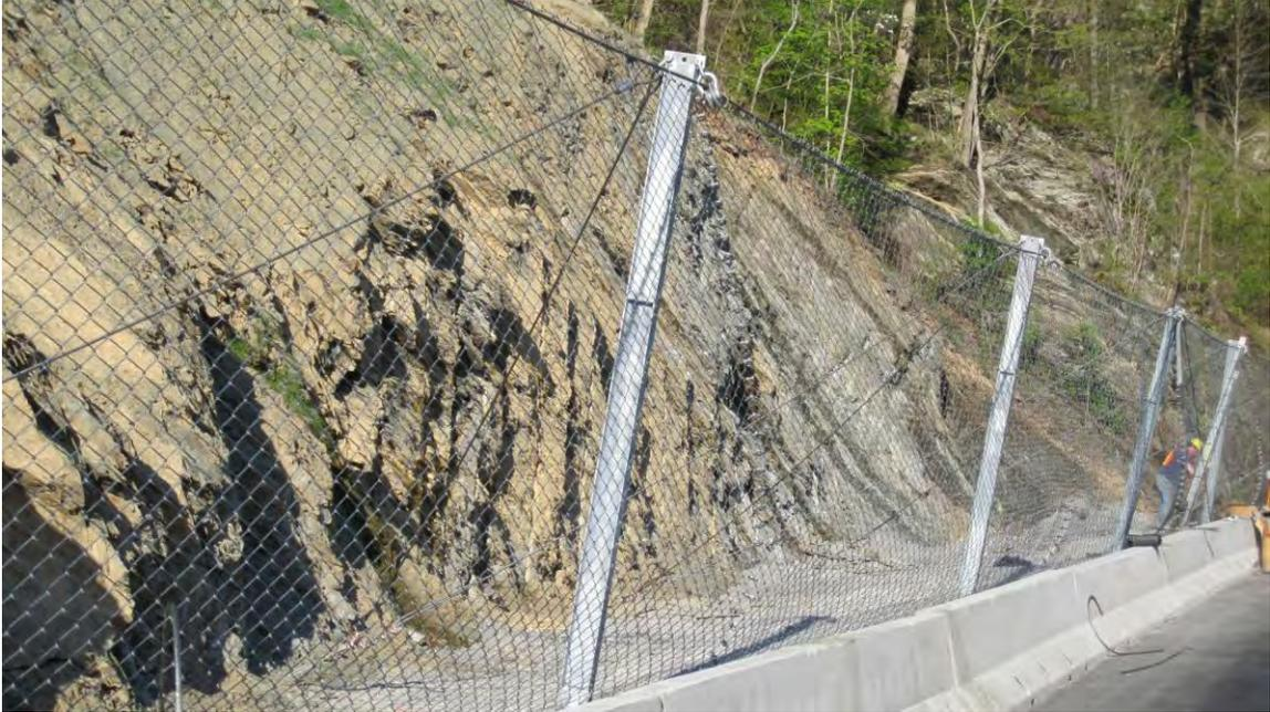
**Figure 7: Installed GBE Rockfall Barrier, Ocoee, TN**
