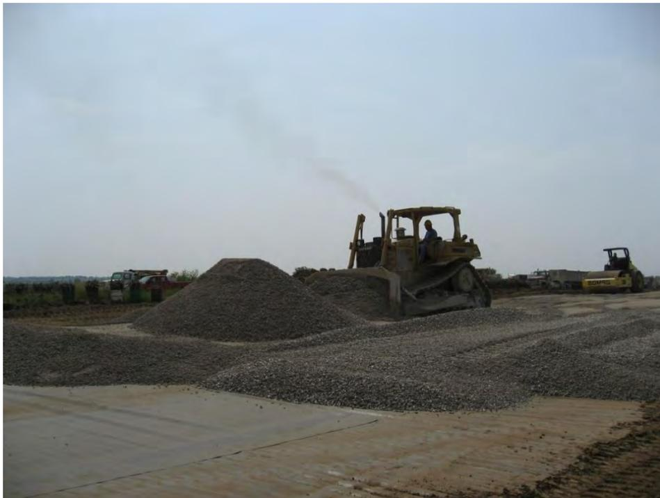
**Figure 15 – Spreading the crushed aggregate**
