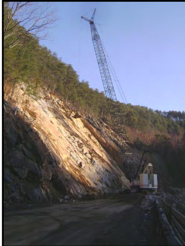
**Figure 5 – Mechanical Scaling Using Pygmy Excavator with Hoe-Ram Suspended From 275-Ton Crane. View to East (Photograph Date January 19, 2010).**
