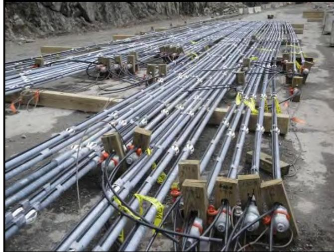
**Figure 12 - Rock Bolt Fabrication and Staging**
