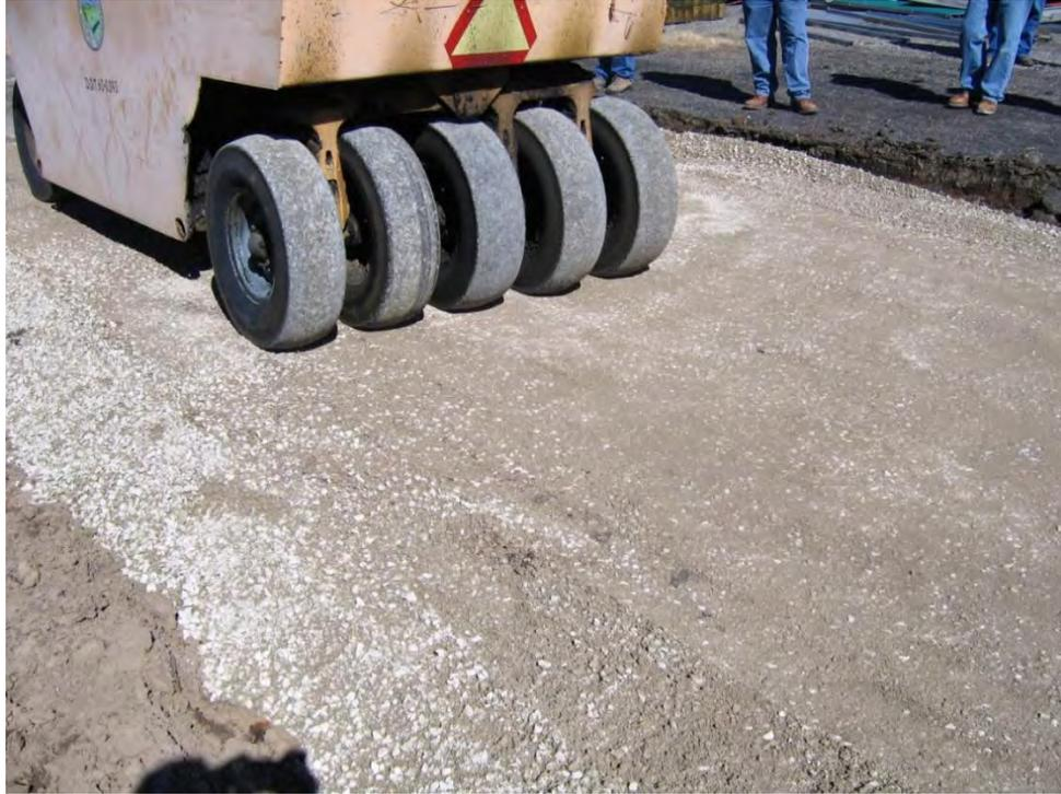
**Figure 7 – Compacting the crushed aggregate**
