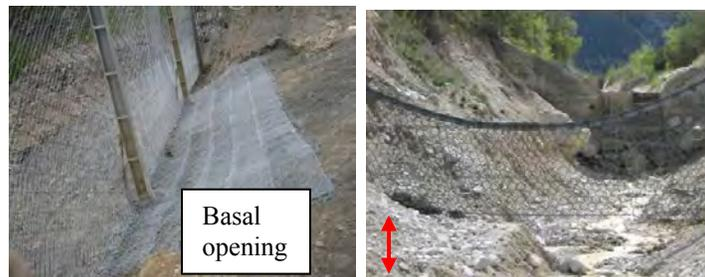
Figures 15 & 16. Particular ground adaptation with a fixed mesh for shallow landslide barriers (left) and extra projected basal openings for debris flow barriers (right)
