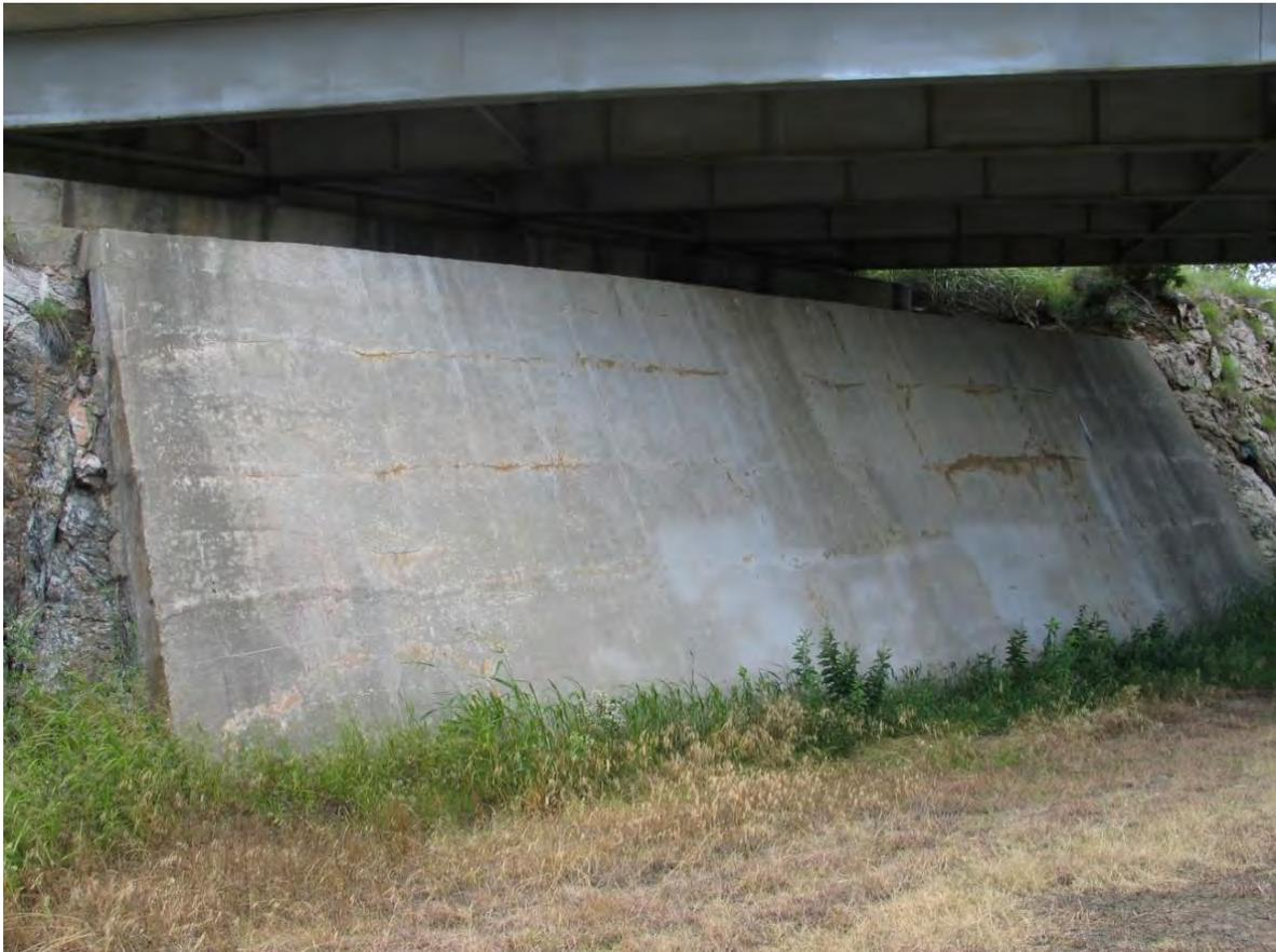
Fig. 4. Slope wall used to retain the clay and loose rock at the northbound bridge abutment.
