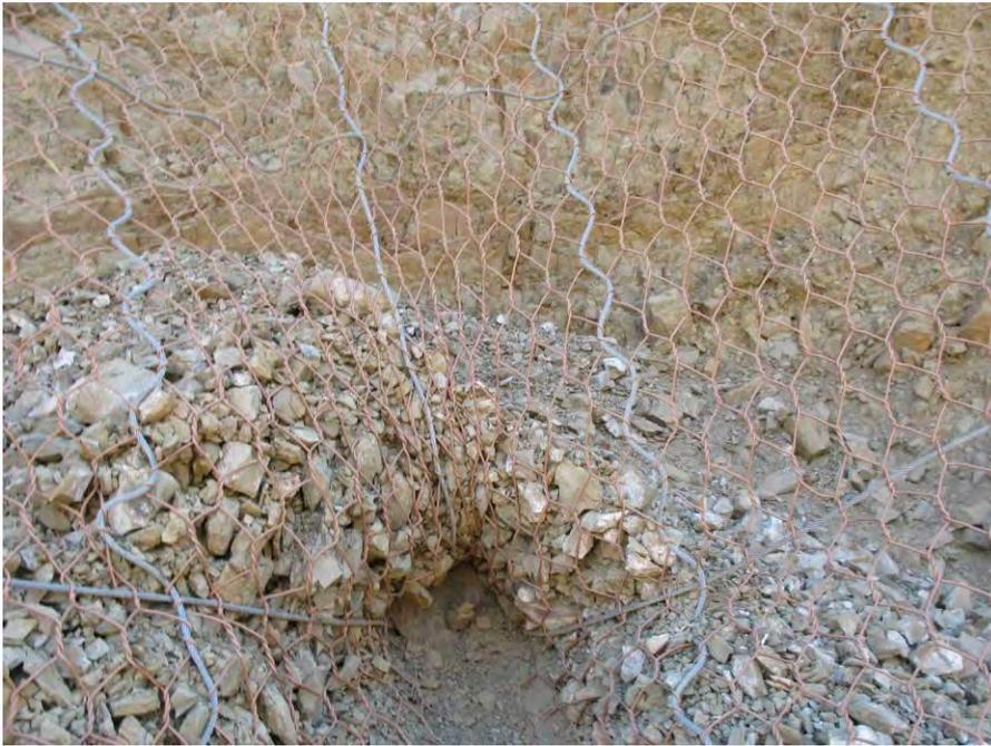
**Figure 9.** Debris accumulation contained by the soil nailing system with the steel cables inserted with RockMesh is transferring efficiently the load from the rocks to the anchors. .
