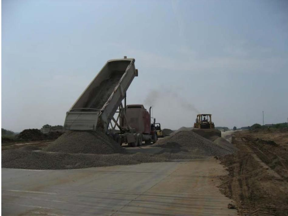
**Figure 14 – End dumping the crushed aggregate. Construction equipment was prohibited from driving on the membrane**
