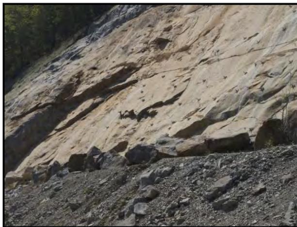
**Figure 10 – View from the Boat Ramp of Rock Bolts and “Guard Rock” Left as the Natural Transition Between the Slope and Pedestrian Walkway.**
