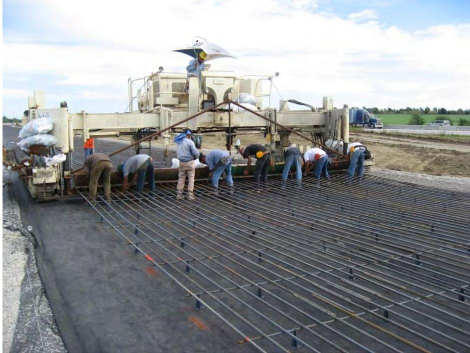
**Figure 20 – Tying the steel reinforcement**
