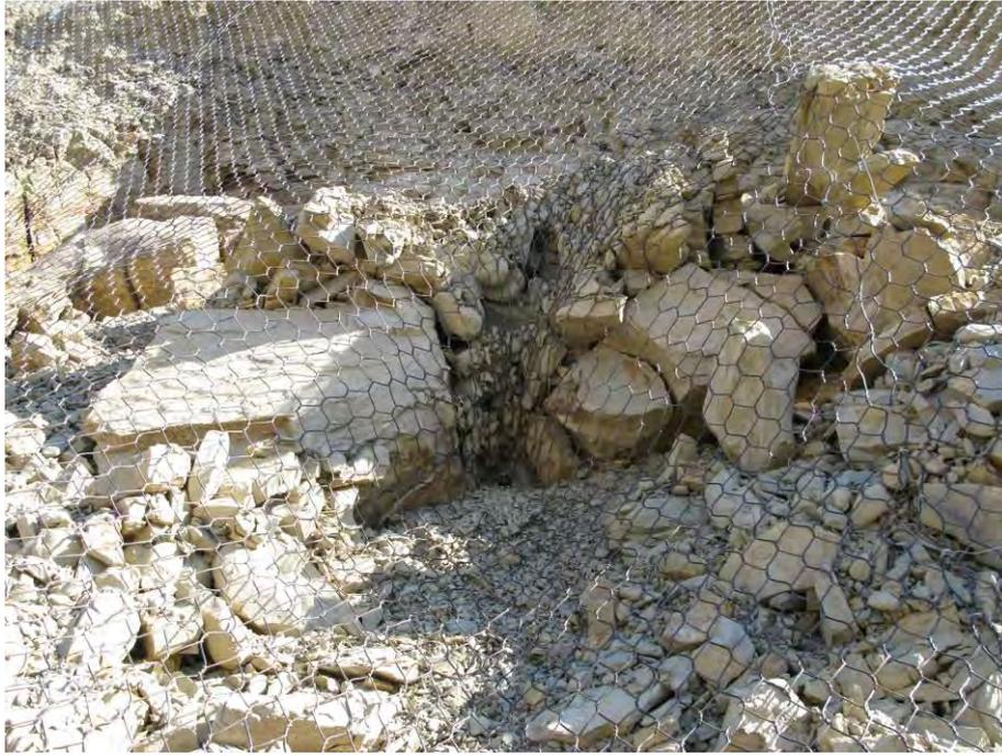
**Figure 11.** Excessive debris accumulation
