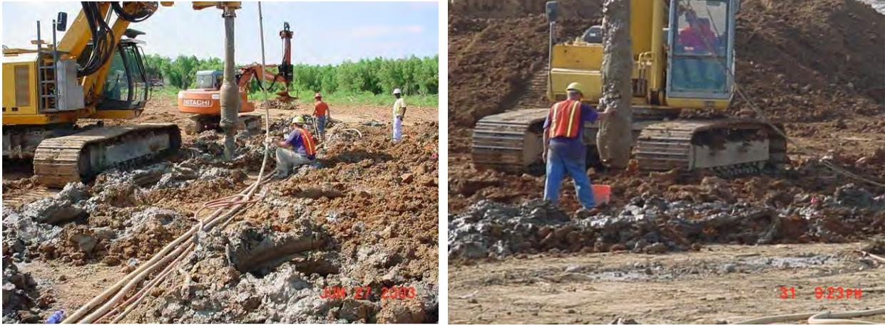
**Figure 17 – Deep Soil Mixing – Soil Cement Columns**
