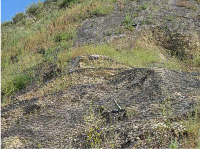
**Figure 1.** Unlevel slope facing with soil nailing
