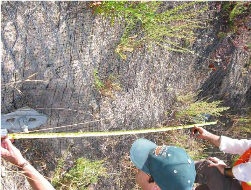
**Figure 4.** Distance of 2.1 m (7 ft) between anchors
