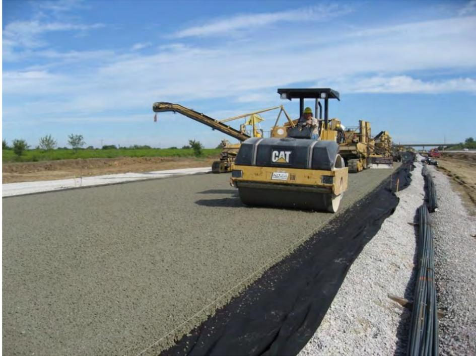
**Figure 18 – Compacting the open graded base layer**
