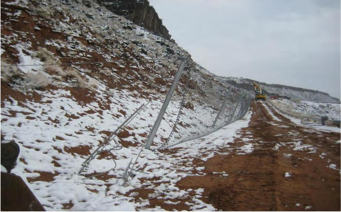
**Figure 4: Installed GBE Rockfall Barrier, Jemez Dam, NM**
