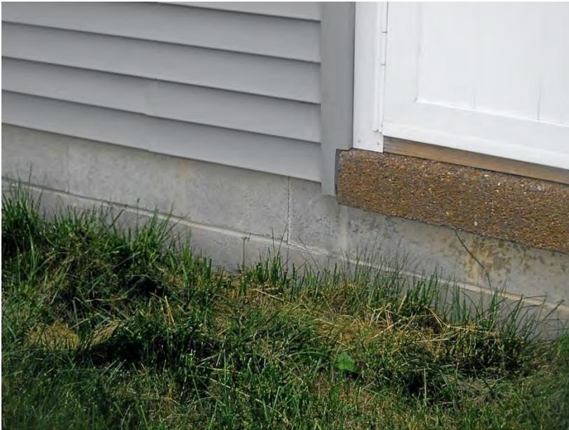
Figure 11. Exterior block wall with cracks in mortar joints, Meadowlake Hills Road residence.
