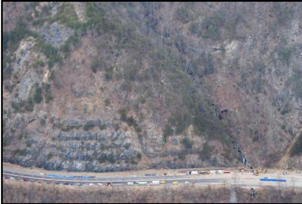
**Figure 2 - Benched Rock Cut Adjacent to Slide**
