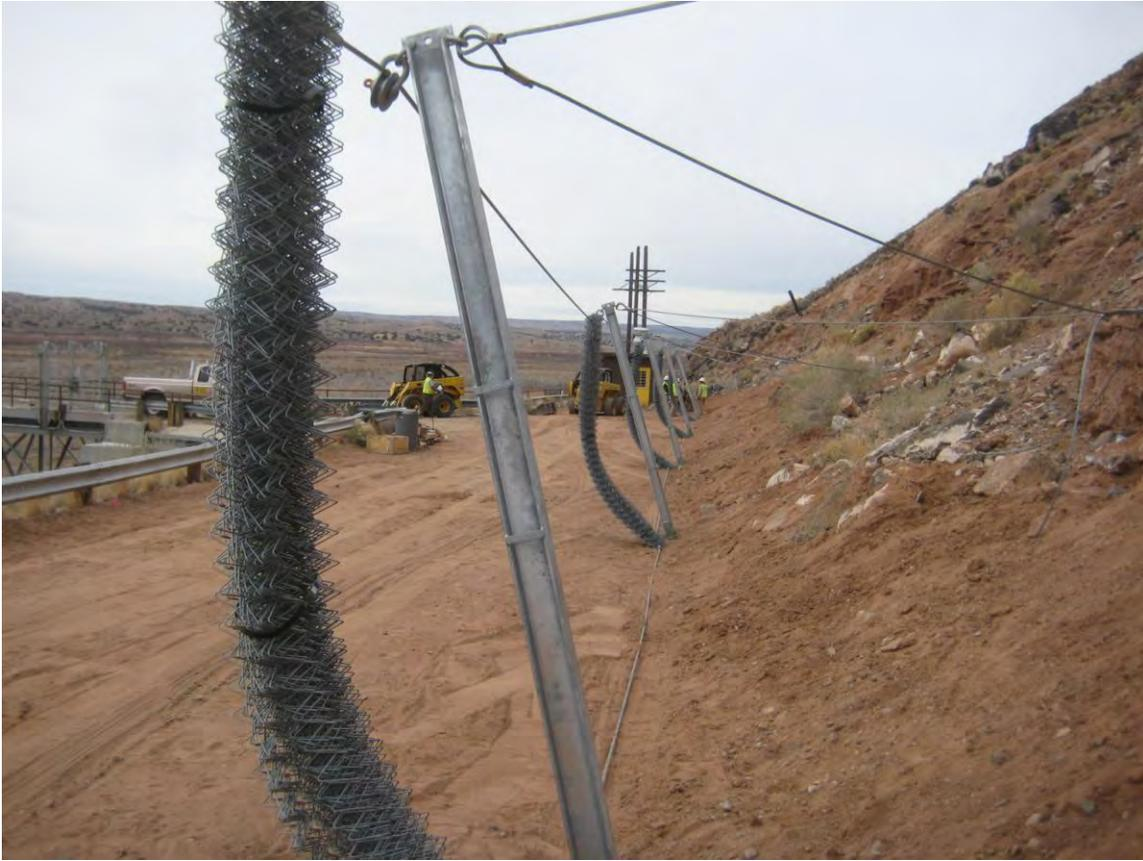
**Figure 2: X-Sectional View of Construction - GBE Rockfall Barrier**
