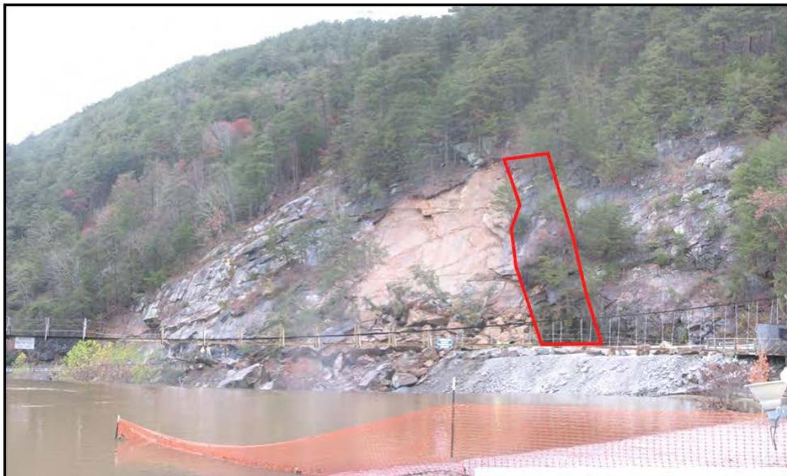
**Figure 6 – View of "Evil Twin" on Right (East) Side of Rockslide Scar Outlined in Red (Photograph Date November 10, 2009).**
