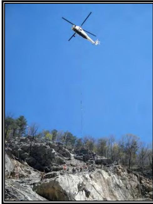
**Figure 14 - CH-53 Installing a Ground Anchor**
