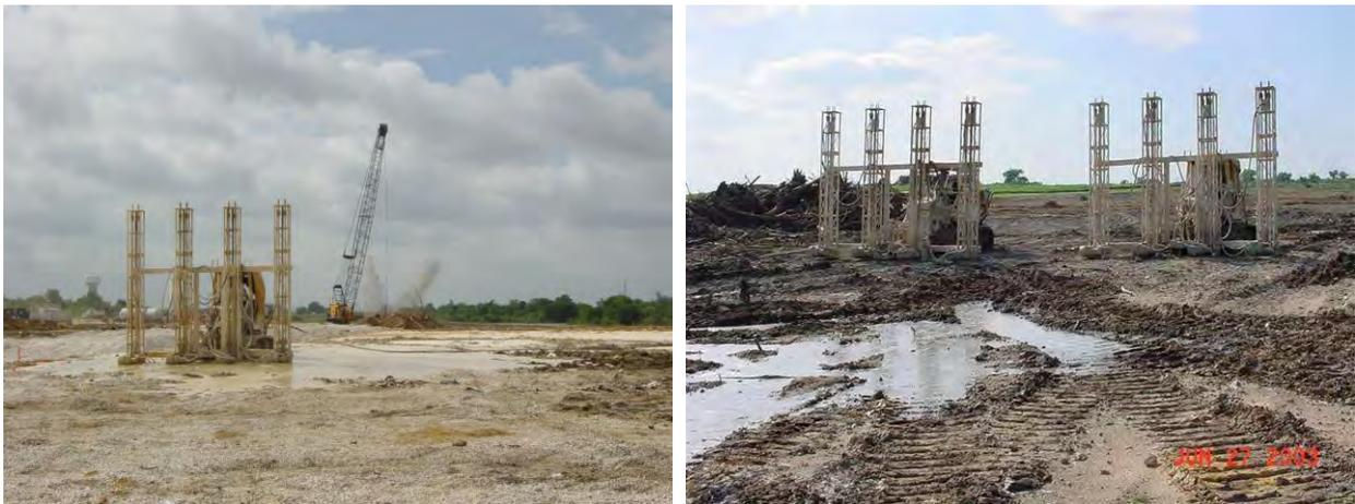
**Figure 19 – Lime-Fly Ash Injection (DDC in background on left)**
