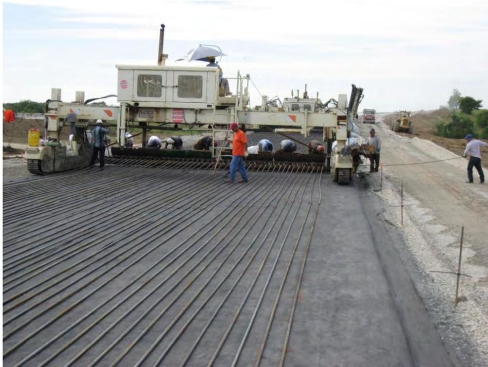
**Figure 19 – Placing the steel reinforcement for the CRCP, another layer of non-woven geotextile was placed upon the open graded base**
