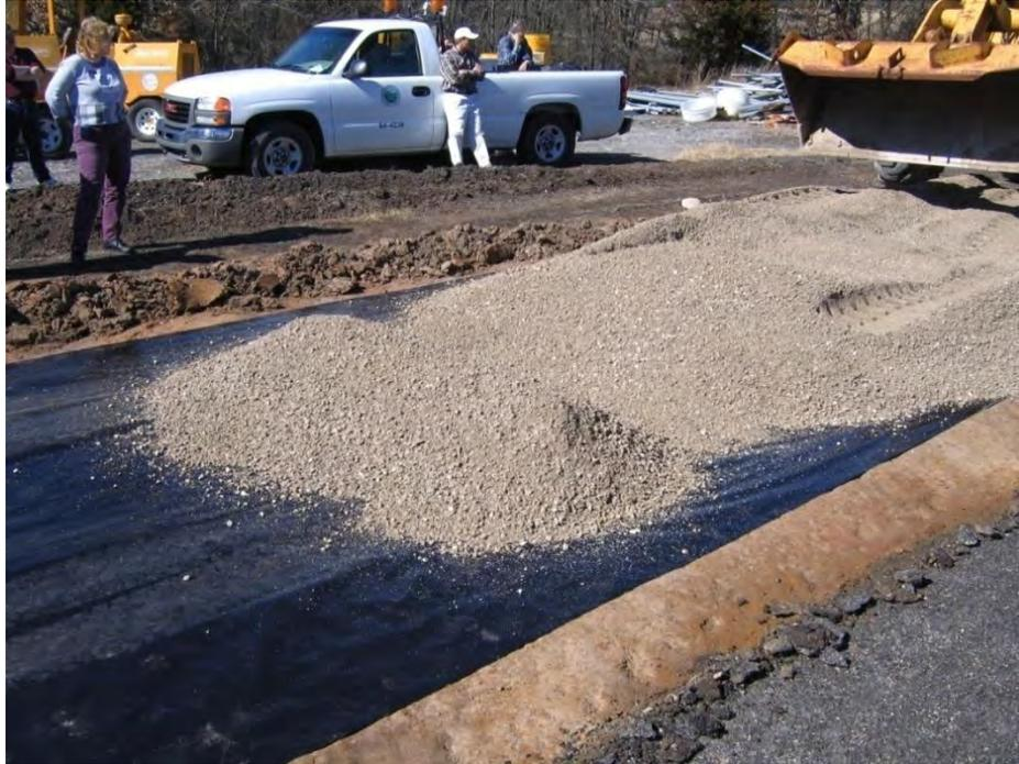
**Figure 5 – Field Test of Proposed Moisture Barrier, spreading the crushed aggregate**
