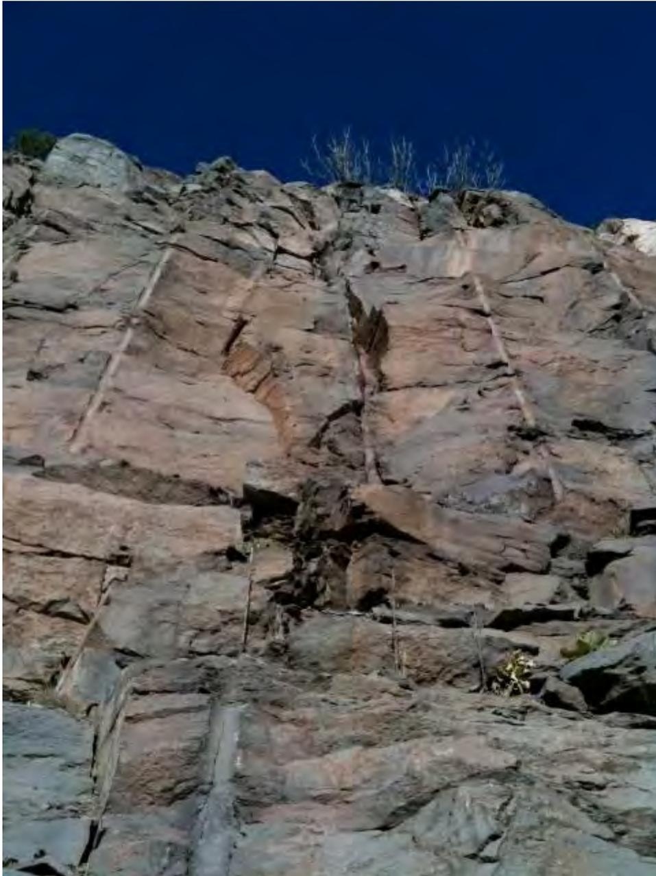
**Figure 5. Picture of the part of the Section 2 rock slope showing pre-split half-casts and some natural fractures sub-parallel to the slope.**
