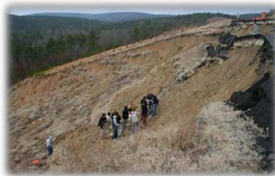
**Figure 1 – A massive highway slope failure in Latimer County, Oklahoma**
