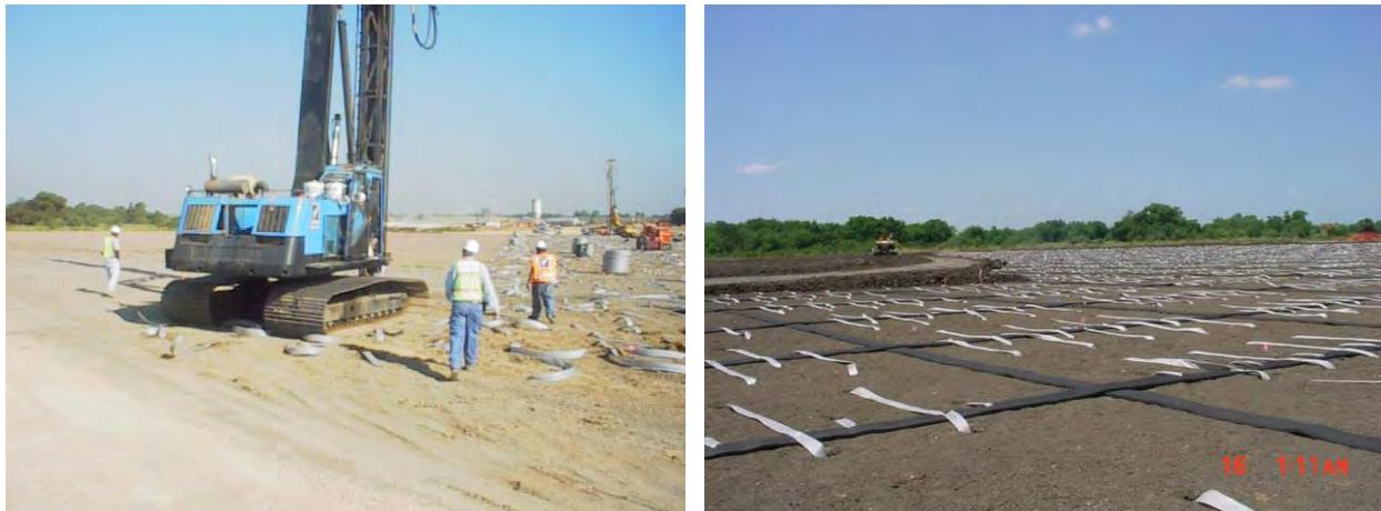
**Figure 16 – Vertical Wick Drain Construction**
