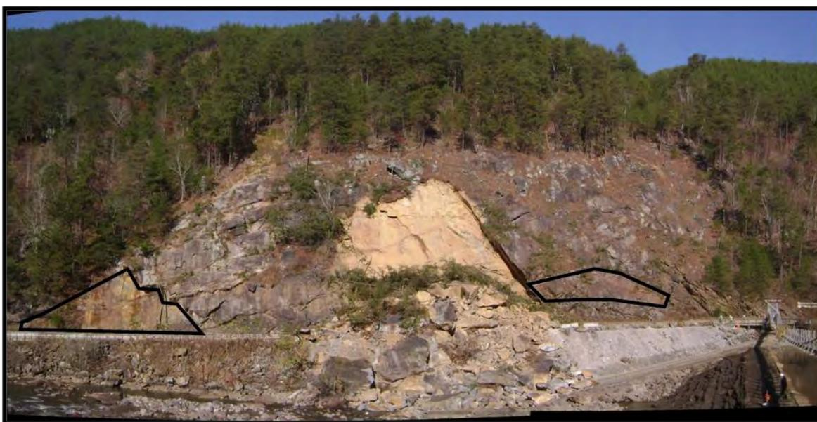
**Figure 7 – View of "Evil Twin" on Right (East) Side of Rockslide Scar. Areas outlined in black are apparent older slide scars on rock face more than 40 years old. TVA dam in lower right, including placement of crack gauges (photograph date November 20, 2009).**
