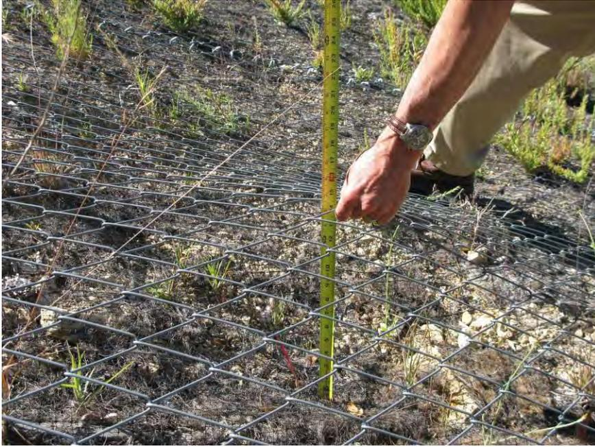
**Figure 3.** Photos of flexible mesh facing high performance single-twist mesh.
