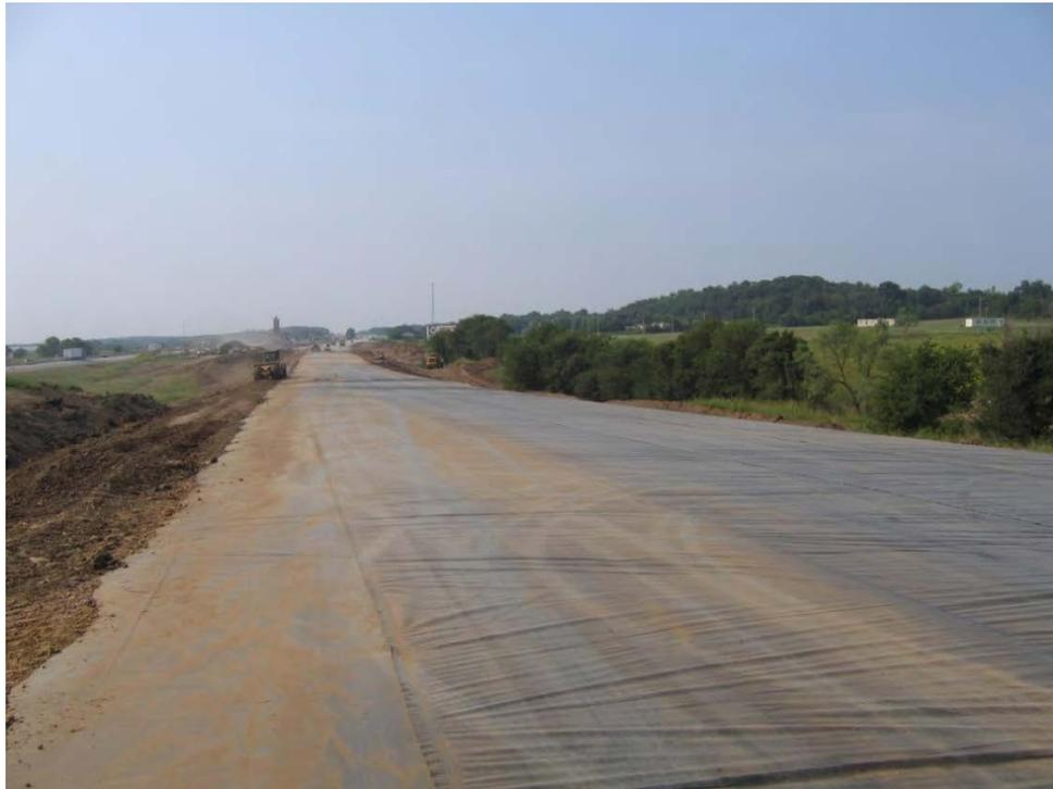
**Figure 13 – Moisture barrier placed across the grading section**
