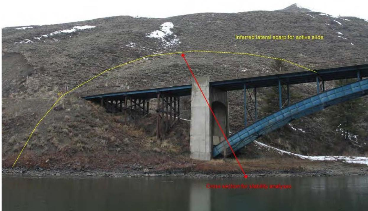
**Figure 5 – Inferred “Active” Landslide at West Abutment**
