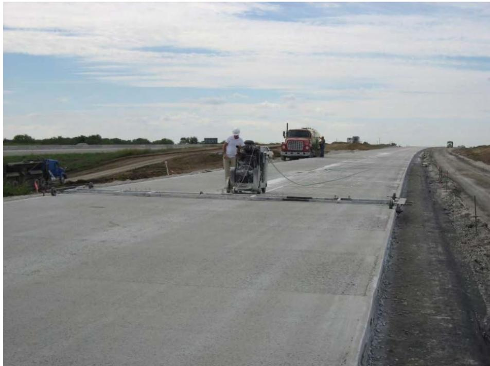
**Figure 21 – Sawing control joints in the new pavement**
