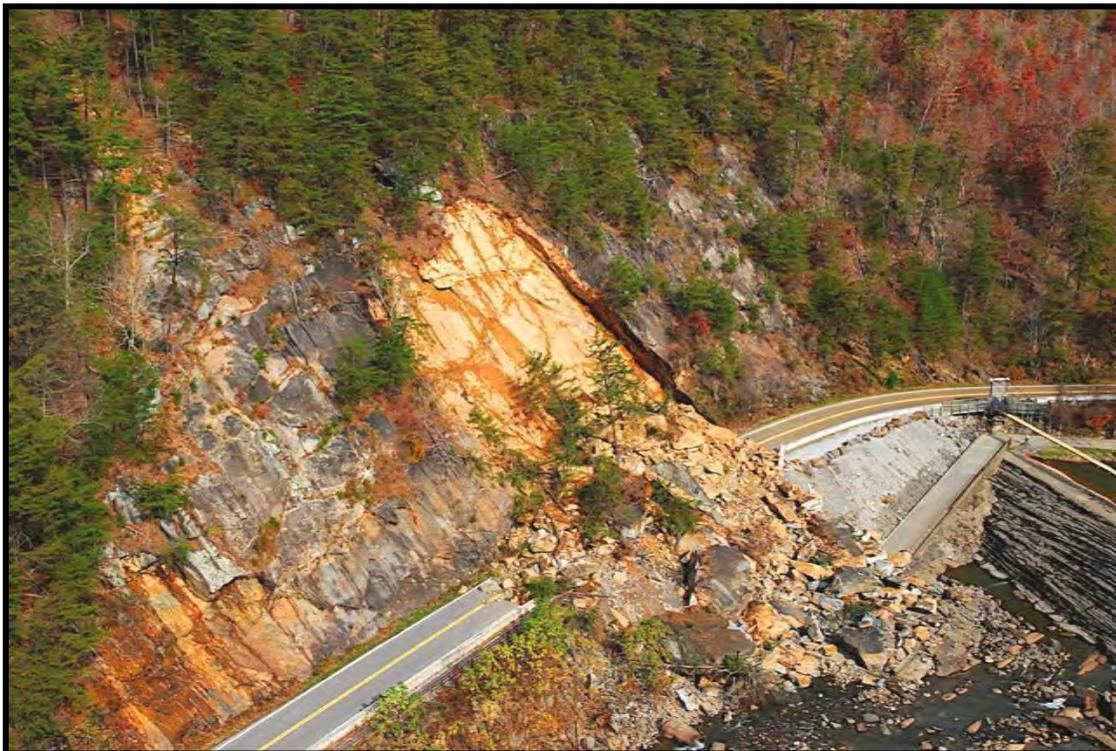
**Figure 2 – Aerial Photograph of the Rockslide on November 15, 2009. Note TVA Dam and Partially Buried Whitewater Raft Put-In on Lower Right. View to the Northeast.**
