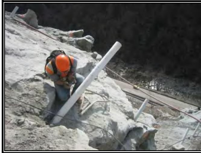
**Figure 10 - Checking Anchor Hole Orientation**
