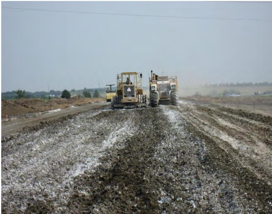
**Figure 11 – Lime Stabilization operations**
