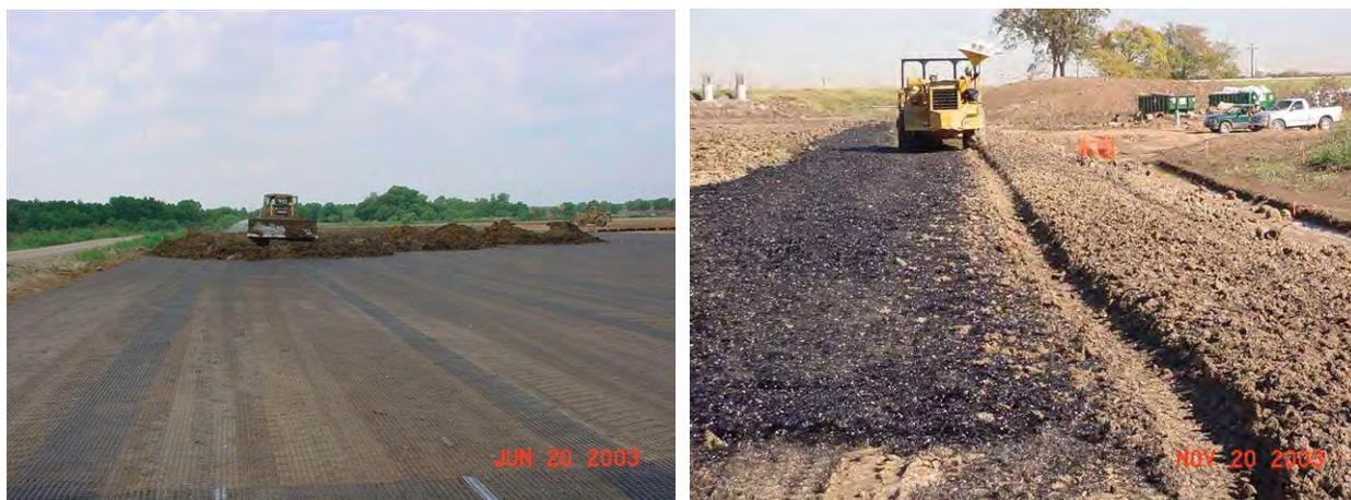
**Figure 21 – Biaxial Geogrid (left) and Fiber Reinforced Soil (right)**
