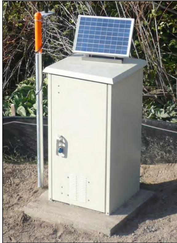
**Figure 3 – Typical ADAS Enclosure**
