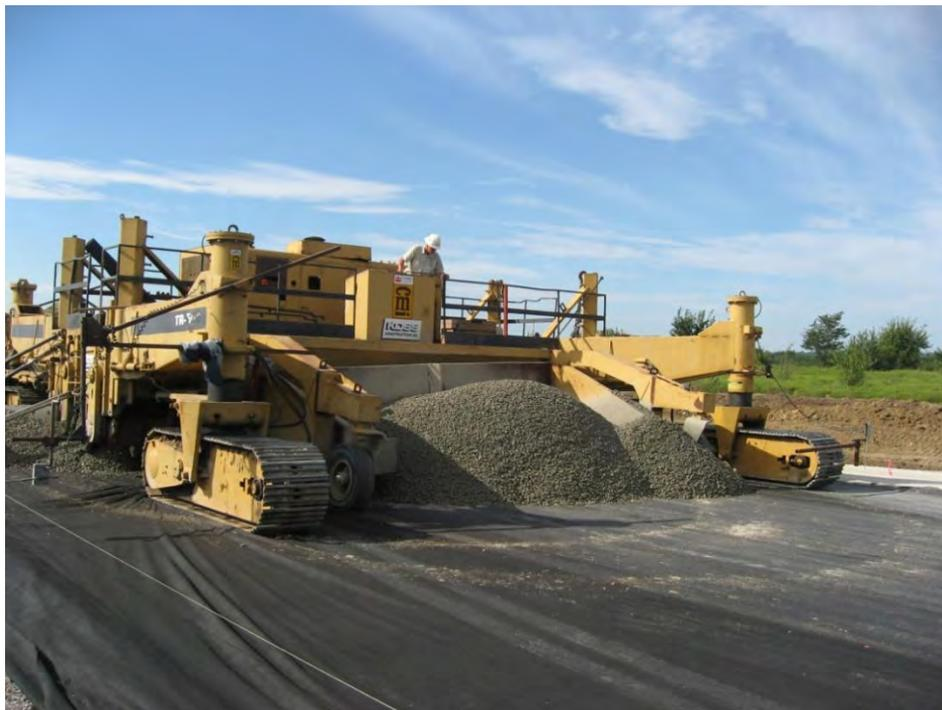
**Figure 17 – Placing the open graded base on top of the crushed aggregate base. A non-woven geotextile separates the two layers**
