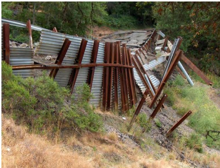
**Figure 1 - Failed Tied-back H-beam Retaining Wall and Roadway Due to Landsliding.**
