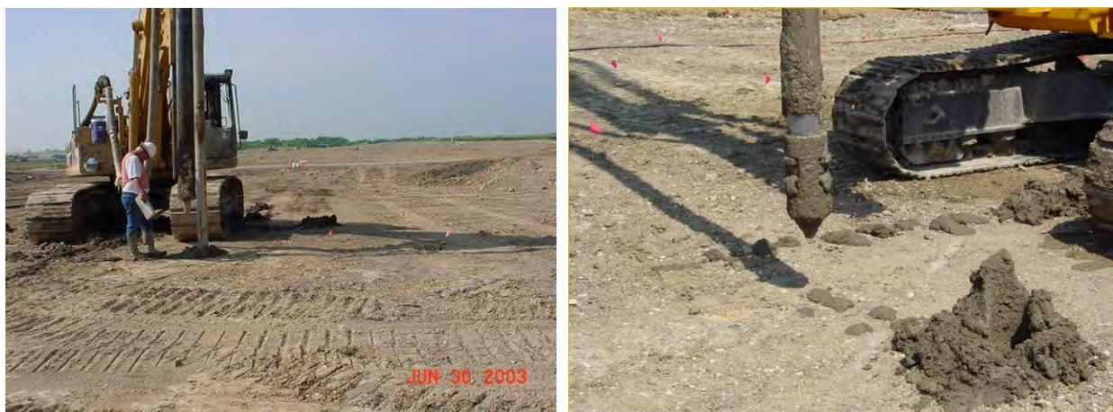
**Figure 20 – Compaction Grouting**
