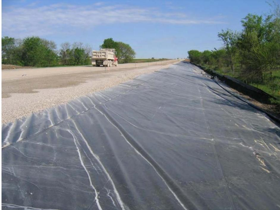
**Figure 16 - The aggregate base layer is completed. Twelve inches of top soil and slab sodding will be placed on the shoulders**
