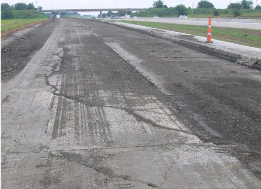
**Figure 10 - Removal of the old pavement; note the thickness of the overlay and the condition of the old concrete pavement**
