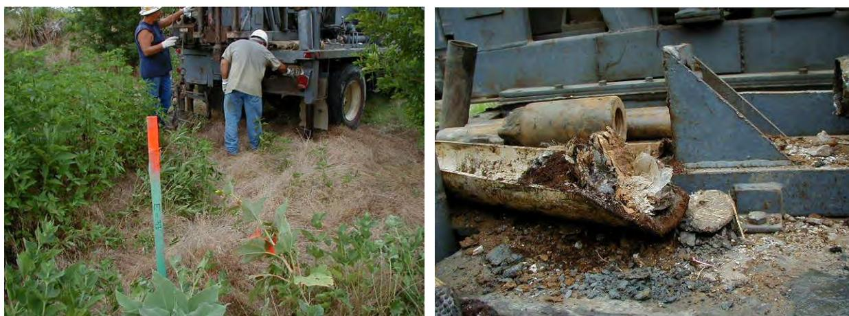
**Figure 6 – Typical Field Exploration and Solid Waste Encountered**
