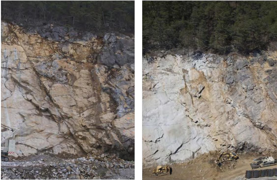
**Figure 8 – Evil Twin Area After Removal of Sliding Rock, But Before Scaling and Bolting. Note release surface formed by discontinuity set 4m dipping steeply to the east (right).**
