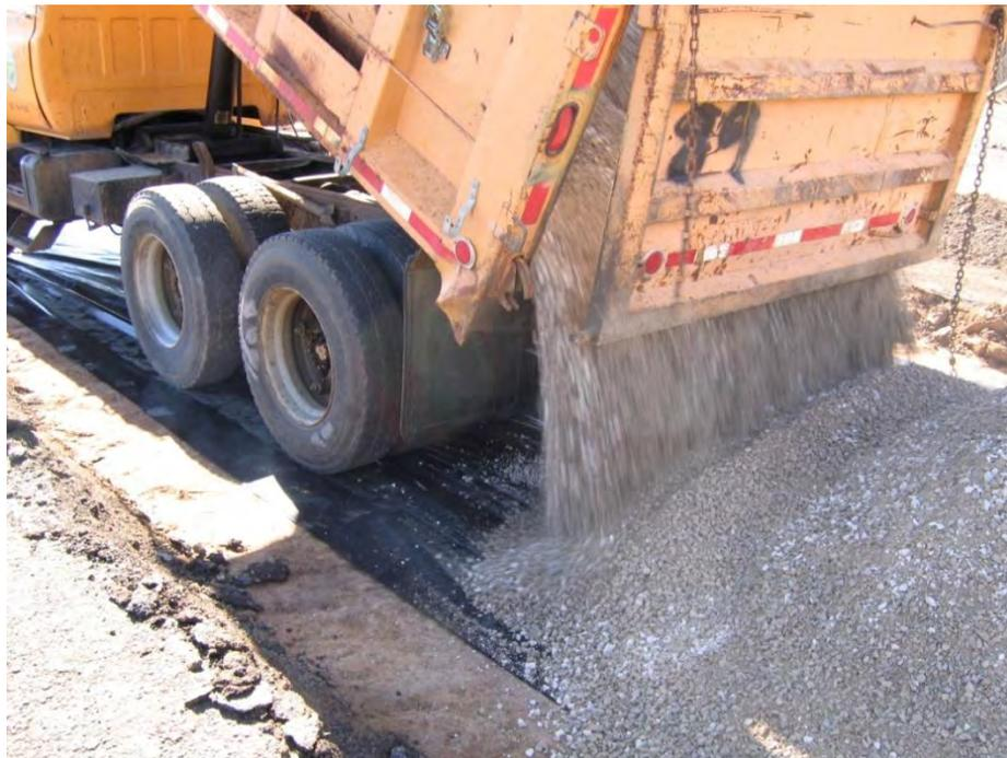
**Figure 4 – Field Test of Proposed Moisture Barrier, dumping the crushed aggregate onto the membrane**
