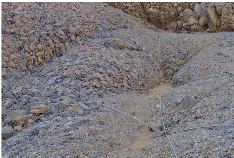
Fig. 2 - Large pockets of debris pushing on the facing and deforming the mesh.
