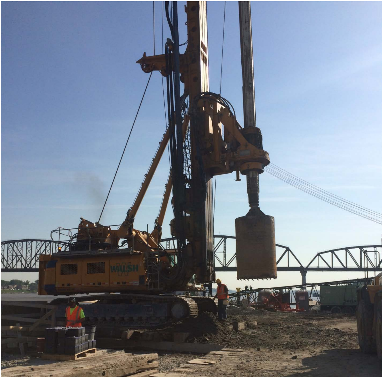
Figure 12. Drilled shaft drill.
