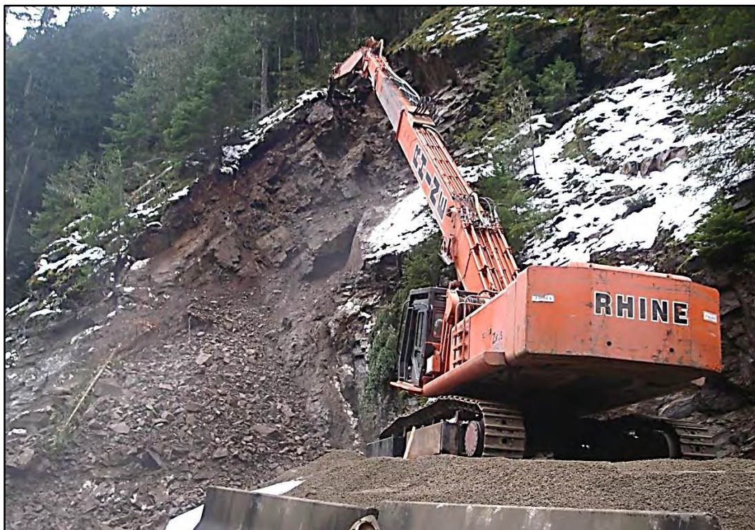
Figure 16: A long-reach excavator removing debris from the slope while on a ramp.
