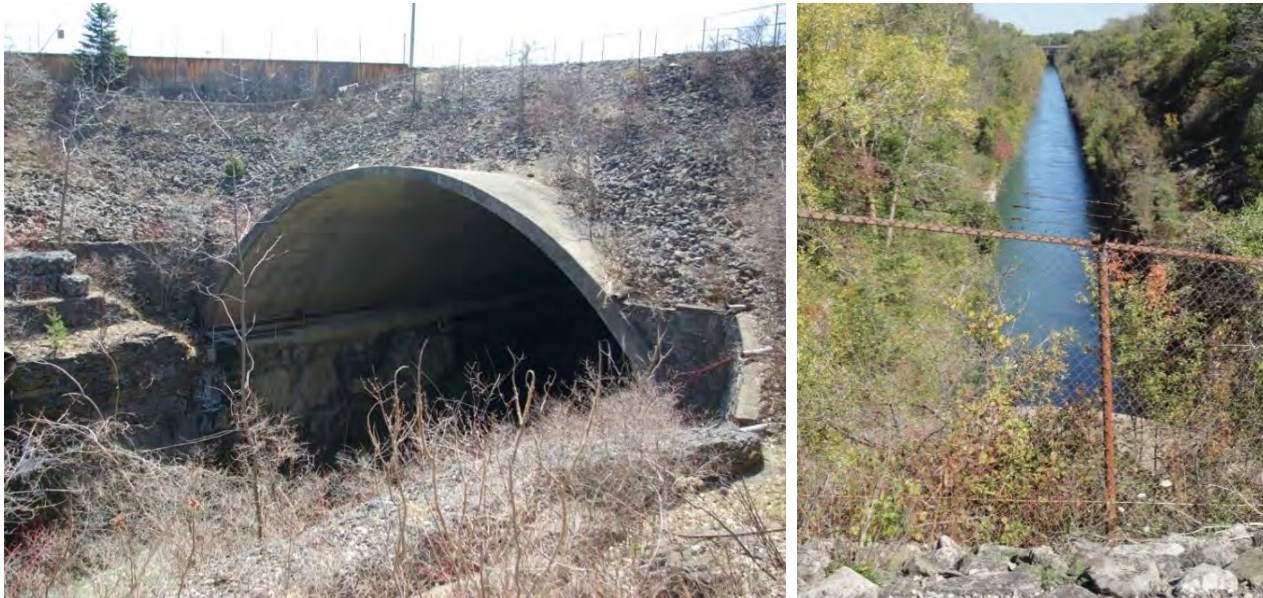
Figure 3: Concrete arch culvert (left) spanning over the Chippawa Power Canal (right)
