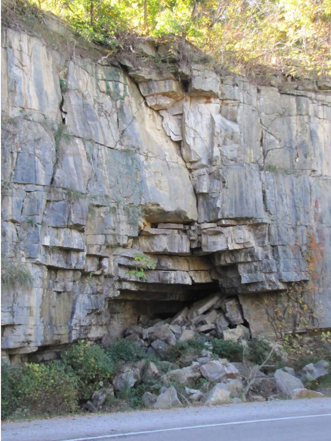
Figure 9. Cavity Located in base of rock cut undermining rock above along vertical joint face
