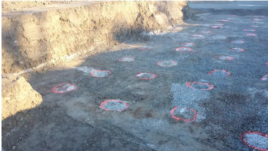
Figure 9 - Garage Footing Subgrade with Exposed CMCs™
