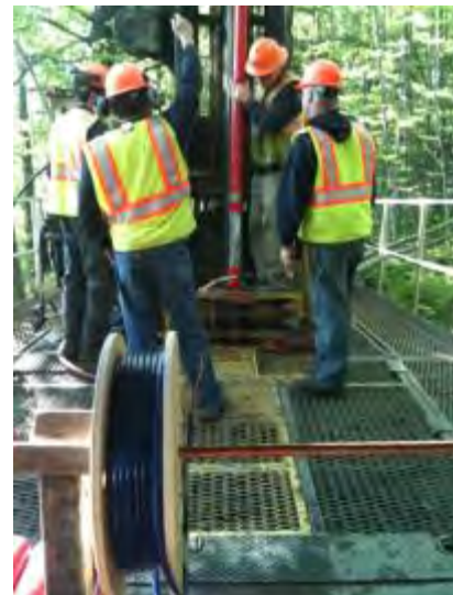
Figure 13 - Installation of inclinometer casing with sonic rig (June 2013).
