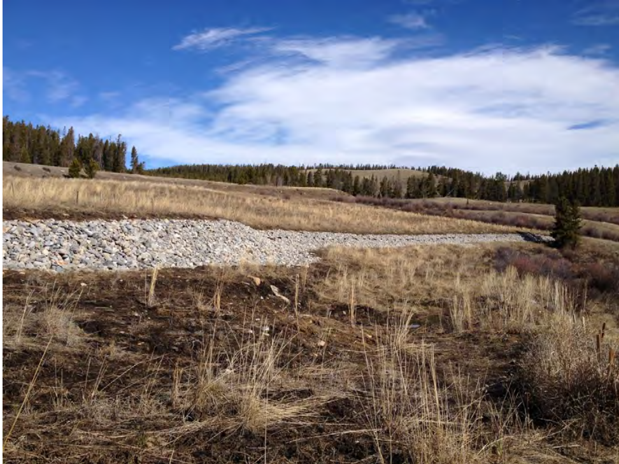
Figure 19 - Completed drainage gallery at Caribou Landslide, Powder River Pass. Drain pipes are exposed at face of rock buttress for future maintenance.
