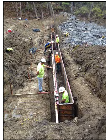
Figure 17 – Concrete cut-off sill under construction
