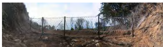
Figure 5 – Channel debris flow barrier with intermediate posts (California - USA)
