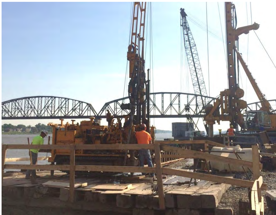
Figure 11. Concrete coring around perimeter of drilled shaft.
