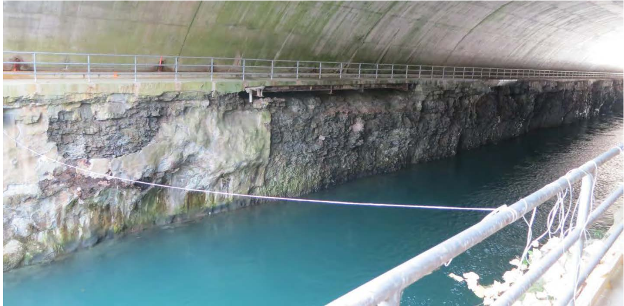
Figure 5: Deterioration of shotcrete lining and rock faces along canal walls
