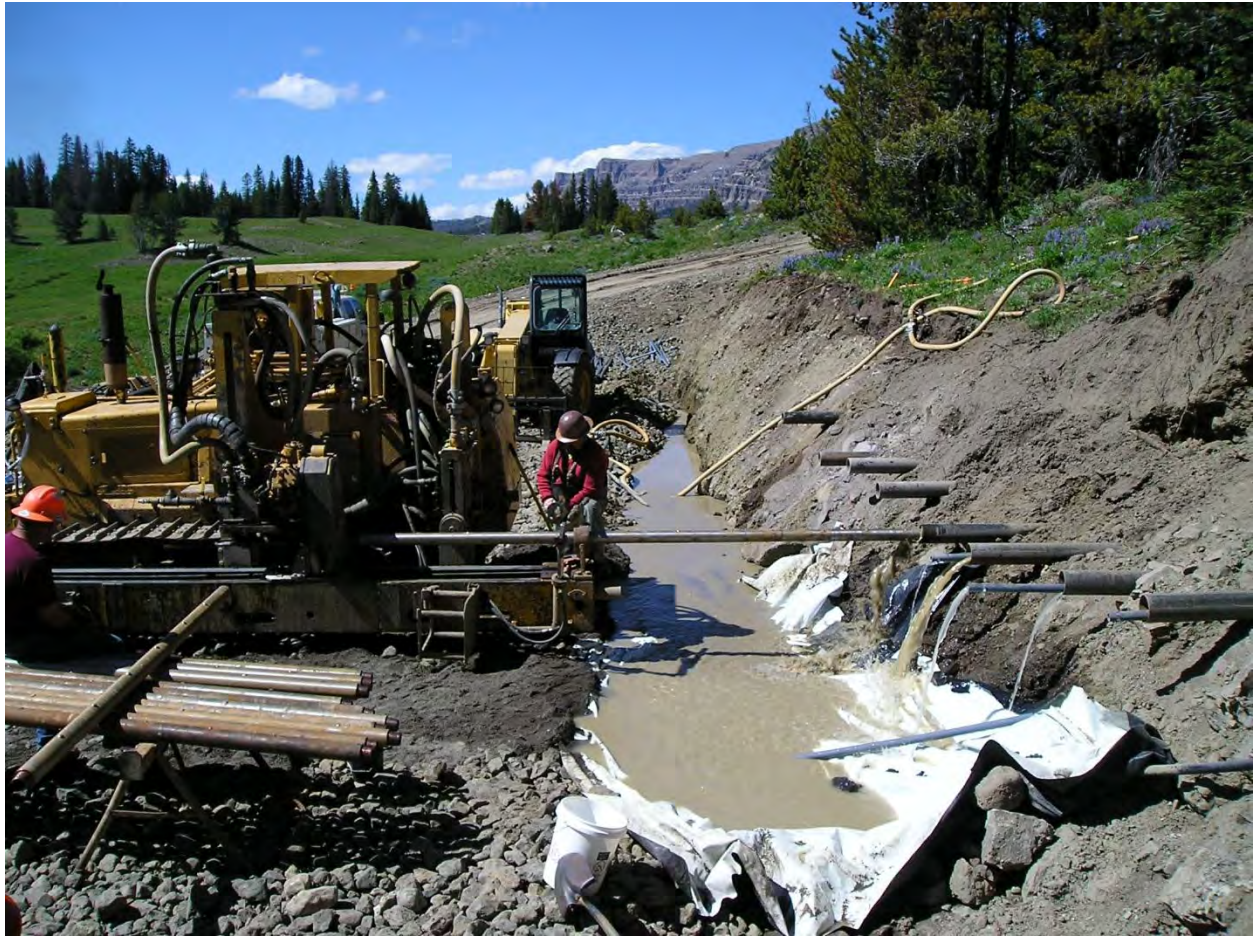
Figure 1 - Construction of horizontal drain pad on Continental Divide Landslide, Togwotee Pass, June 2010.
