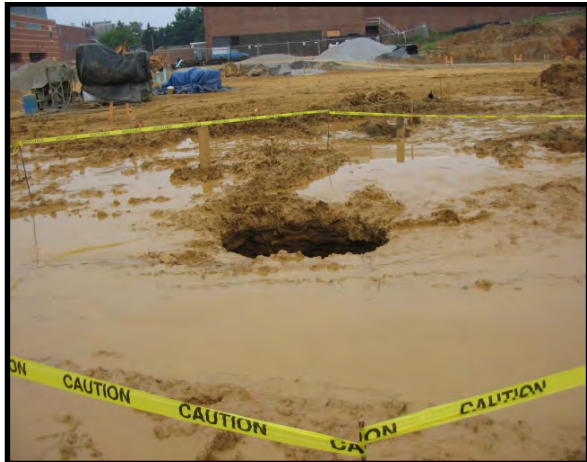
Photos 3 and 4: Sinkholes Encountered During Construction of Campus Building
