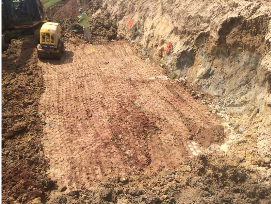
Figure 5. On-site soil placement in compacted lifts.
