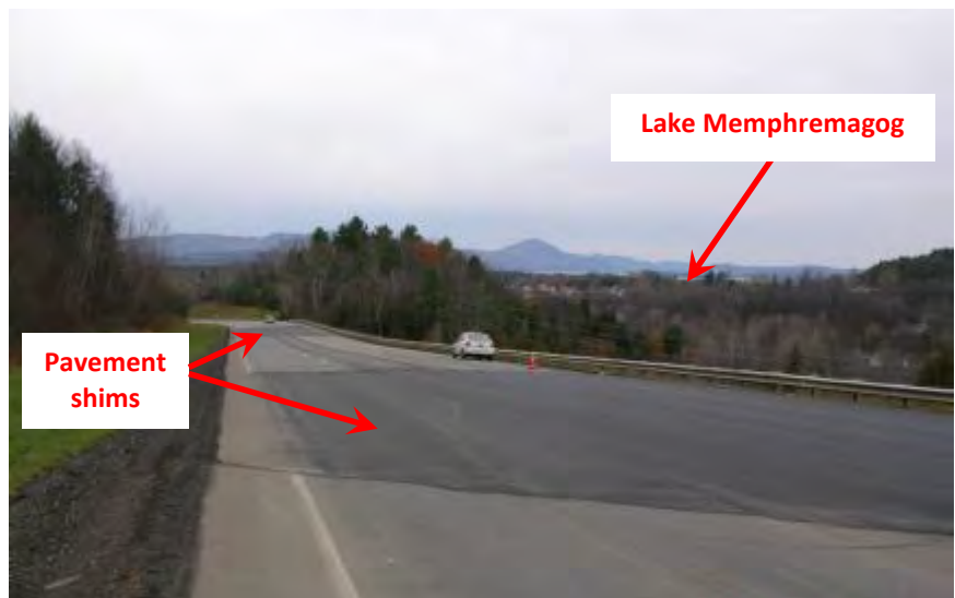
Figure 5 - View to northwest showing pavement shims at headscarp crossing of roadway. Note depression in roadway and stressed guardrail (October 31, 2006).
