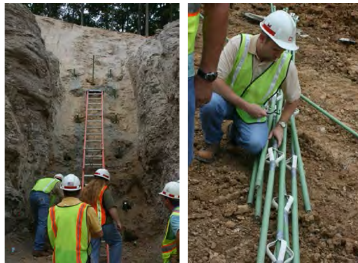
Figure 18. View of Vertical Clay Seams and Soil Nail Installation, September 2008
