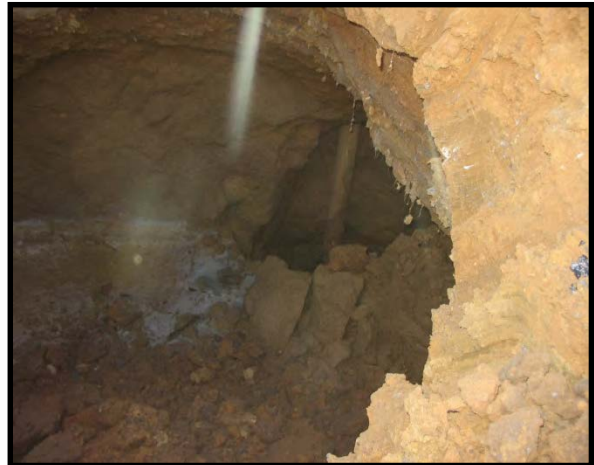
Photos 3 and 4: Sinkholes Encountered During Construction of Campus Building
