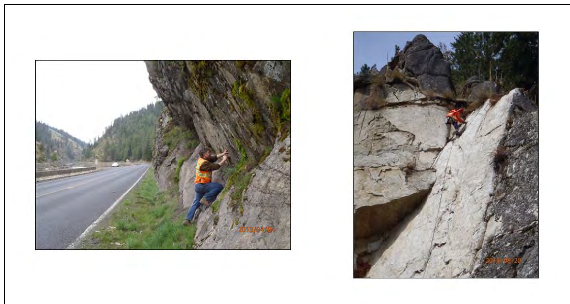
Figure 6: Rockfall catchment zones typically are inadequate (less 90% catchment) to arrest the rockfall. Note blind corners.
