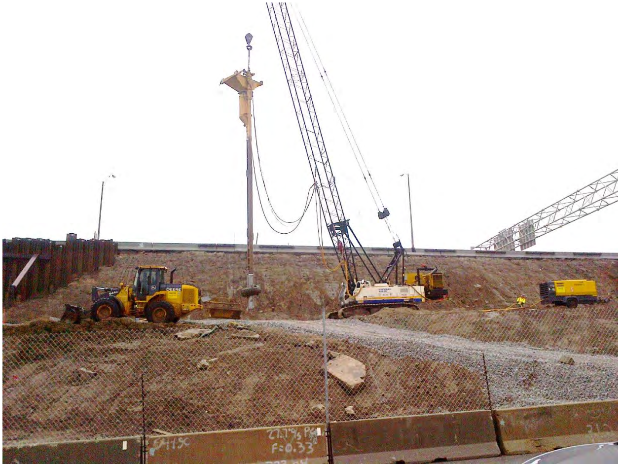
Figure 5. Stone column installation.
