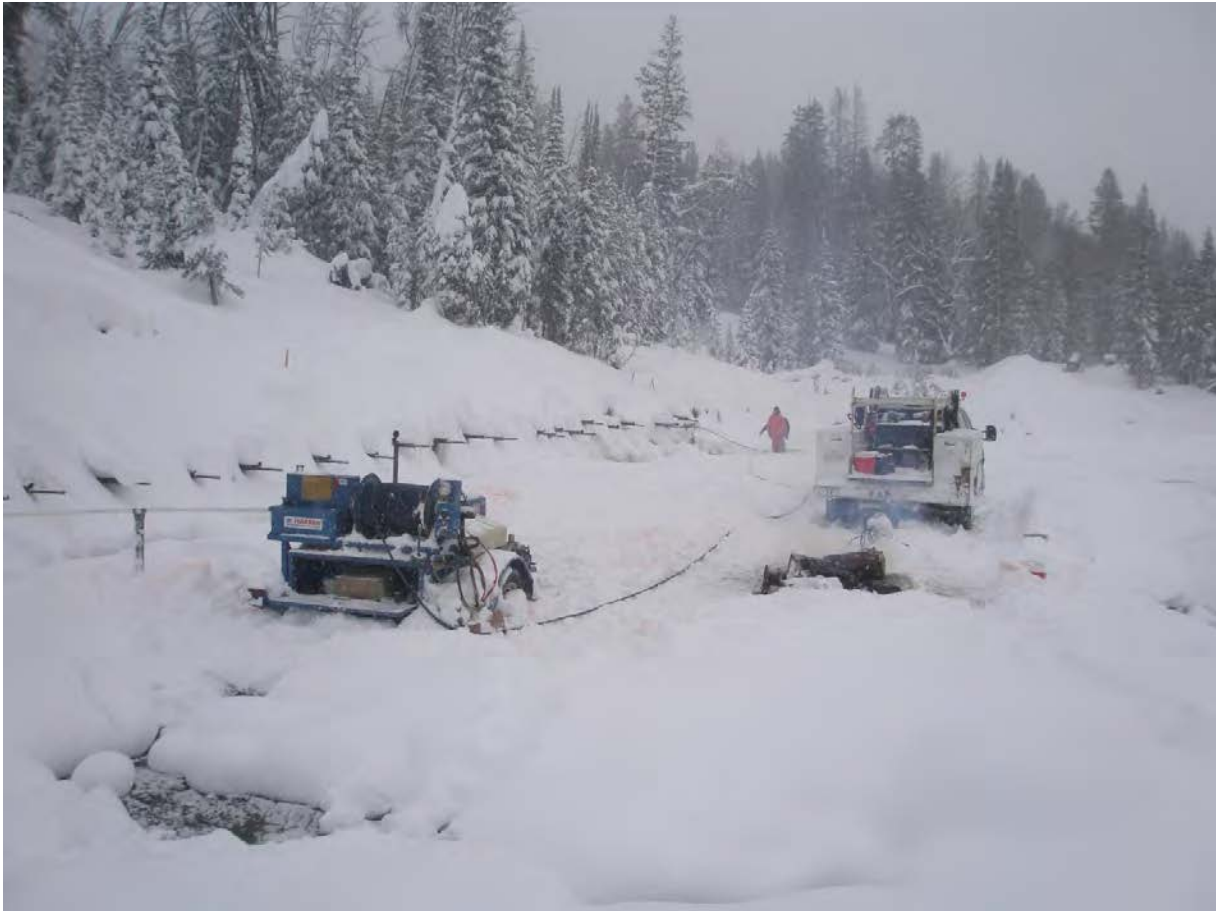
Figure 12 - Jetting of HD's on County Line Landslide, Togwotee Pass, November 2010.
