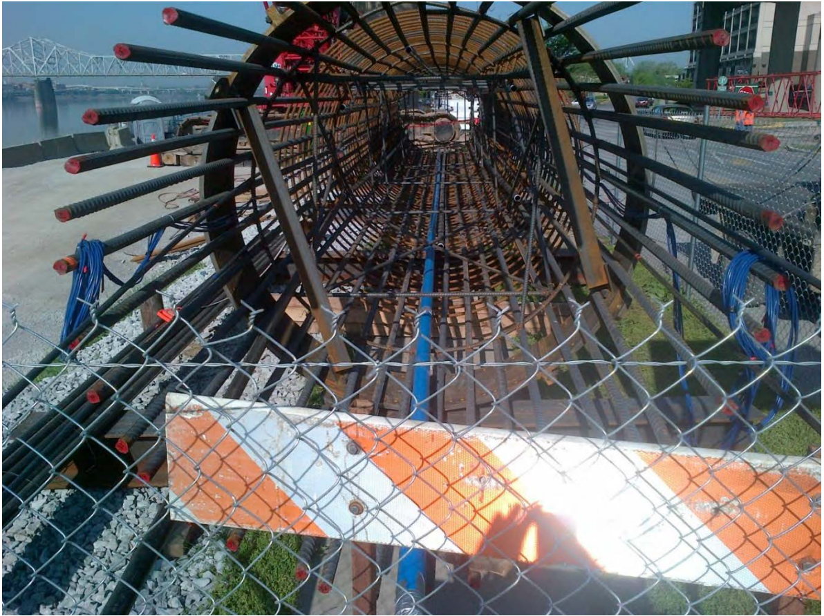
Figure 6. Rebar cage and initial O-cell installation.
