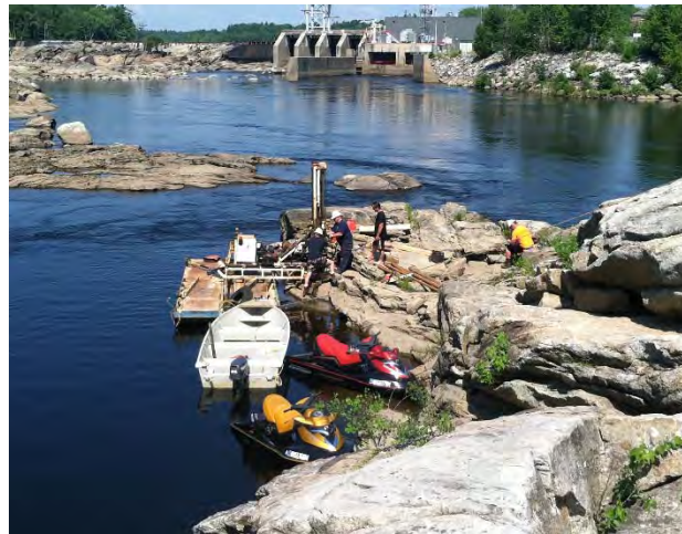
Figure 6 – Test Boring at Bedrock Pinnacle
