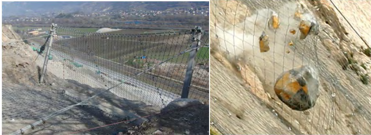
Figure 4: Catchment area of attenuating structure (left) and guided boulder along rock face (right) from Glover et al., 2012.
