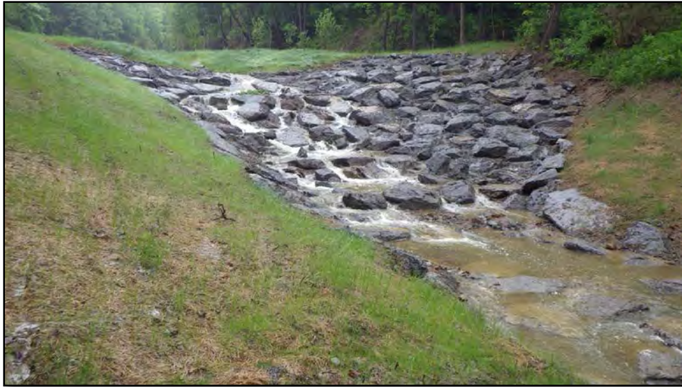
Figure 18 – View of the grouted riprap drop structure
