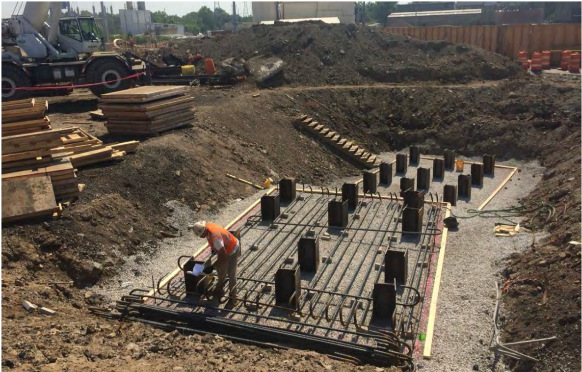
Figure 4. Typical H-pile foundation.
