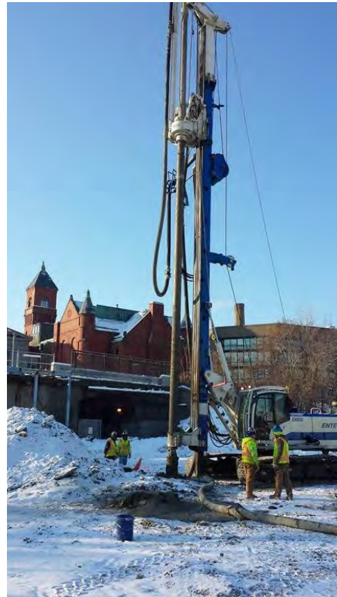
Figure 8 – CMC™ Installation
