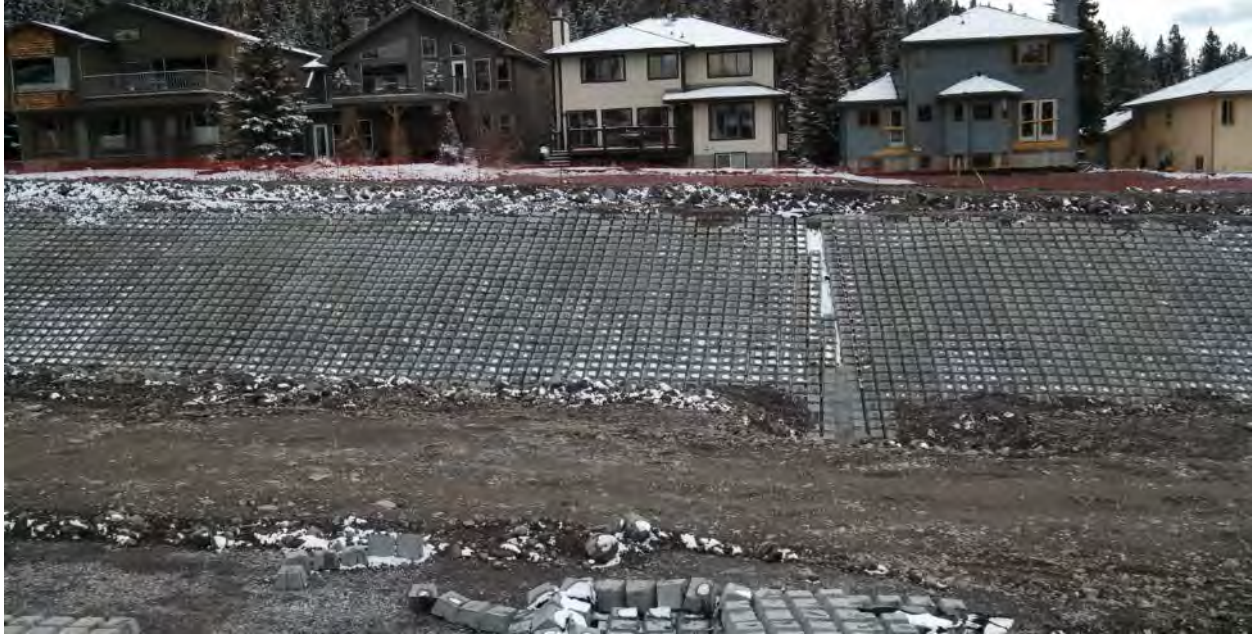
Figure 4 - Excavated channel with articulated concrete mats to prevent mobilization of sediment along the active channel of the Cougar Creek alluvial fan. Photographed during construction. BGC Engineering.
