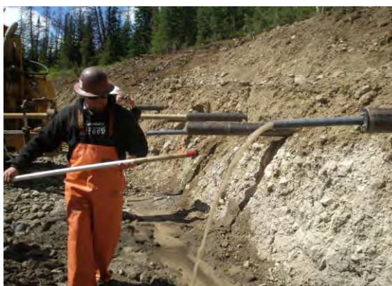
Figure 11 - Pajari assembled in protective casing for preparation to survey HD.
