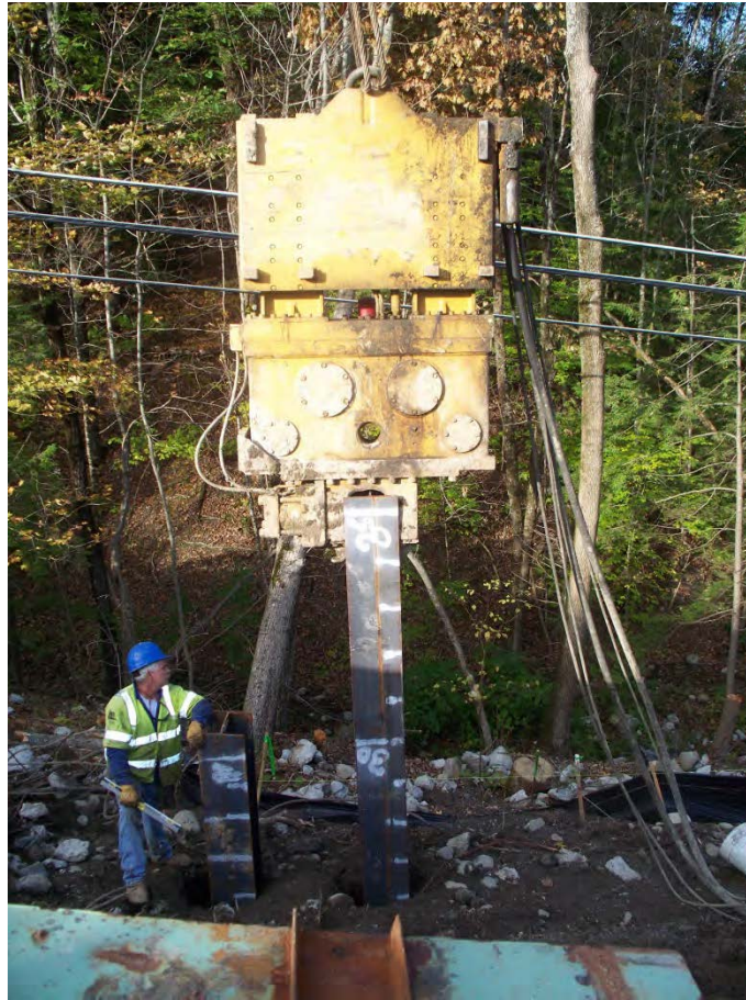
Figure 8 – Installation of HP12x53 stabilization pile by CPM Constructors using an H&M 1700 vibratory hammer supported by a Link Belt LS-318 Crawler Crane. (courtesy of Bryan Steinert)
