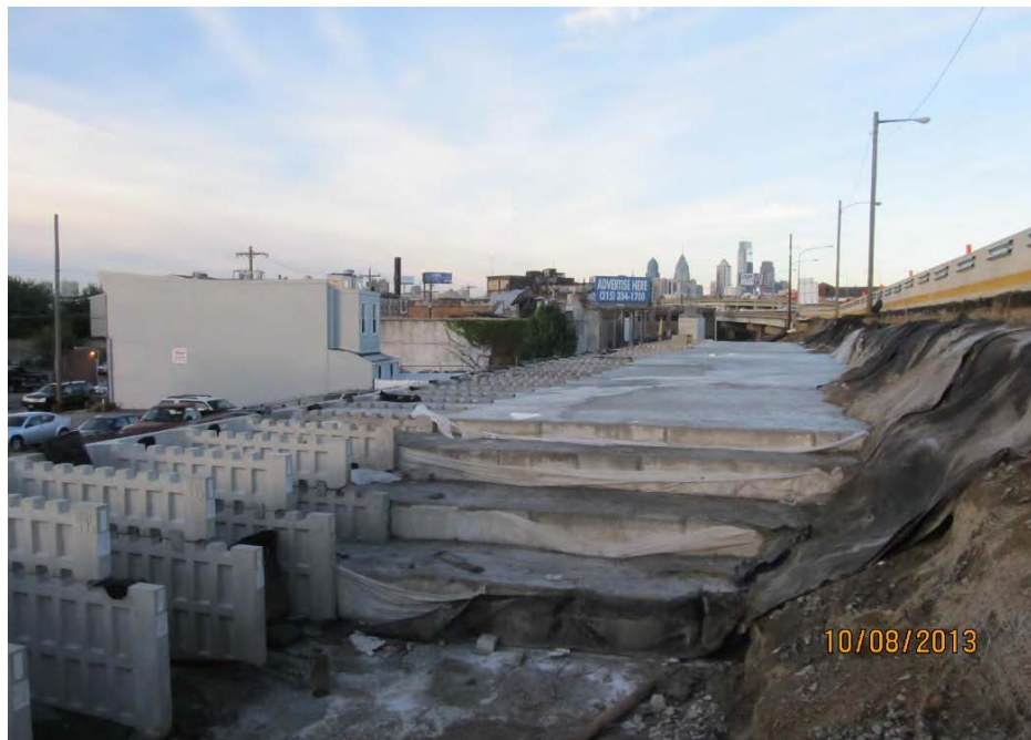
Figure 6: Lightweight Cellular Concrete Sloped at Transition Zone
