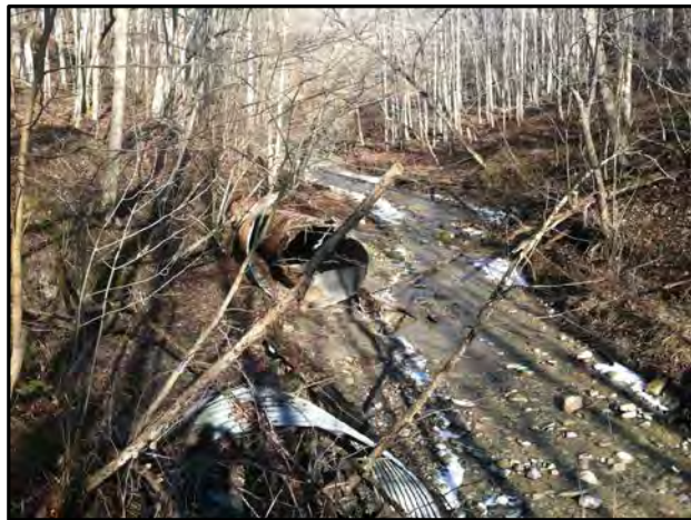
Figure 5 – Dislodged End & Pipe Sections
