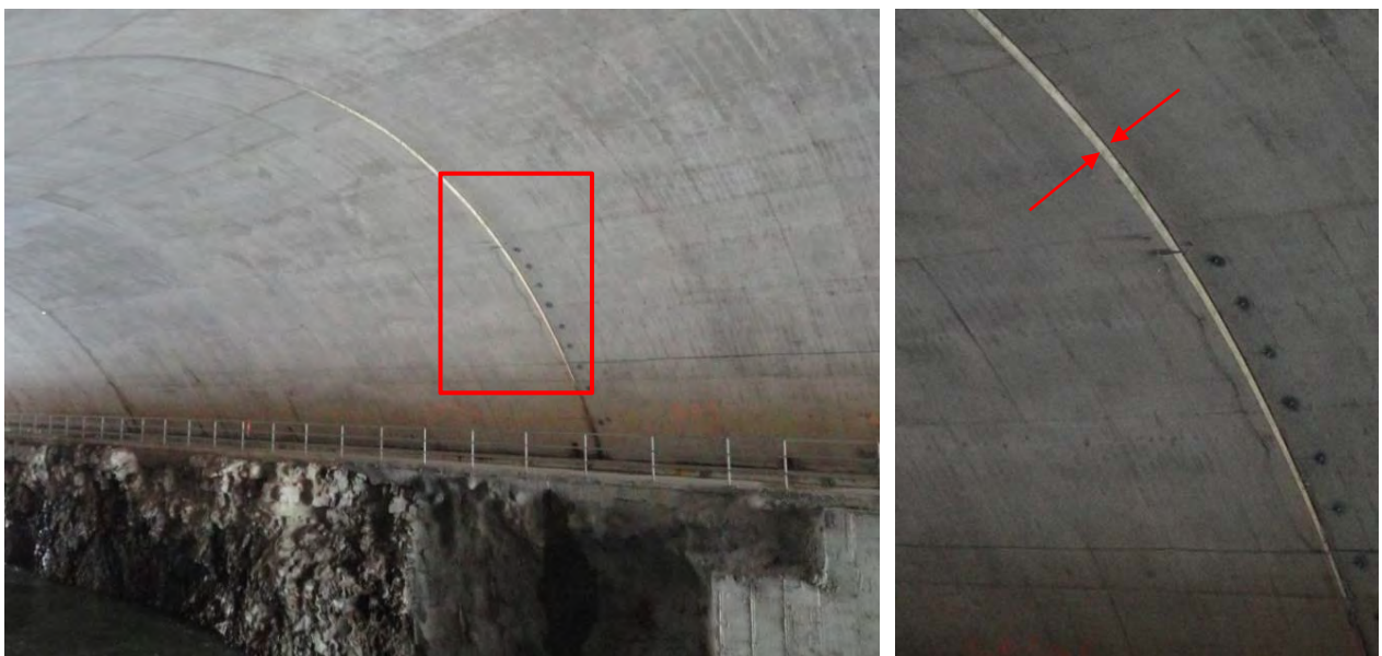
Figure 4: Displacements of culvert segments (right: detail of displacements)
