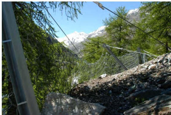
Figure 6 – Impacted open slope debris flow barrier (Italy)
