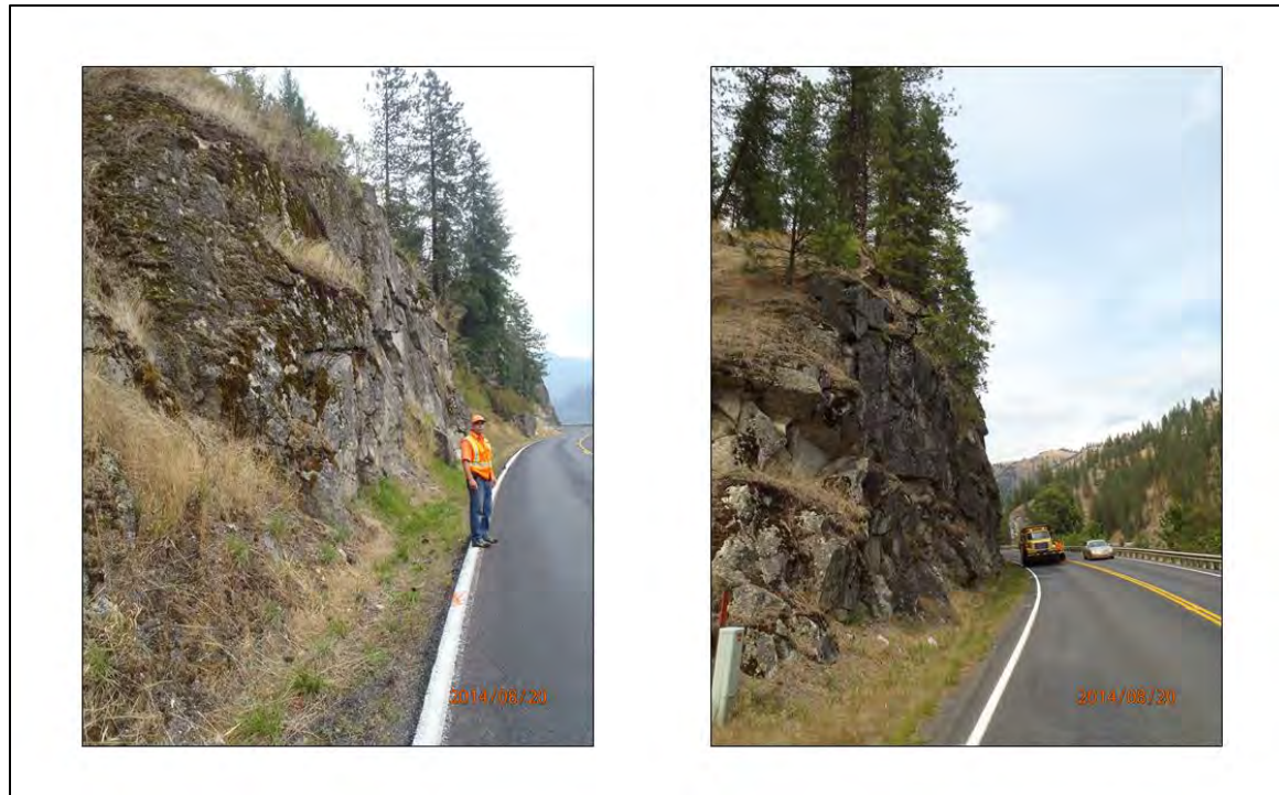
Figure 6: Rockfall catchment zones typically are inadequate (less 90% catchment) to arrest the rockfall. Note blind corners.
