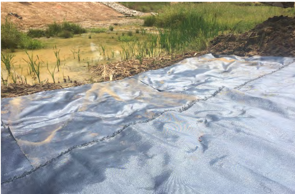
Figure 4. Horizontal installation of high strength wicking geotextile.
