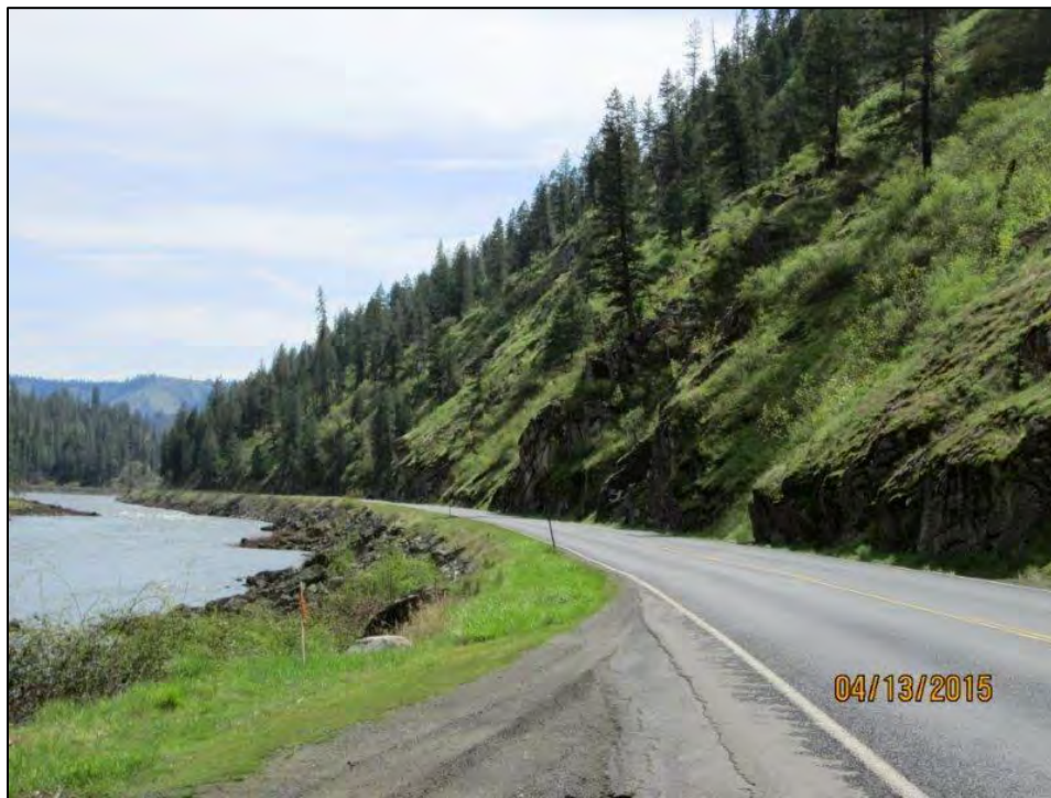
Figure 8: Most of the cut slopes have been stable with some raveling and minor rockfall since the slopes were constructed in 1935.
