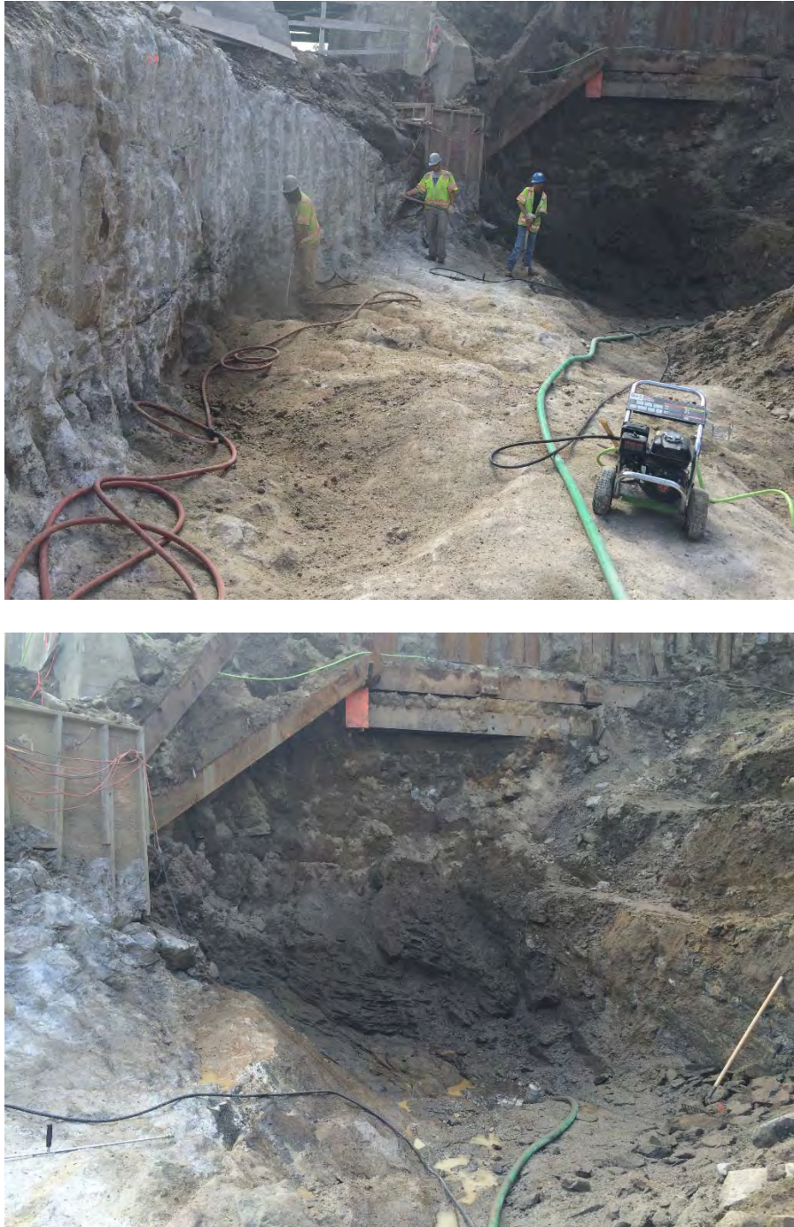
Figure 19 – Line Drilling to Excavate Granite Intrusion (top) and Contact Zone between Granite and Altered Schist (bottom)
