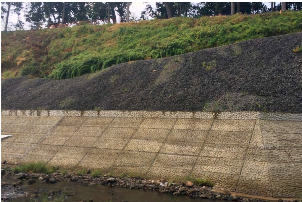
Figure 3 – Phase 1 Concrete Buttress at South Embankment
