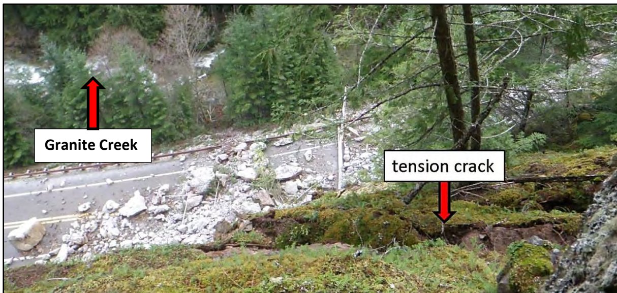
Figure 5: Looking down from the top-of-cut at a large tension crack, debris, and Granite Creek.
