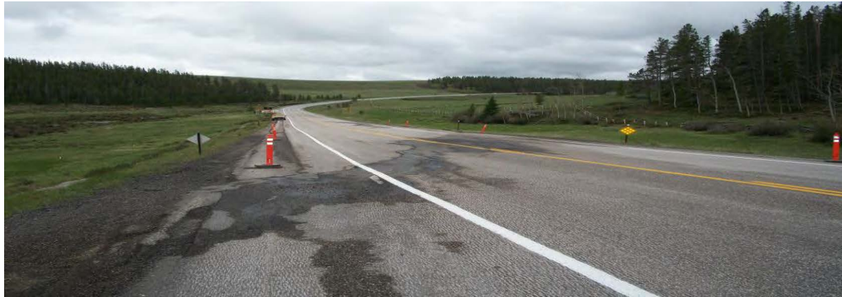
Figure 3 - Damage to US 16 on Powder River Pass by the Caribou Landslide. Excessive moisture due to winter snowpack accelerated slide movement. A horizontal drain pad was constructed near Crazy Woman Creek to the left of the photo.
