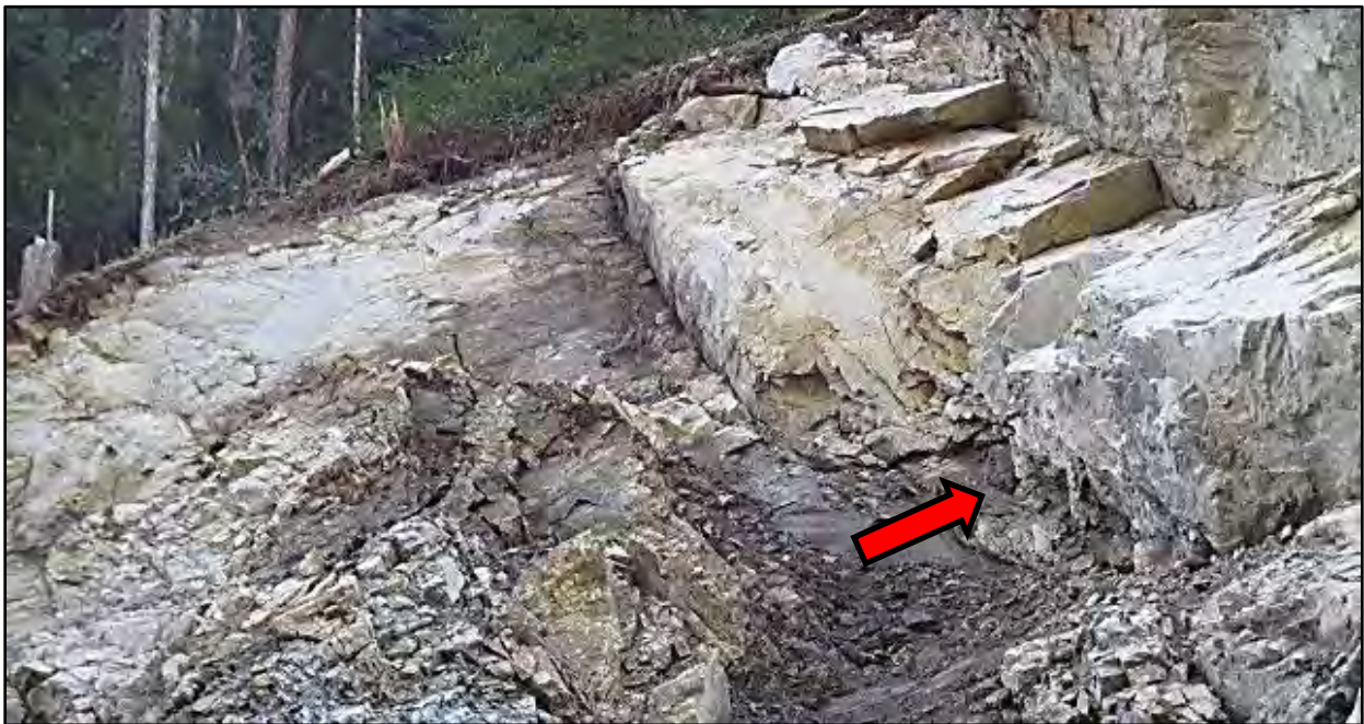
Figure 19: Minor blast damage to the back slope from the surface charges.
