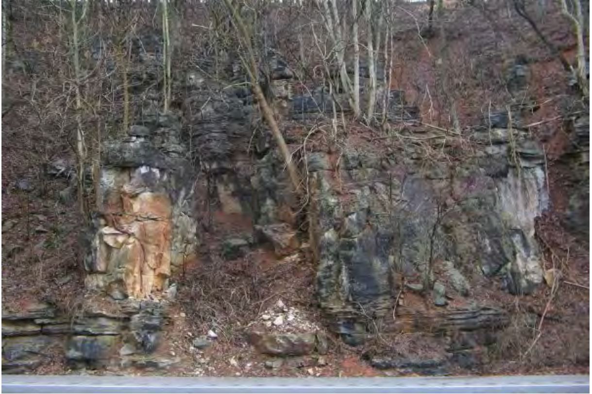
Figure 7. Solutioning in Limestone along Natural Rock Slope Face on I-40 in Putnam County, TN located at margin of Highland Rim and Cumberland Plateau
