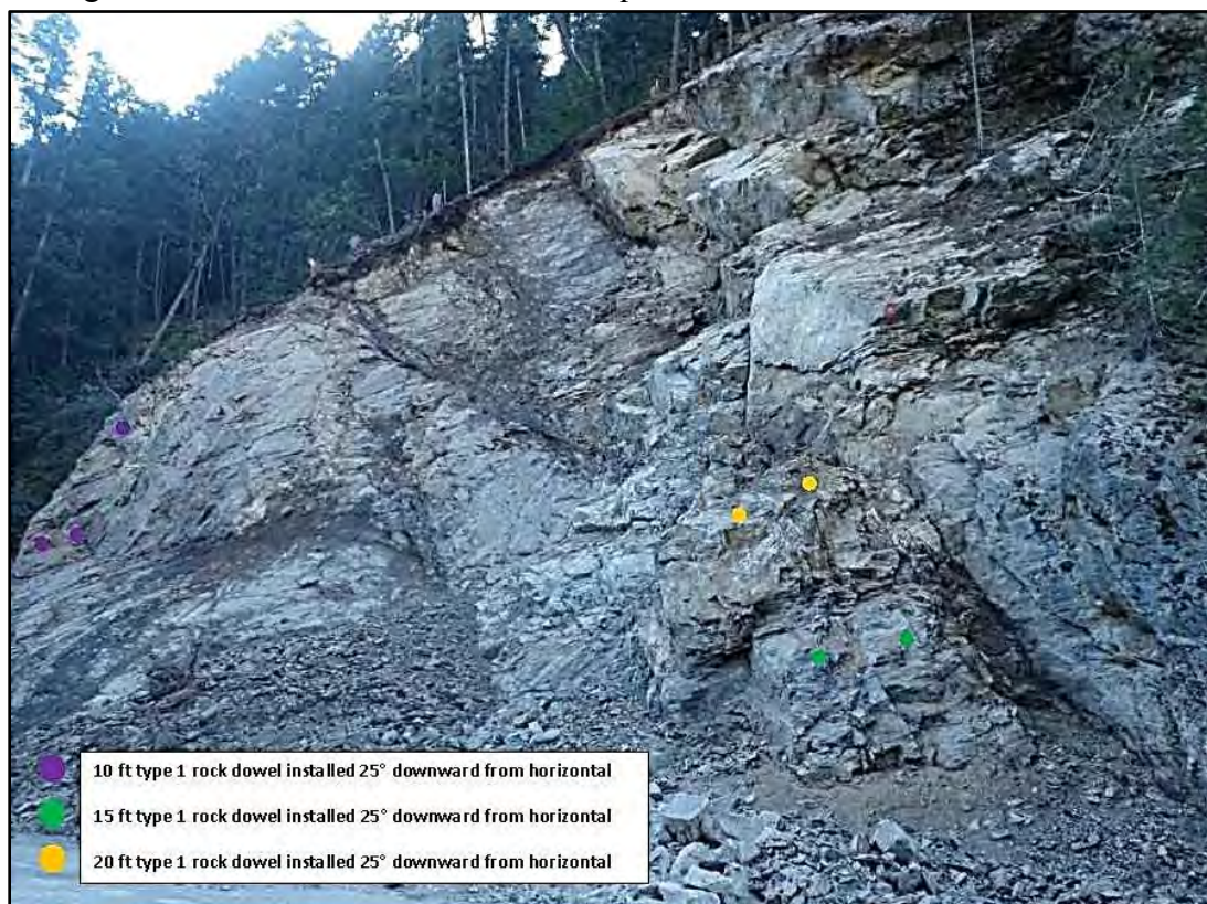
Figure 22: Additional recommended slope reinforcement in the eastern & western sections.
