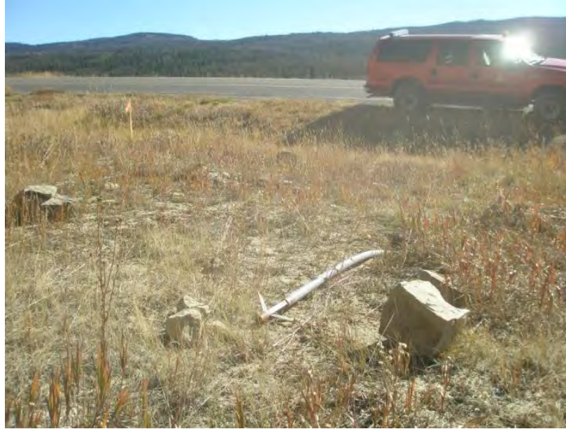
Figure 7 - Care should be taken for correct azimuth and angle of a drain. However, the photo above proves when horizontal drilling, bits tend to have a mind of their own.
