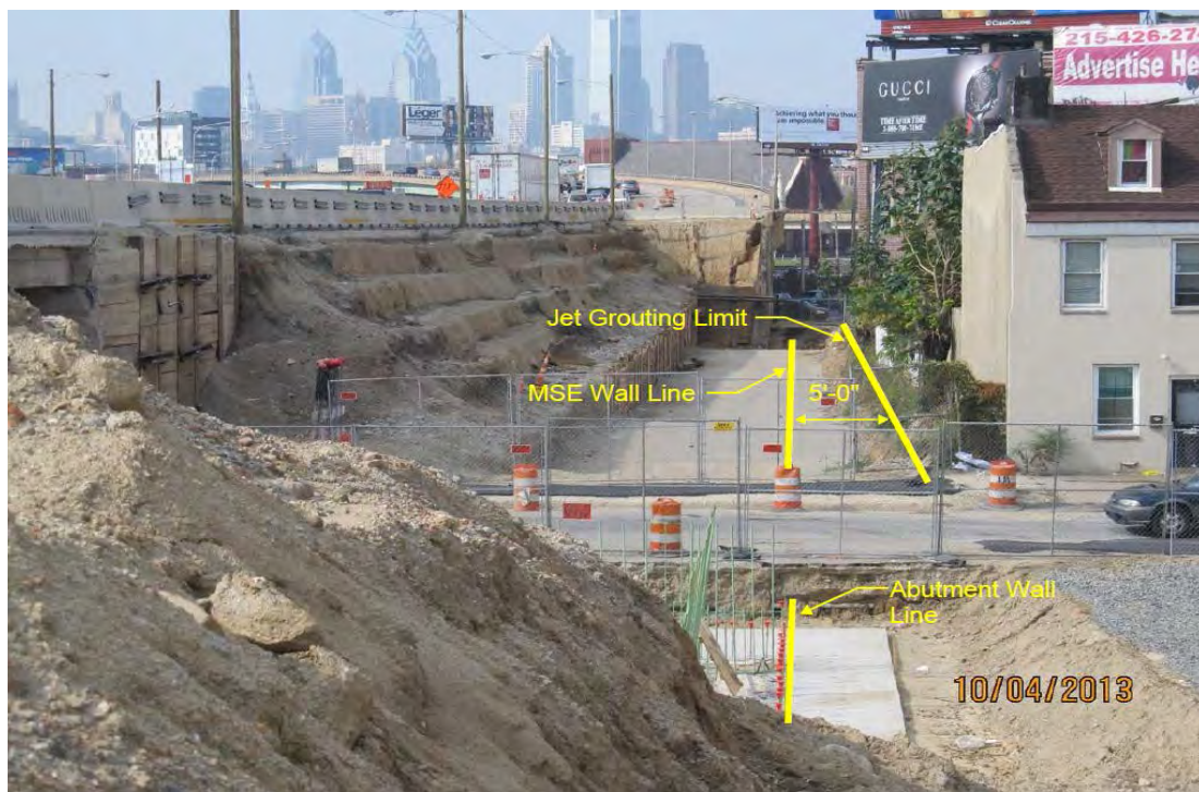
Figure 4: Proximity Proposed Jet Grouting Treatment Limits To Buildings
