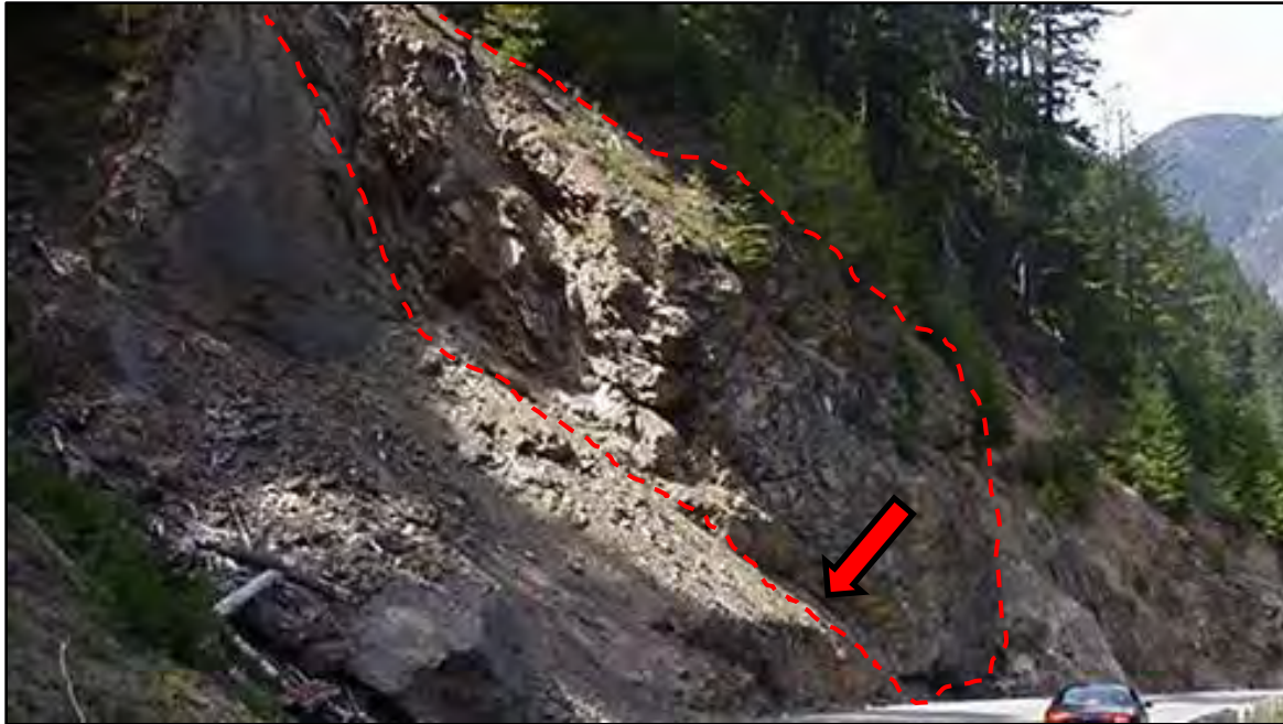
Figure 9: The slope before the failure with a roadway-dipping discontinuity near the toe-of-slope.
