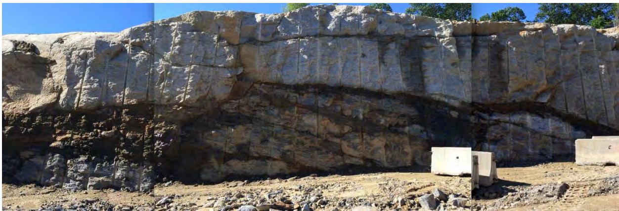
Figure 20 – Granite Intrusion over Altered Schist in Roadway Cut
