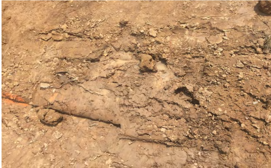
Figure 7. Water observed at face of slope during construction.
