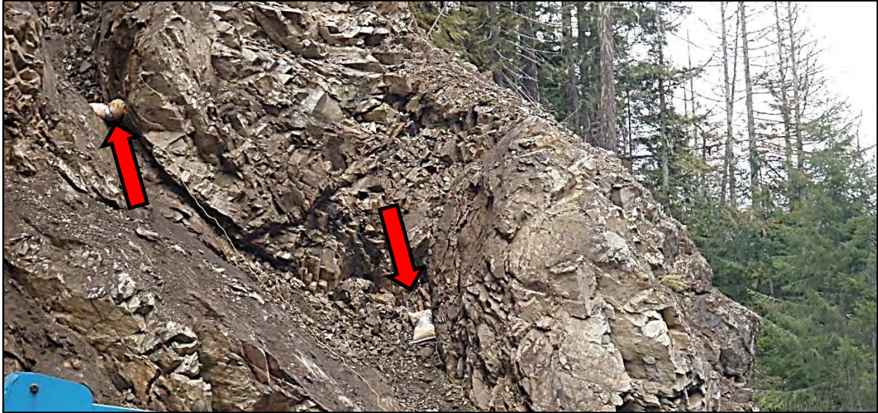
Figure 18: Surface charges placed on the slope.
