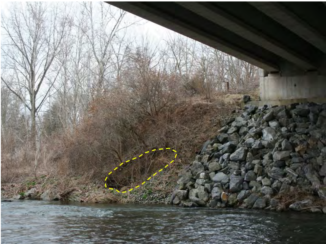
Figure 5 – Recurring sinkhole adjacent to SR33 bridging crossing the Bushkill Creek. Taken in April of 2015.
