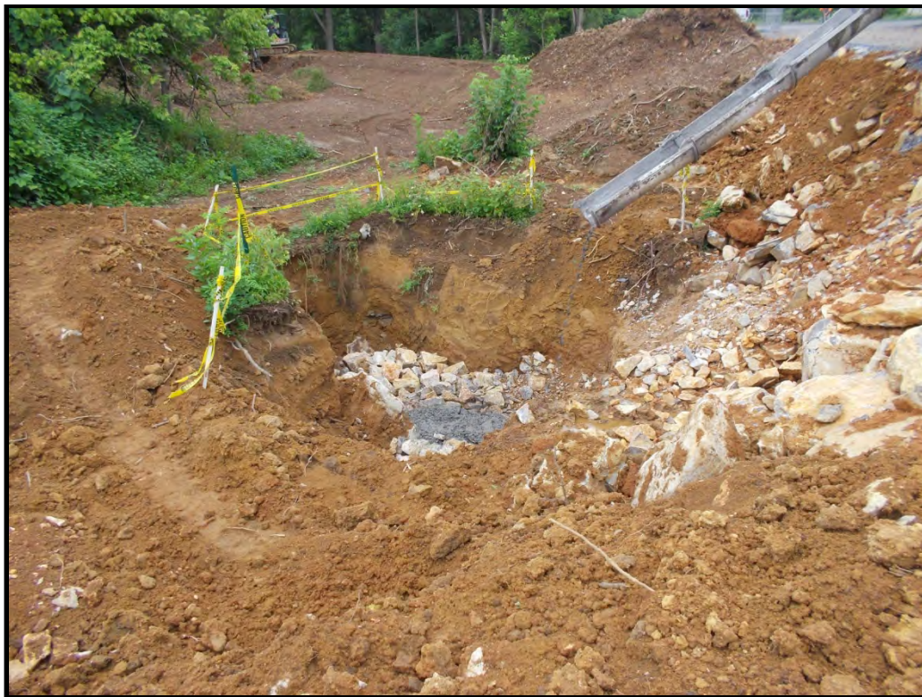
Photo 10: Sinkhole Repair
