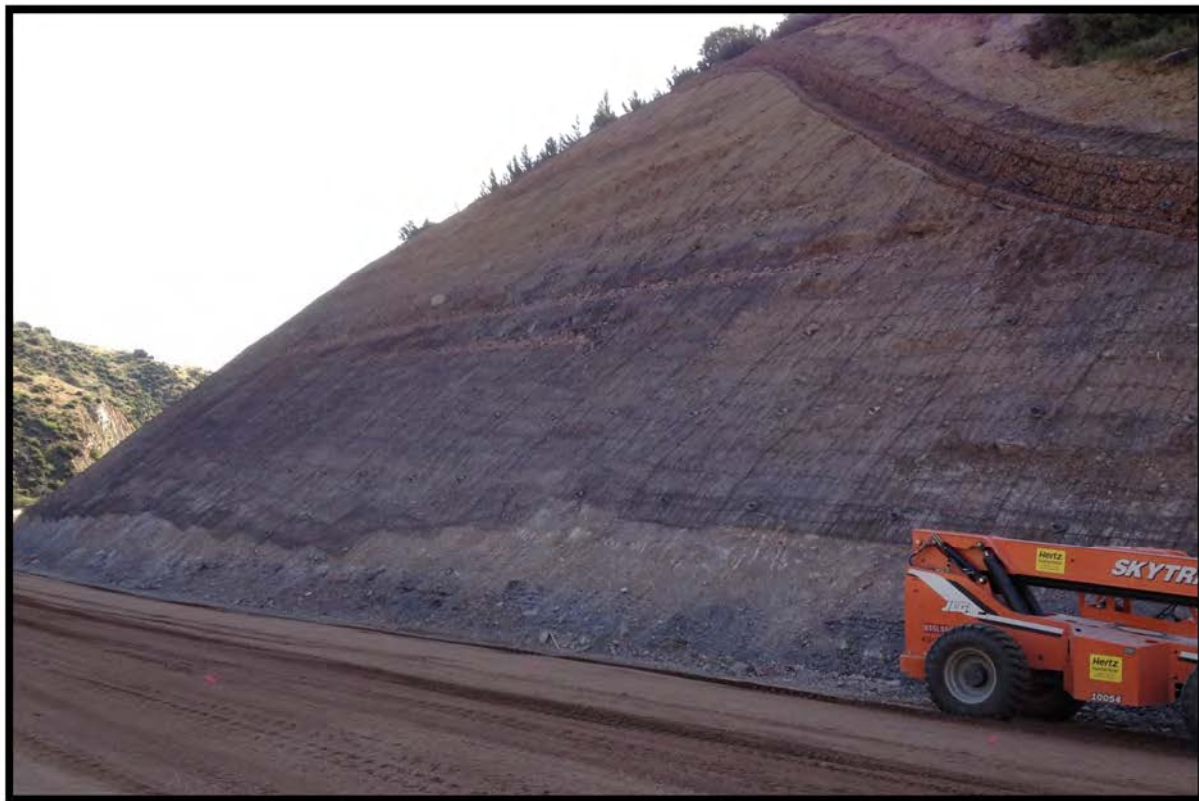
Figure 8 – Photograph of the finished cut slope with the mesh fully installed and the seeding effort half completed.
