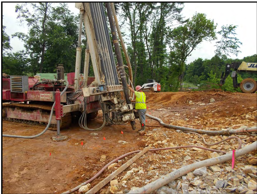
Photo 7: Battered Micropile Installation
