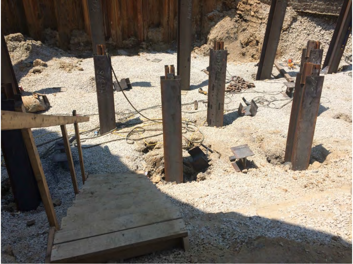
Figure 9. Cavitation after pile driving.
