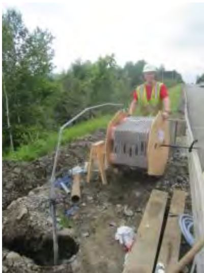
Figure 14 - Installation of SSA inclinometer (June 2013).
