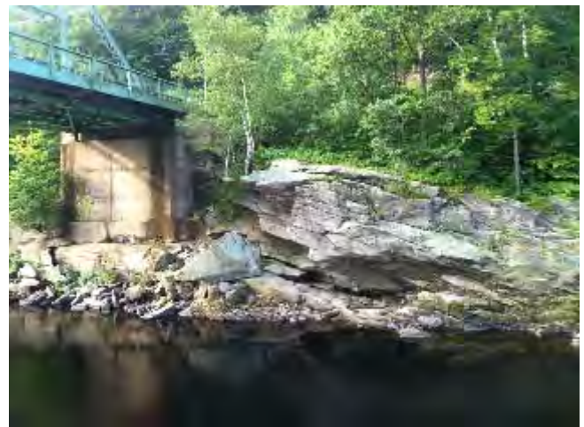
Figure 2 – Undermined Area, Durham Abutment
