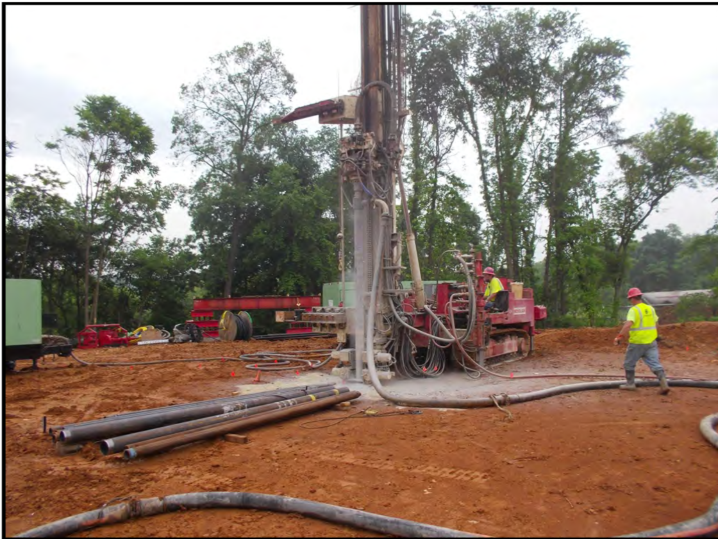
Photo 6: Micropile Installation
