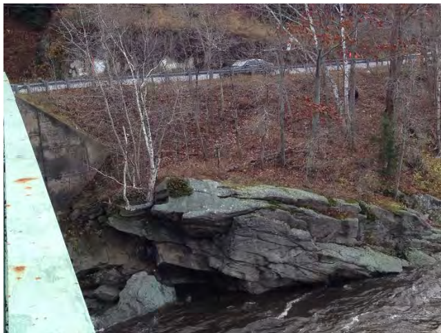
Figure 2 – Undermined Area, Durham Abutment
