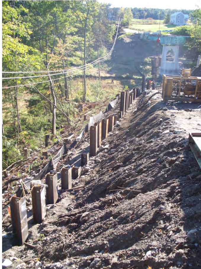
Figure 7 – Installed HP12x53 stabilization piles along the north side of the west approach embankment. (courtesy of Bryan Steinert)
