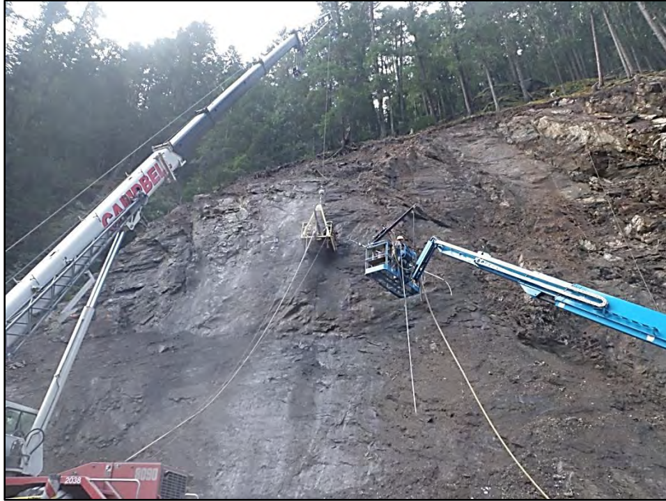
Figure 23: Drilling the dowel locations from a crane and a man-lift.
