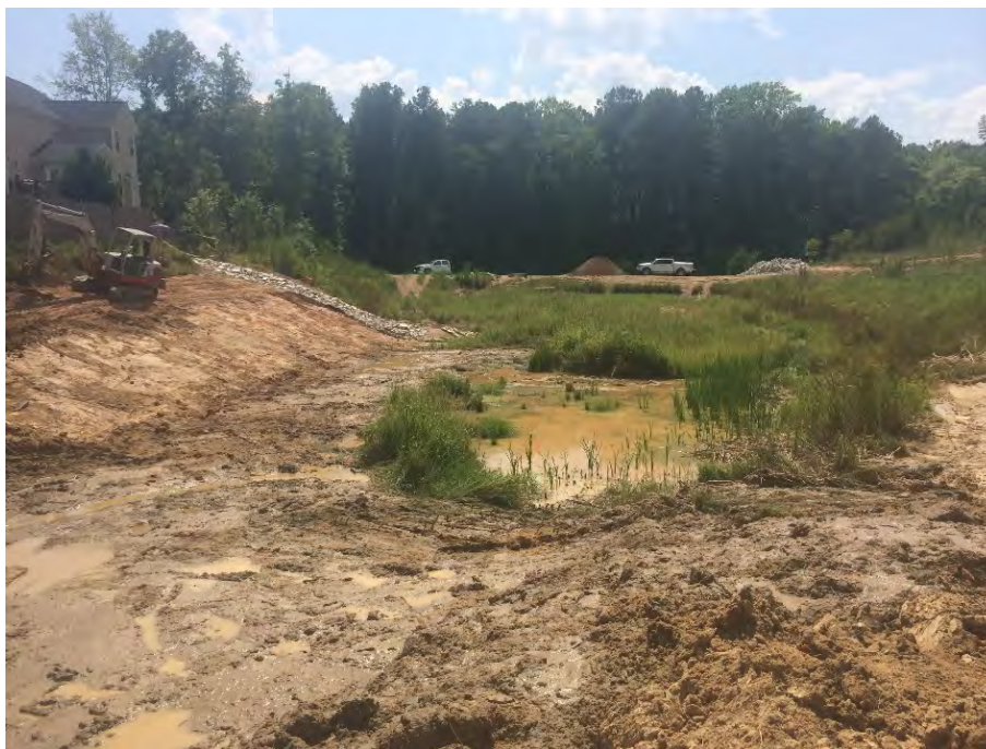
Figure 6. Final grading of the high strength wicking geotextile reinforced slope.
