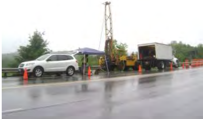
Figure 12 - Drilling conventional geotechnical borings on shoulder of roadway (June 2013).
