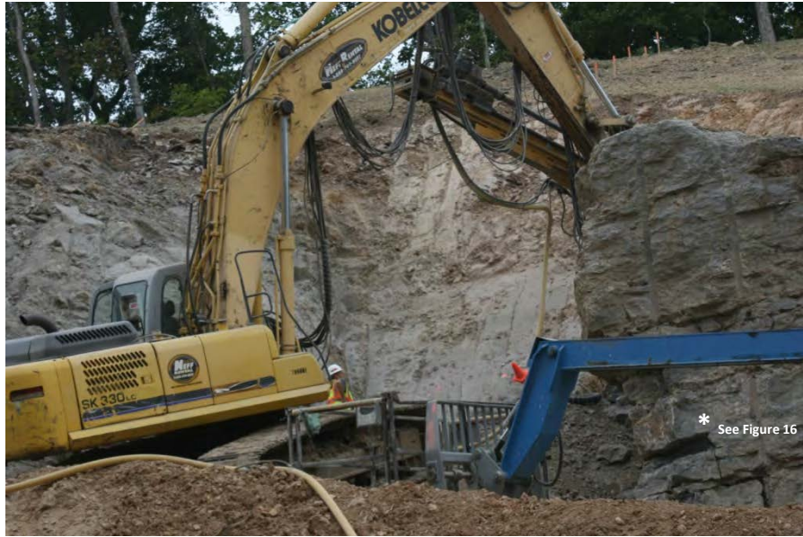
Figure 15. Excavation of mudcutter at the top of the left rim excavation - 2008
