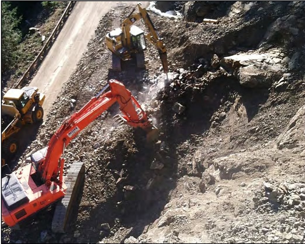
Figure 20: A hoe-ram and an excavator removing material from the lower portion of the slope.
