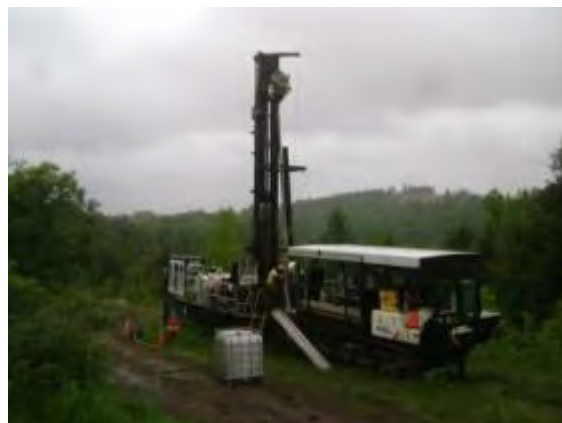
Figure 10 - Drilling test borings on the counter berm using a track-mounted sonic drilling rig (June 2013).
