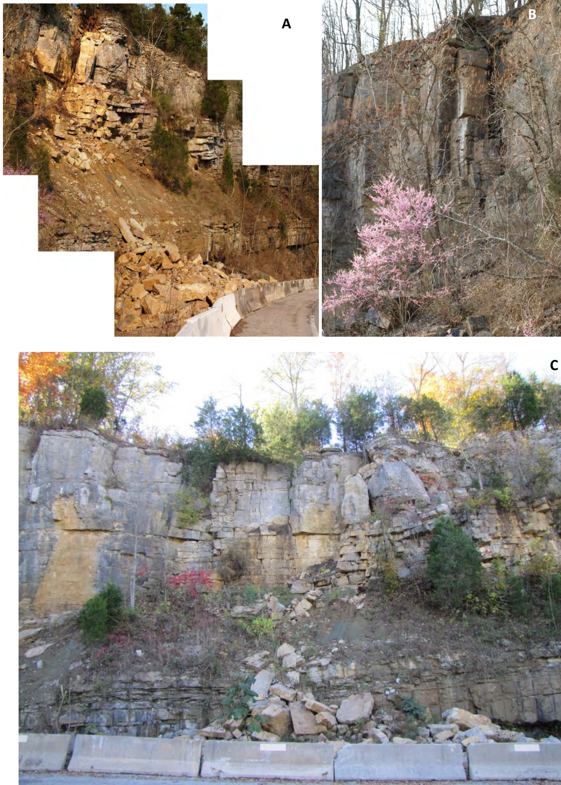
Figure 8. SR-16, Franklin County, TN – Shale layers undermine overlying larger limestone boulders with vertical joints leading to secondary toppling failure of the rock
