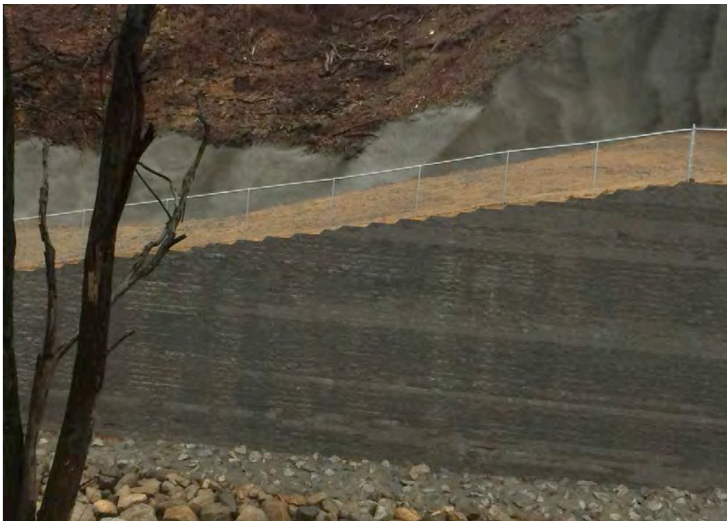
Figure 11 – Completed Project GCS Wall
