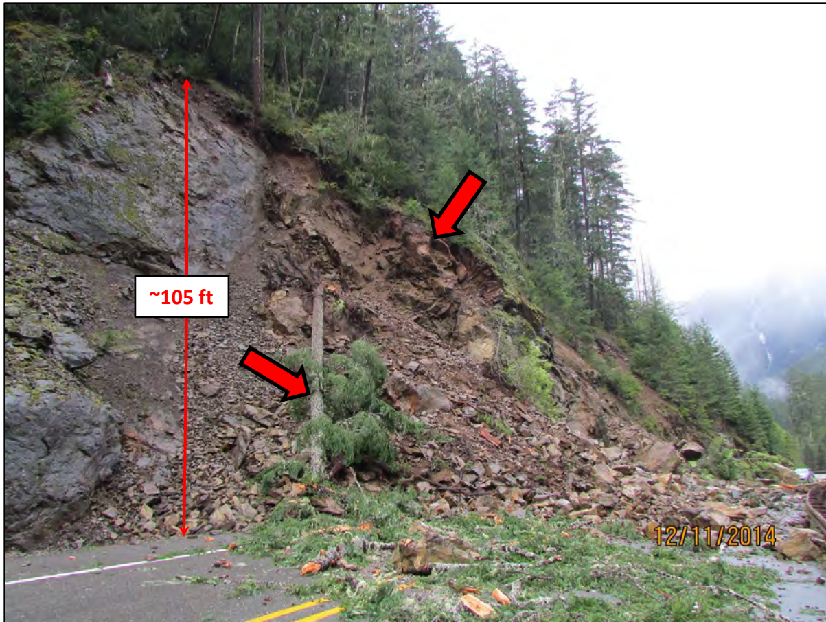
Figure 4: Eastern view of debris on the slope and scattered over both lanes of the highway.
