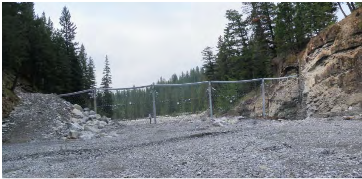
Figure 3 - Flexible debris net located at the head of the Cougar Creek fan is 40 m wide by 6 m tall and is designed to trap coarse sediment, while allowing fine grained sediment and water to pass. BGC Engineering.
