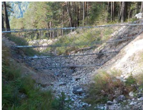
Figure 4 – Channel debris flow barrier with no posts (Italy)
