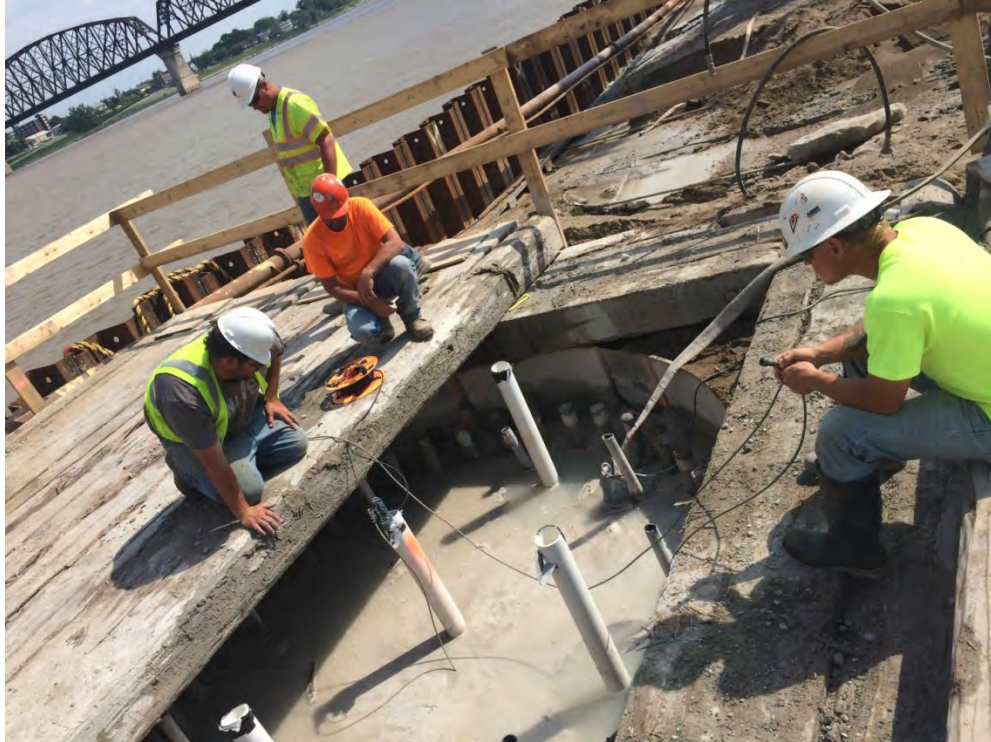
Figure 10. Cross hole sonic logging of drilled shaft.
