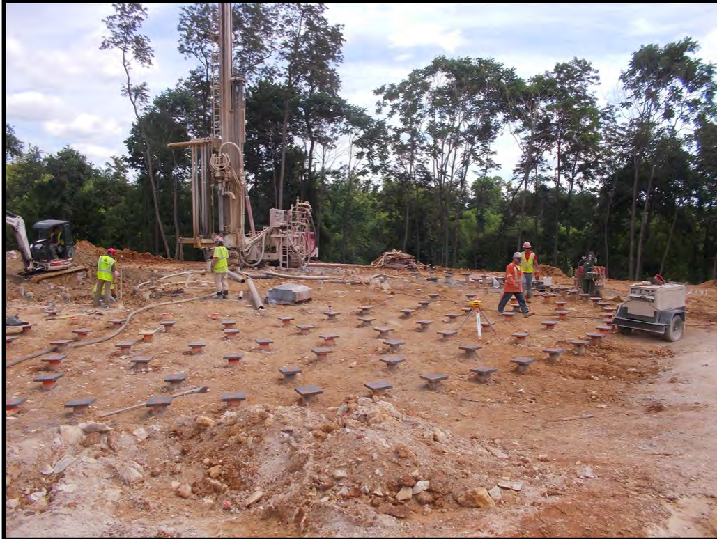
Photo 8: Completed Micropiles
