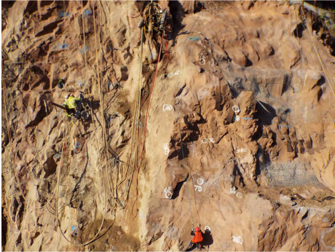
Figure 6 – Image of a portion of the south side of the slope where a flash coat of shotcrete was applied before drilling and installation of the anchors. Flash coating was necessary due to the observed weak rock conditions.
