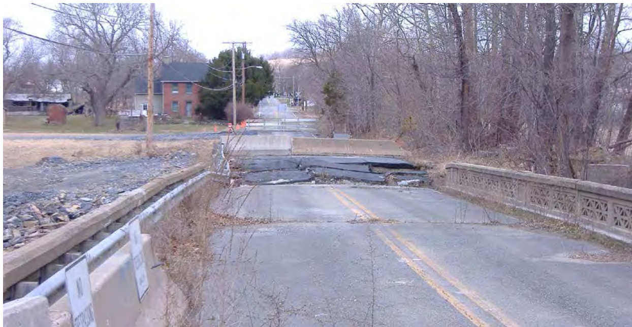
Figure 3 – North Abutment of SR 2017 Bridge over the Bushkill Creek after October 2000 sinkhole.
