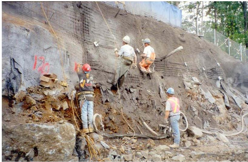
Figure 2 – Soil Nail Wall Being Constructed
