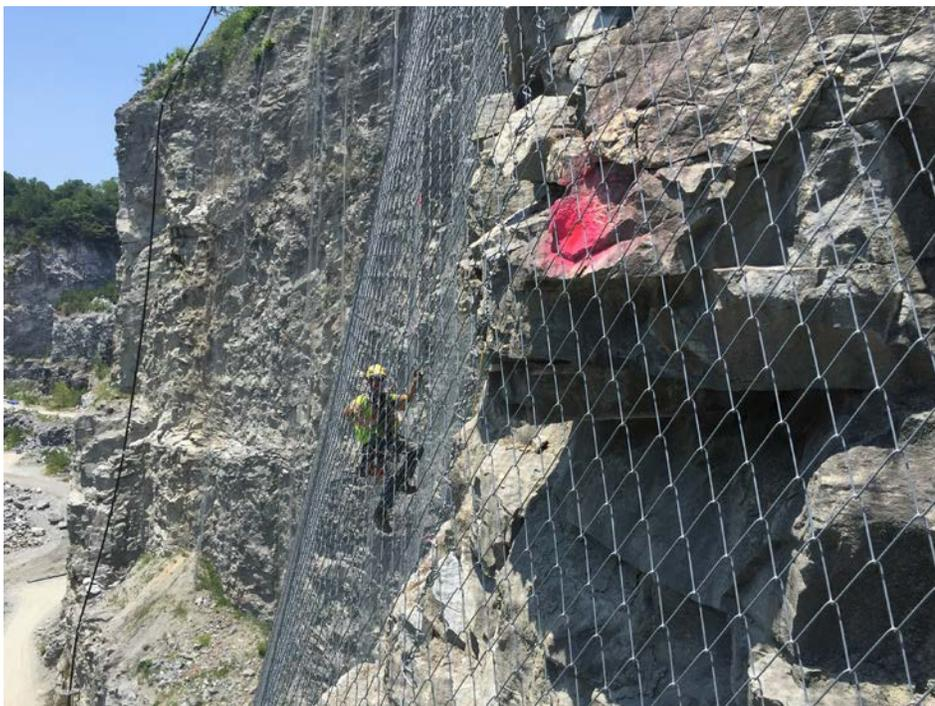
**At left:** Rock dowel layout using rope access techniques on the Bellwood Quarry rock slope, as part of temporary rockfall mitigation efforts for tunneling associated with the City of Atlanta, Water Supply Program – Phase 1. *Photo courtesy Dave Scarpatto, Scarptec, Inc.*
