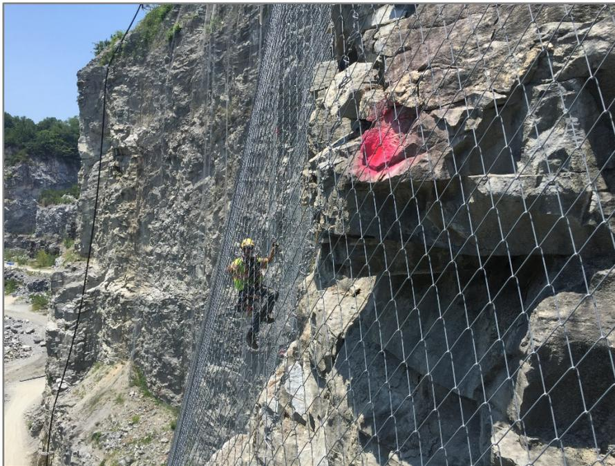
**Figure 3 – Rock dowel layout with paint using rope access
