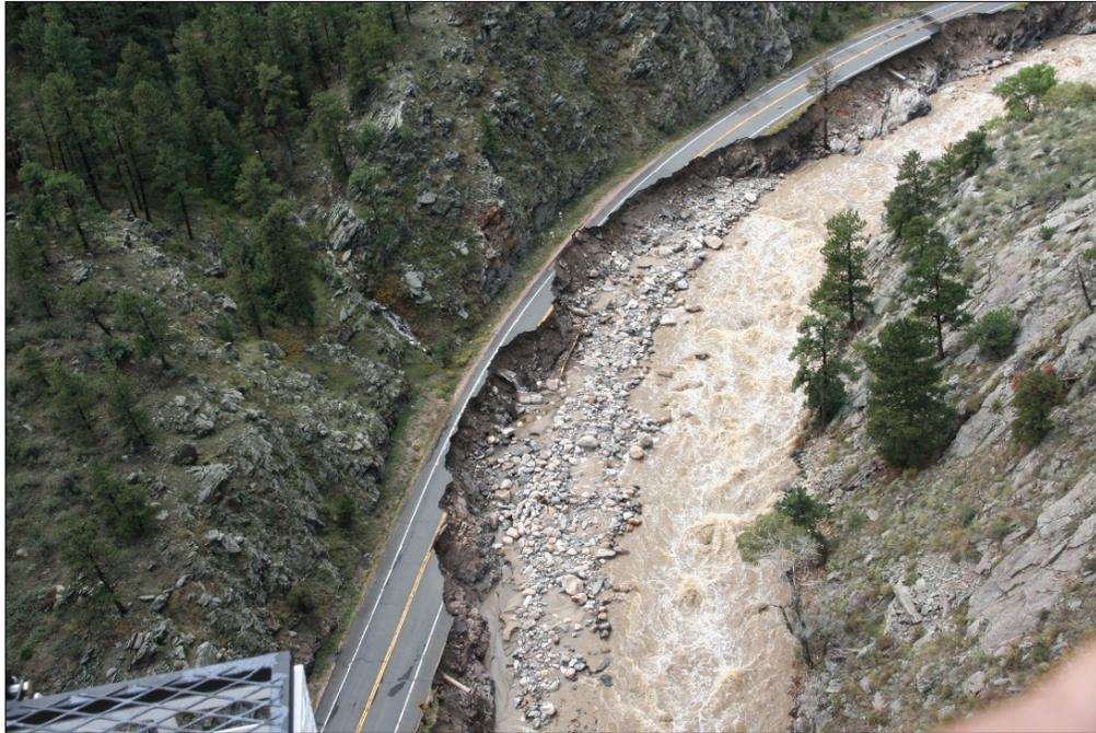
**Figure 3. Photograph of highway destruction after 2013 flood.**
