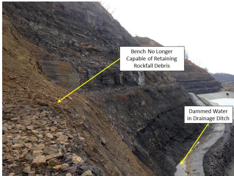
**Figure 6 – Heavy bench accumulation of rockfall debris. Bench can no longer retain additional rock blocks and soil, and they are being passed downslope.**
