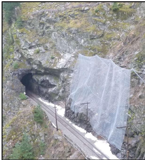
**Figure 2. Typical Attenuator installation showing a series of hinged posts with support cables, and a freely hanging net.**
