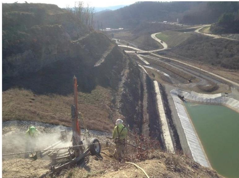
**Figure 13 – Drilling cable anchor with wagon drill.**
