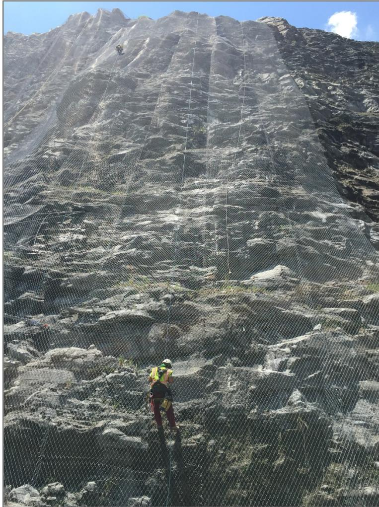
**Figure 2 – Constructed rockfall drape
