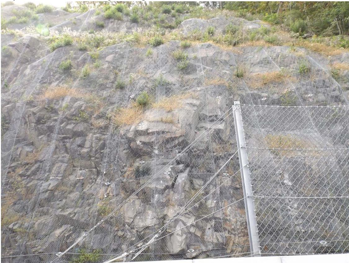
1. Combined drapery mesh and rockfall barrier for rockfall mitigation
