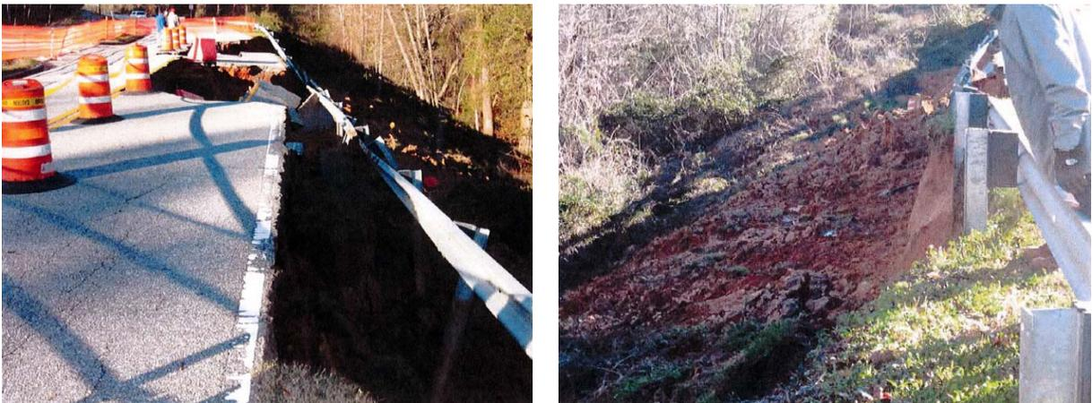
**Figure 9 (left): Slope failure undermining roadway platform**
