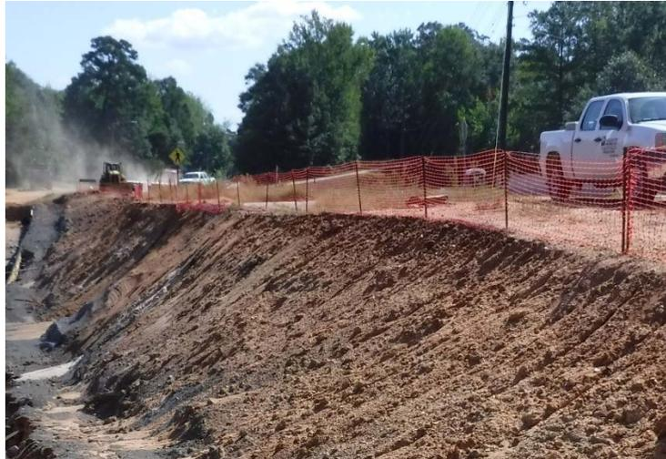
**Figure 22: Slope prepared to begin construction of GCS wall**
