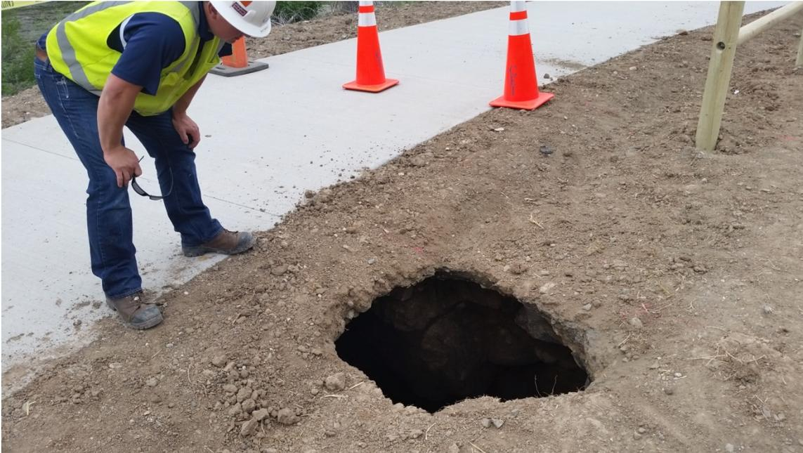
**Figure 8 – A collapsed void was encountered during installation of a fence.**
