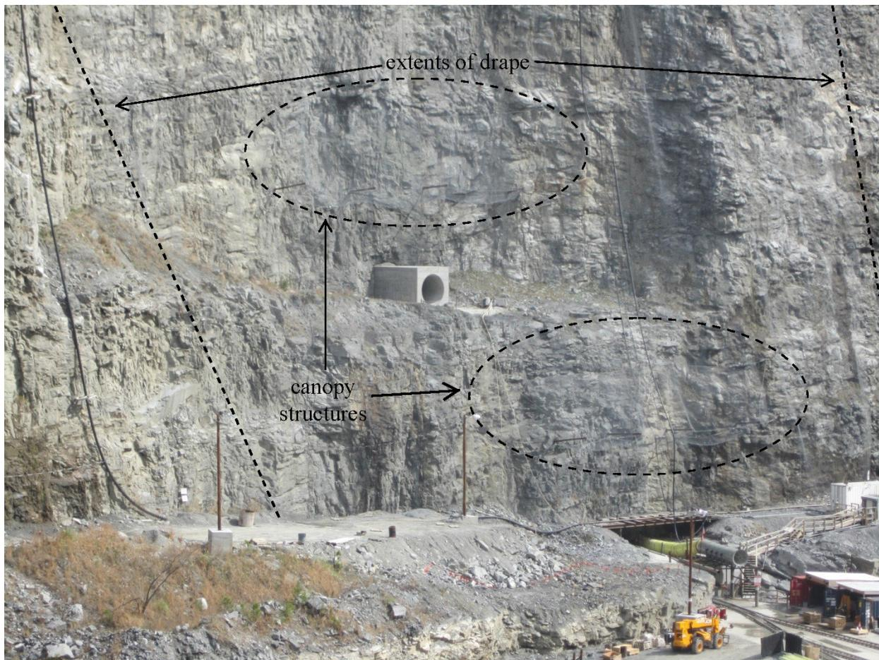
Figure 6. General area of tunnel portal stabilization area and the two canopies.
