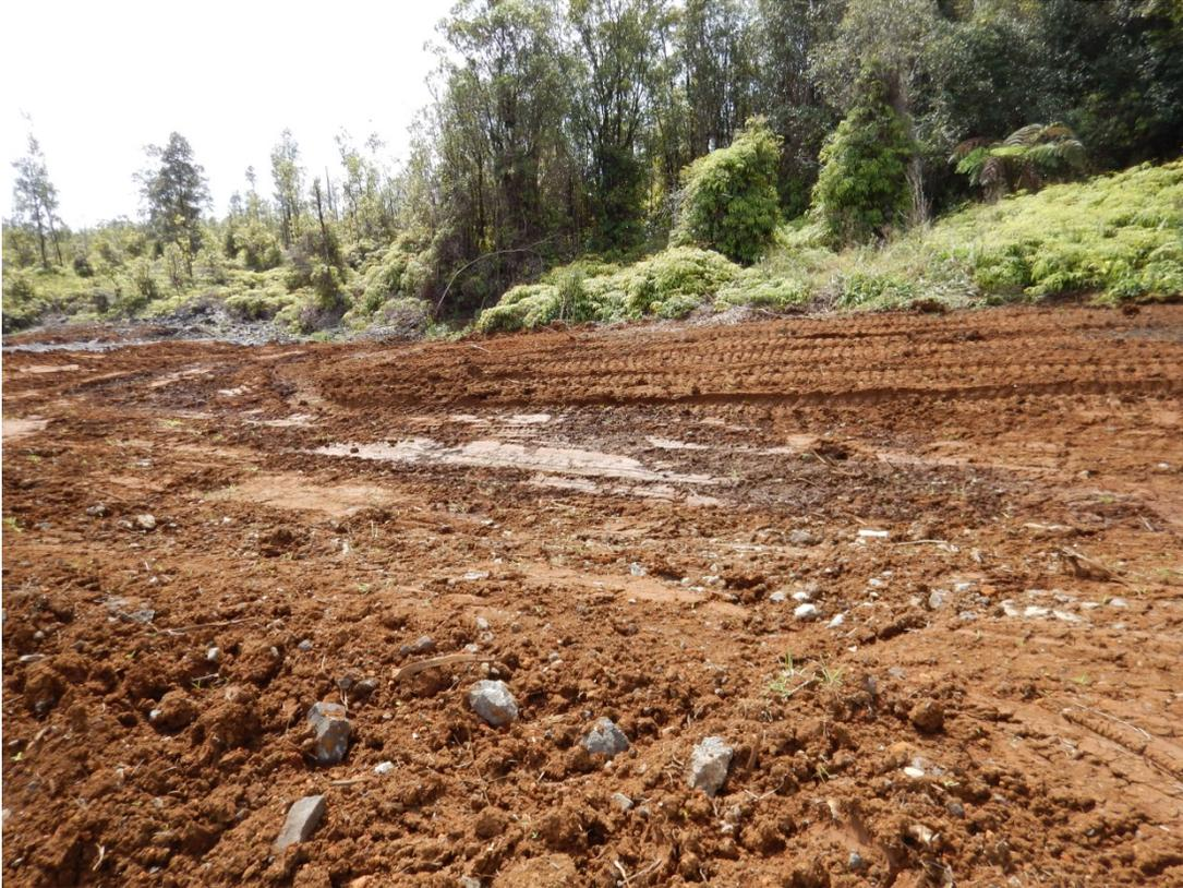
**Figure 6 - Weathered ash material exposed during construction of the Saddle Road, East Side project. Note the degree of rutting and sheen visible.**
