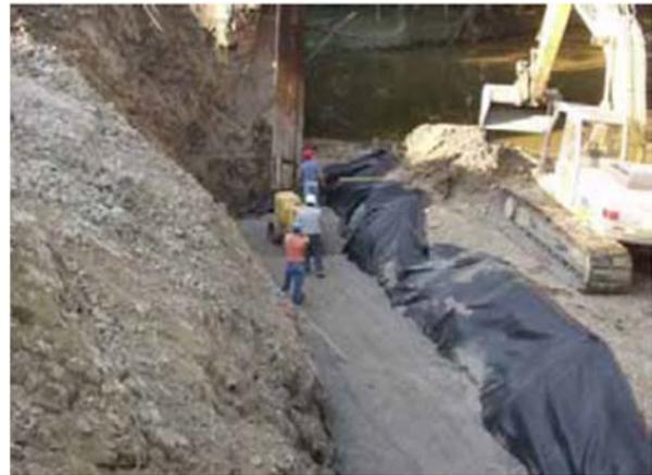
**Figure 3 (left): Site excavated and ready for GCS wall foundation**
