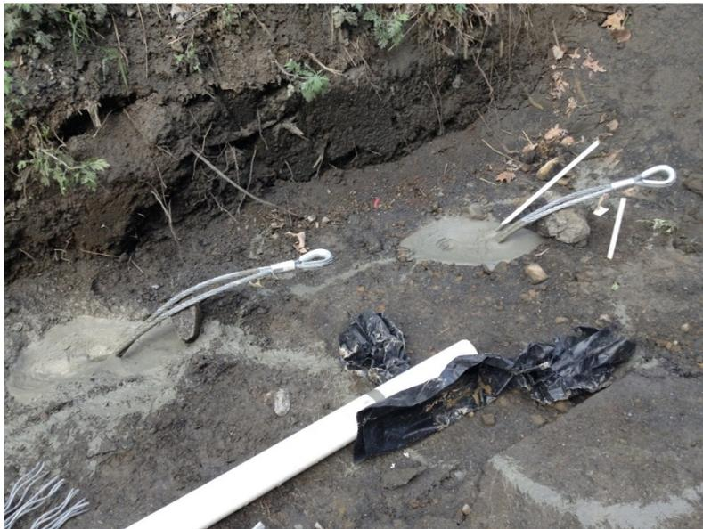
**Figure 6 – Anchor Pair After Tremie Grouting**
