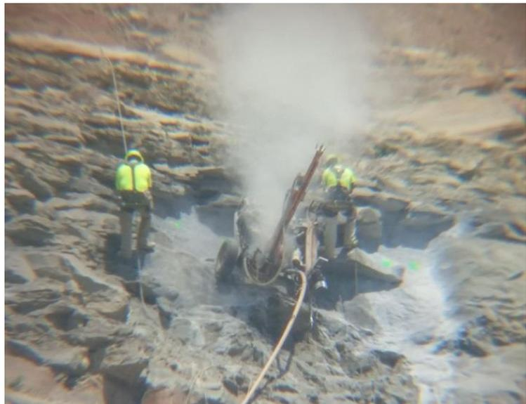
**Figure 11 – Drilling shotcrete support dowels.**
