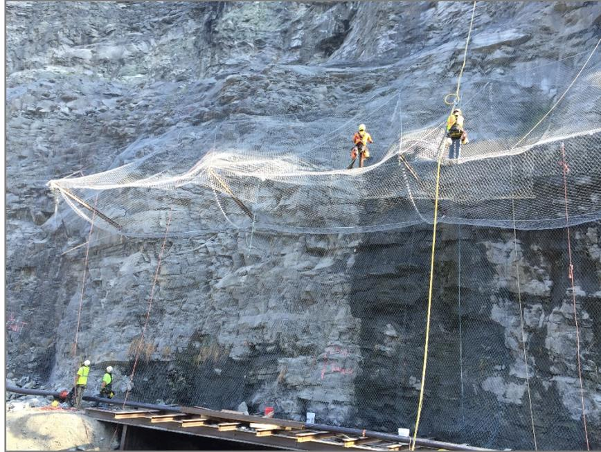
**Figure 5 – Canopy construction and drape tie-in
