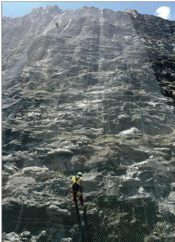
Figure 2. Constructed rockfall drape.
