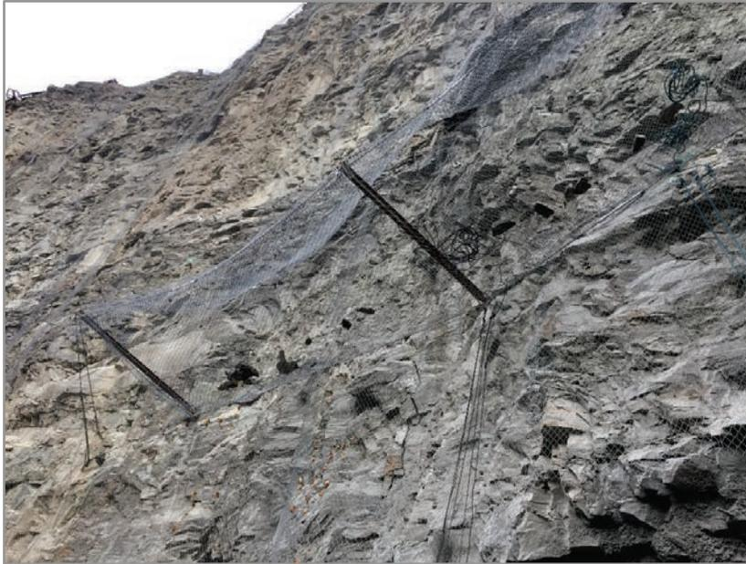
Figure 6. Adit canopy rock debris subject to maintenance cleaning.
