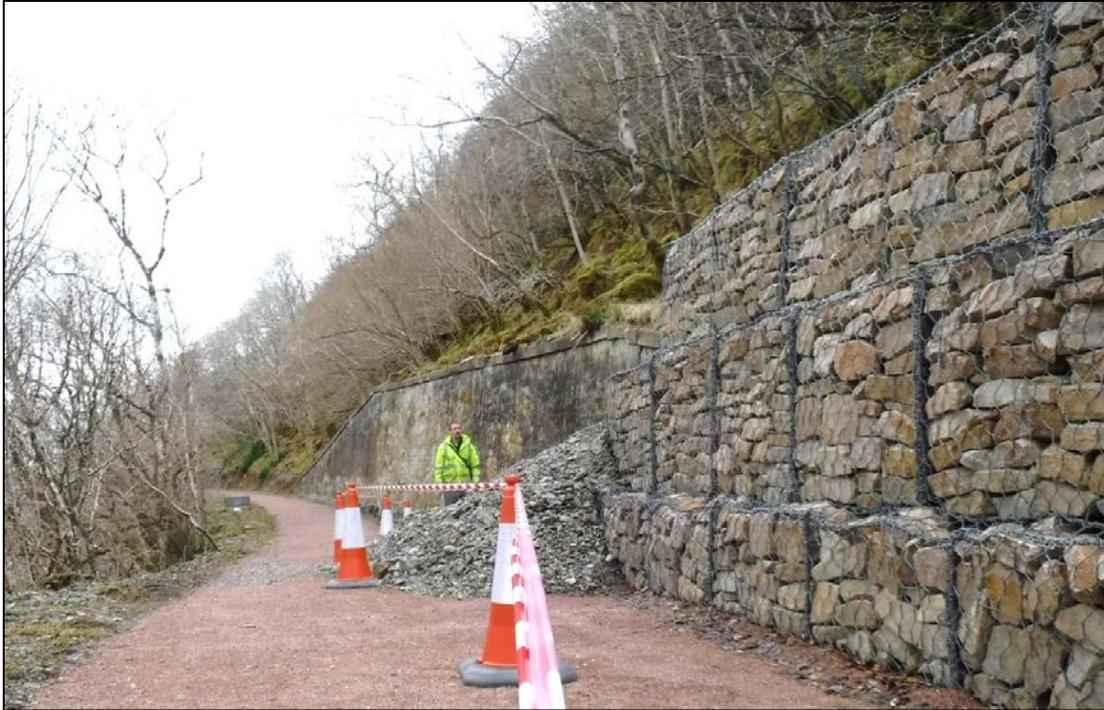
**Figure 9: Northern end of the embankment after the impact, showing overspill of debris.**
