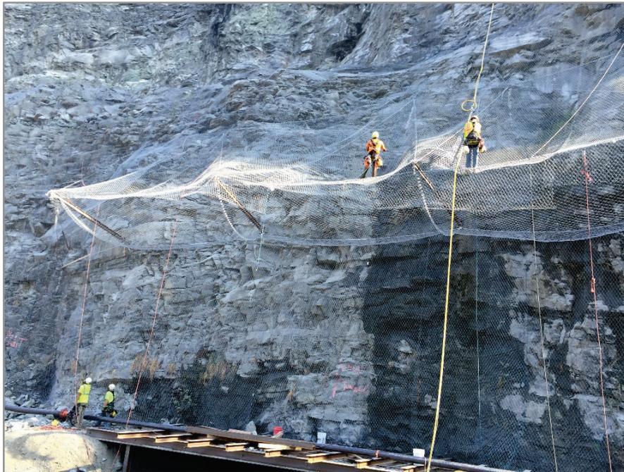
Figure 5. Canopy construction and drape tie-in.
