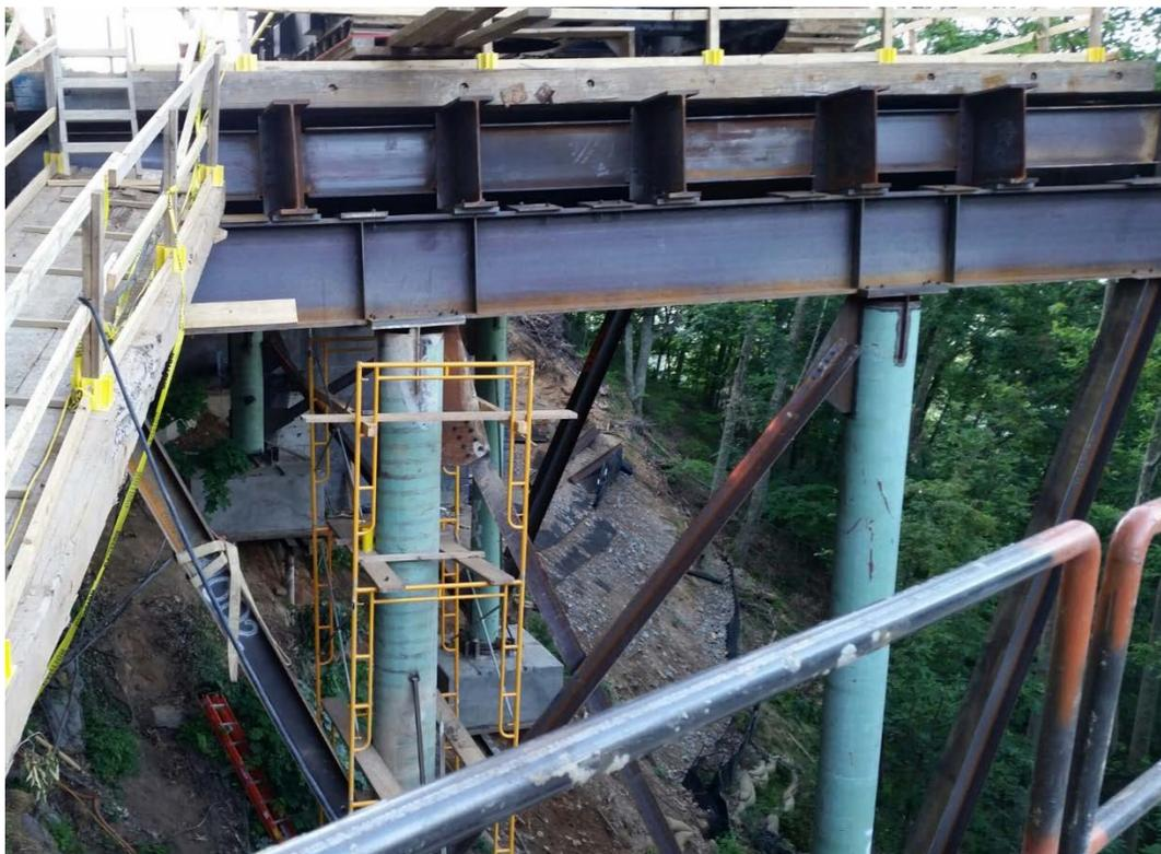
**Figure 8 – Temporary Falsework**
