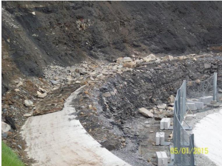
**Figure 9 – Scaled debris in concrete ditch resting on blasting mats and contained by temporary barrier.**
