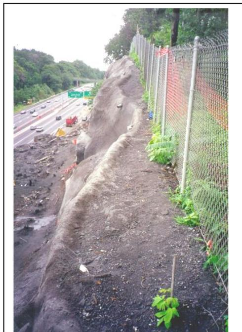
Figure 3 – Completed Wall, note presplit holes at the toe of the wall.
