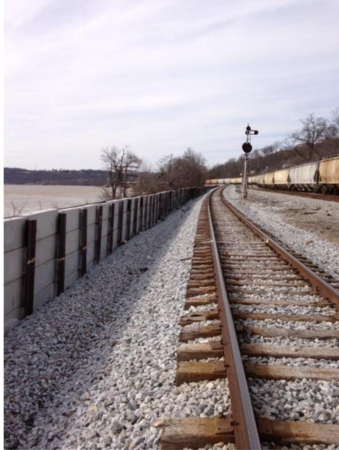
**Figure 5 – Soldier pile wall installed downslope of the railroad.**
