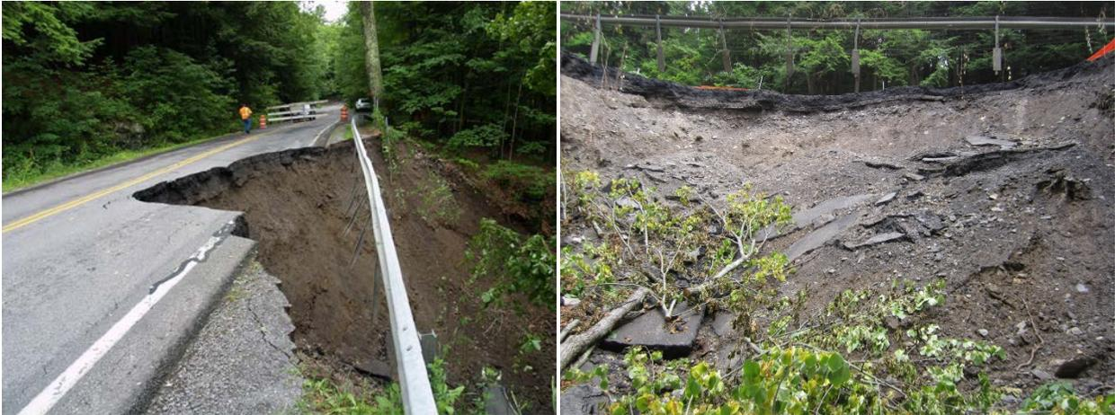
**Figure 1 (left): CR 31 Site condition upon initial site visit. The pavement in the foreground would later fall into the gap created by the landslide.**
