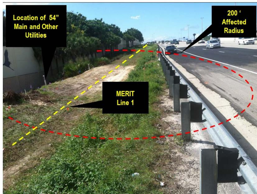
**Figure 1: Impact to roadway and infrastructure due to sinkhole**
