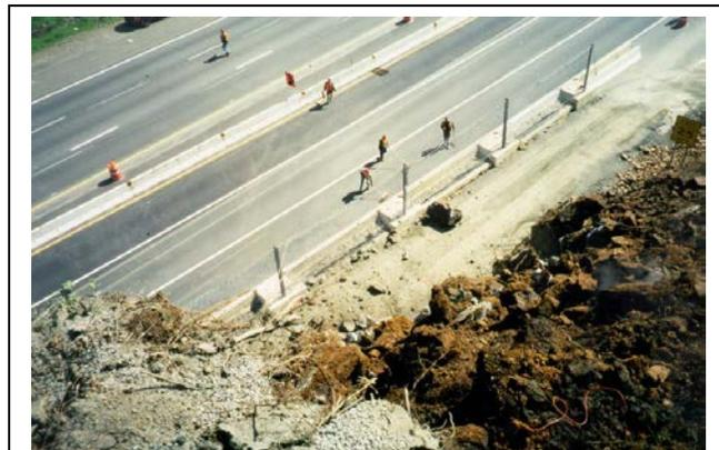
Figure 1 – Temporary Traffic and Rockfall Barrier
