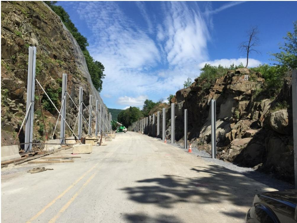
**Figure 9 – Completed Posts Prior to Mesh Installation**
