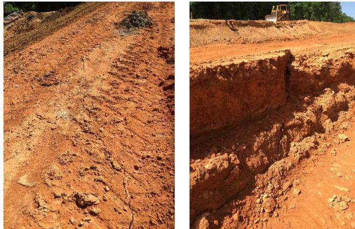
**Figure 17 (left): Stress cracking during slope reconstruction**
