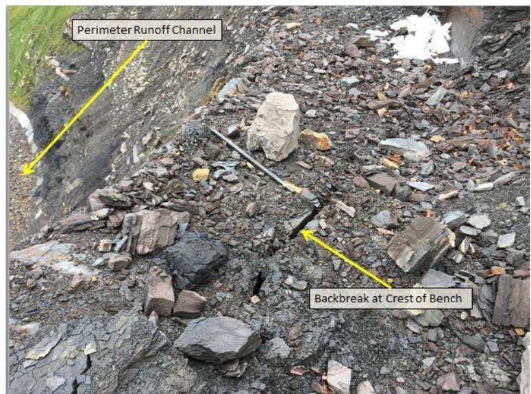
**Figure 5 – Backbreak along crest of bench above north end of perimeter runoff channel. Grade stake for scale.**
