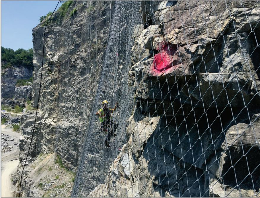
Figure 3. Rock dowel layout with paint using rope access.
