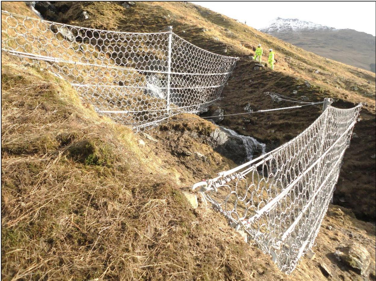
**Figure 5: Debris flow protection fences in Argyll, Scotland (courtesy Maccaferri UK).**
