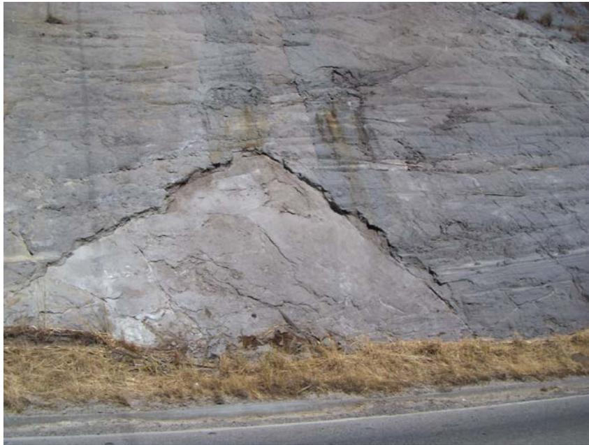
**Figure 4. Typical Surficial Failure on Bituminous Sandstone Slopes. Depth of Failure Surface is Approximately 8 Inches Below Slope Face.**
