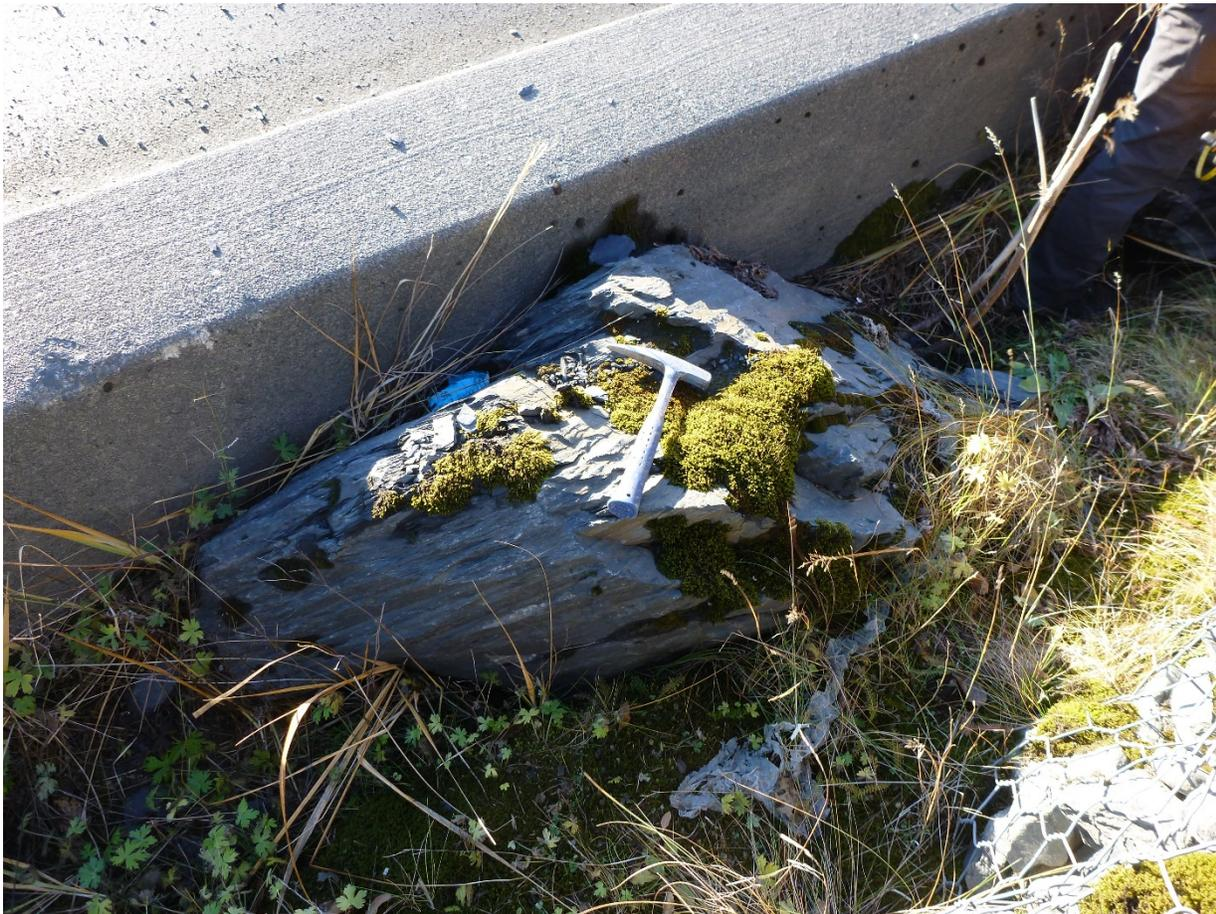
**Figure 5 – Example of Rockfall Block Downslope of Gabions at Base of Pillar Mountain Slide (Rock Hammer Approximately 1 Foot Long for Scale)**
