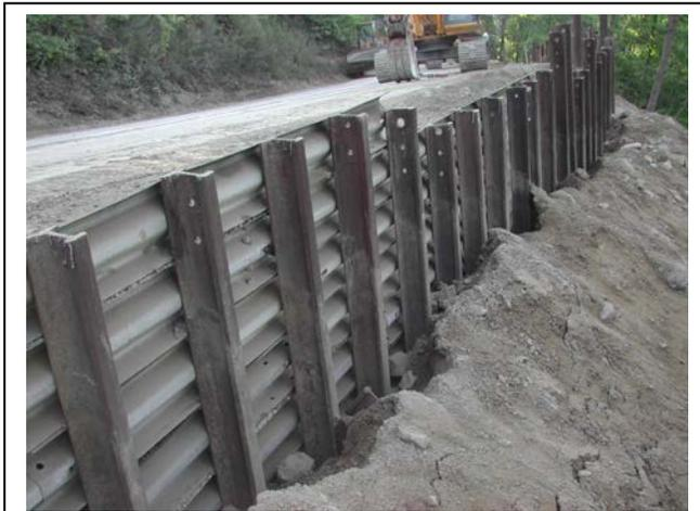
Figure 5 – Railroad Rail Wall Embankment Stabilization
