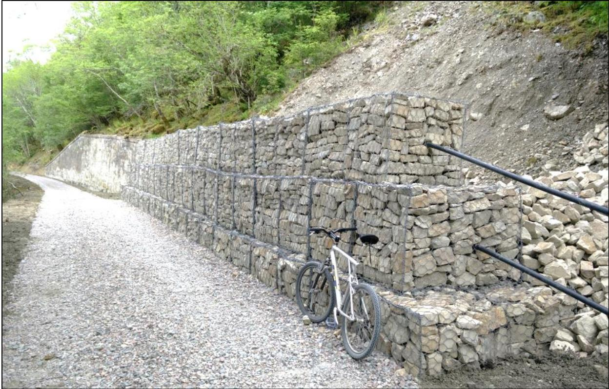
**Figure 8: Photograph north showing the completed Parafil® reinforced gabion embankment adjacent to the cycle path. Rope ducts are visible to the right.**
