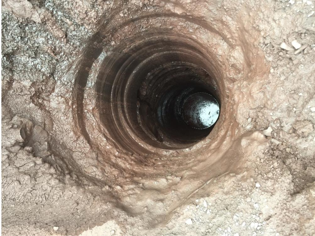
**Figure 8 – Typical Caisson With Shallow Bedrock**
