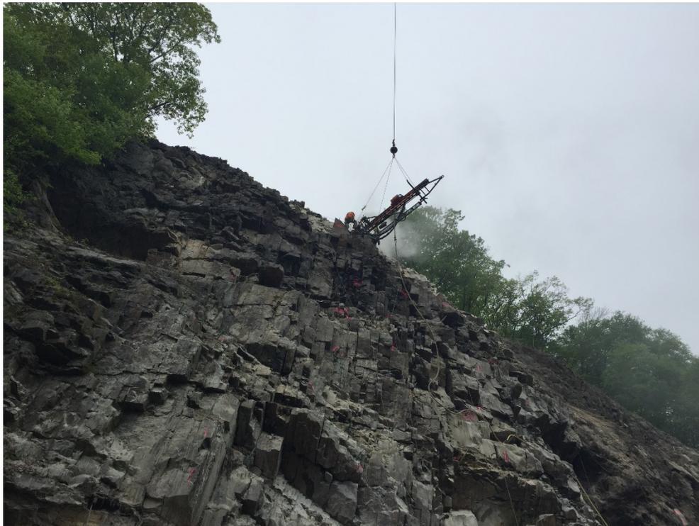
**Figure 4 – Rock Bolt Installation on Steeply Dipping, Thinly Bedded Sandstone**
