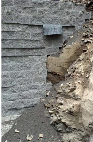
**Figure 9: Facing block placement around rock outcrop**
