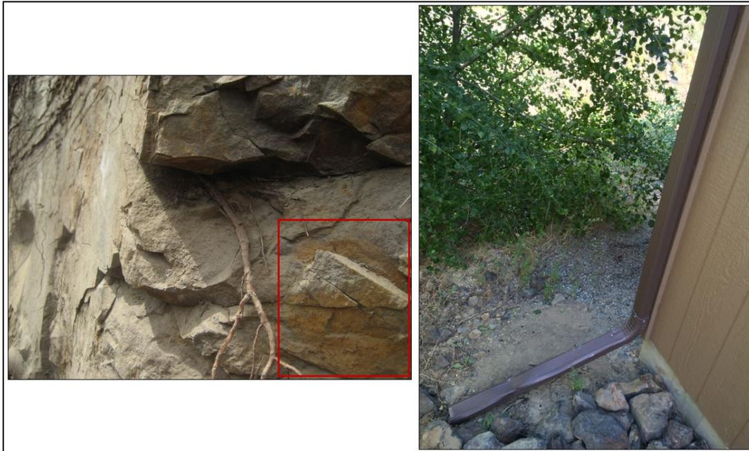
**Figure 8 – Oxide staining evidence from surface water infiltration into the rock mass (left). Downspouts from the residents on the brow of the slope (right).**
