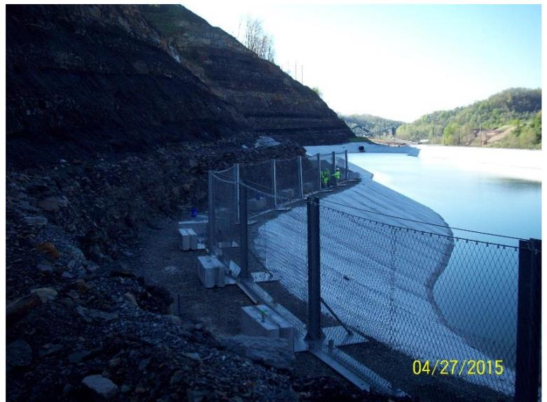
**Figure 8 – Temporary rockfall barrier.**
