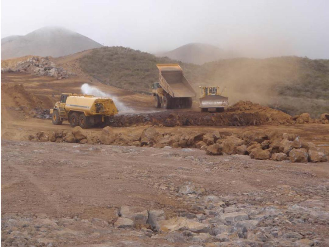
**Figure 7 - Mixing ash and rock to achieve compaction and stable embankment subgrade for Saddle Road, West Side project.**
