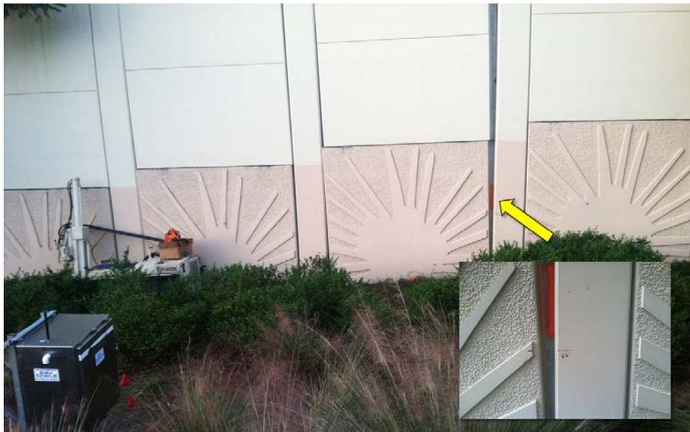
**Figure 3: Shows the amount of movement of the sound barrier and DPT installation**
