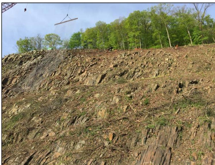
9. Moveable rockfall drapery used during scaling
