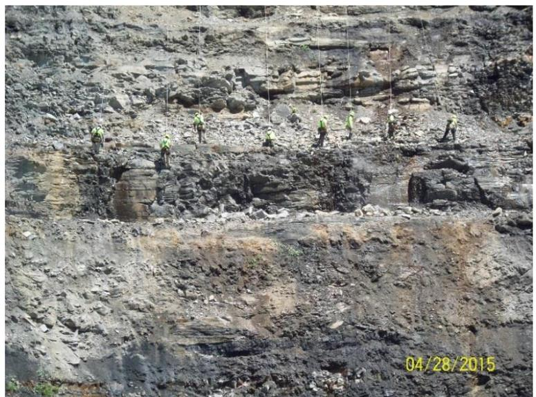
**Figure 10 – High scalers scaling rock face.**
