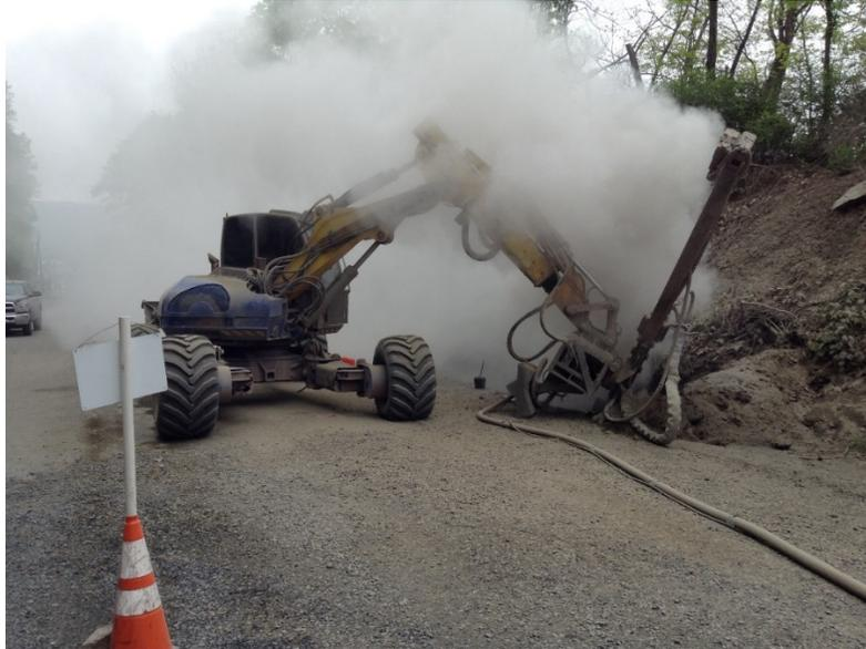
**Figure 5 – Drilling Ground Anchors with Articulated “Spider” Drill**
