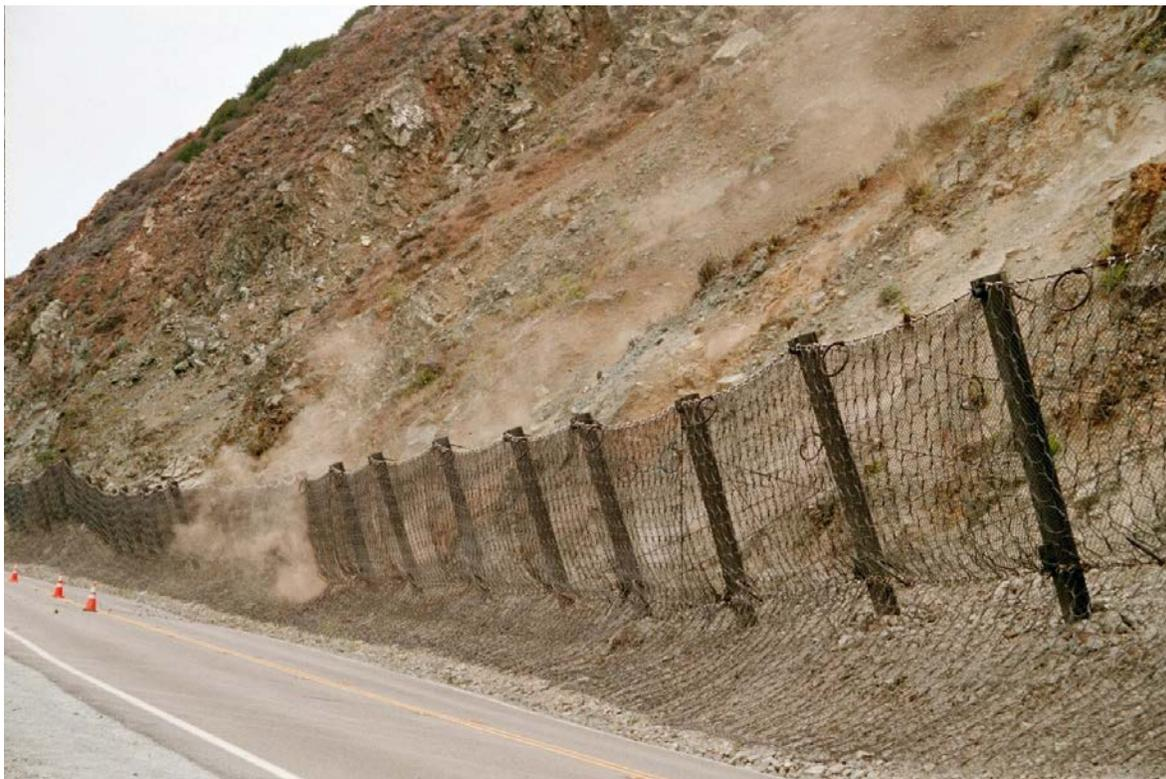
**Figure 8 – Rockfall Barrier Live Demonstration Cow Cliffs (US-1, Big Sur) – 53<sup>rd</sup> HGS Field Trip 2002**
