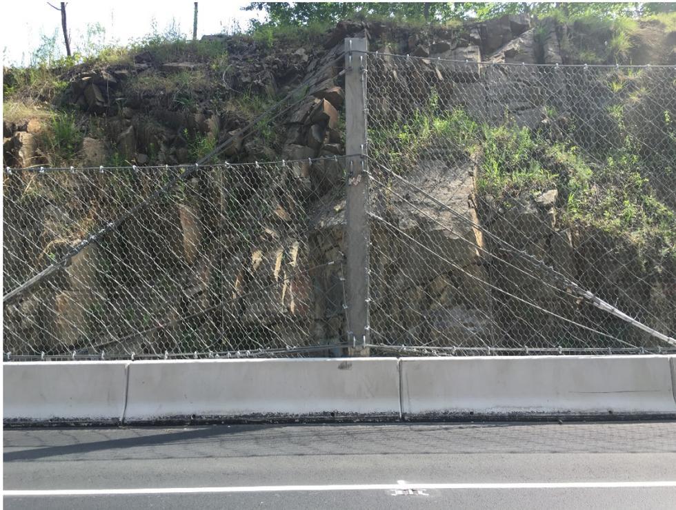
**Figure 10 – Completed Fence Section at Height Transition Post**
