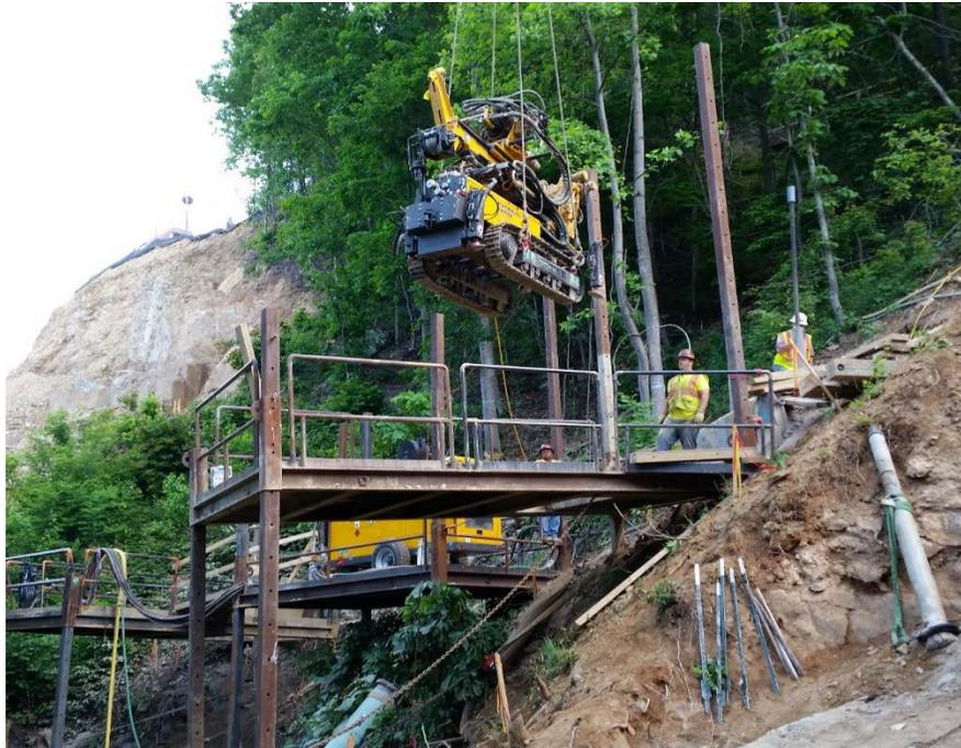
**Figure 7 – Setting Drilling Rig on Temporary Platform**
