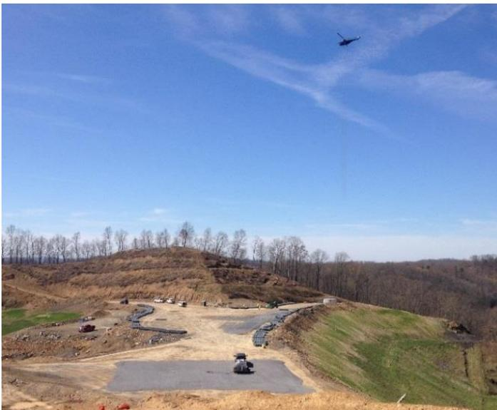
**Figure 15 – Drape assembly/staging area and pick.**
