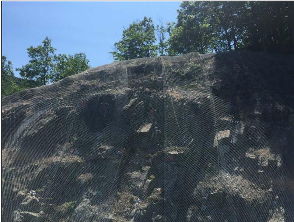
13. Tensioned Spider mesh overlaid by TECCO drapery mesh
