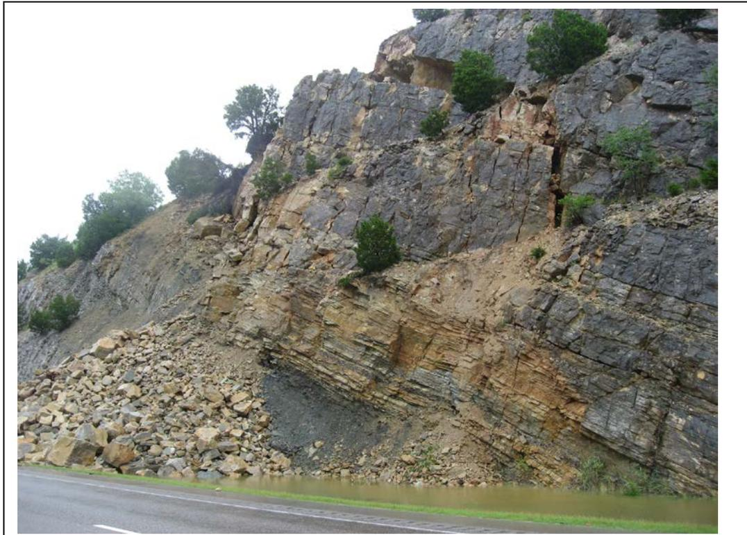
Figure 6 – I-35 Rockslide and destabilized slope, Arbuckle Mountains
