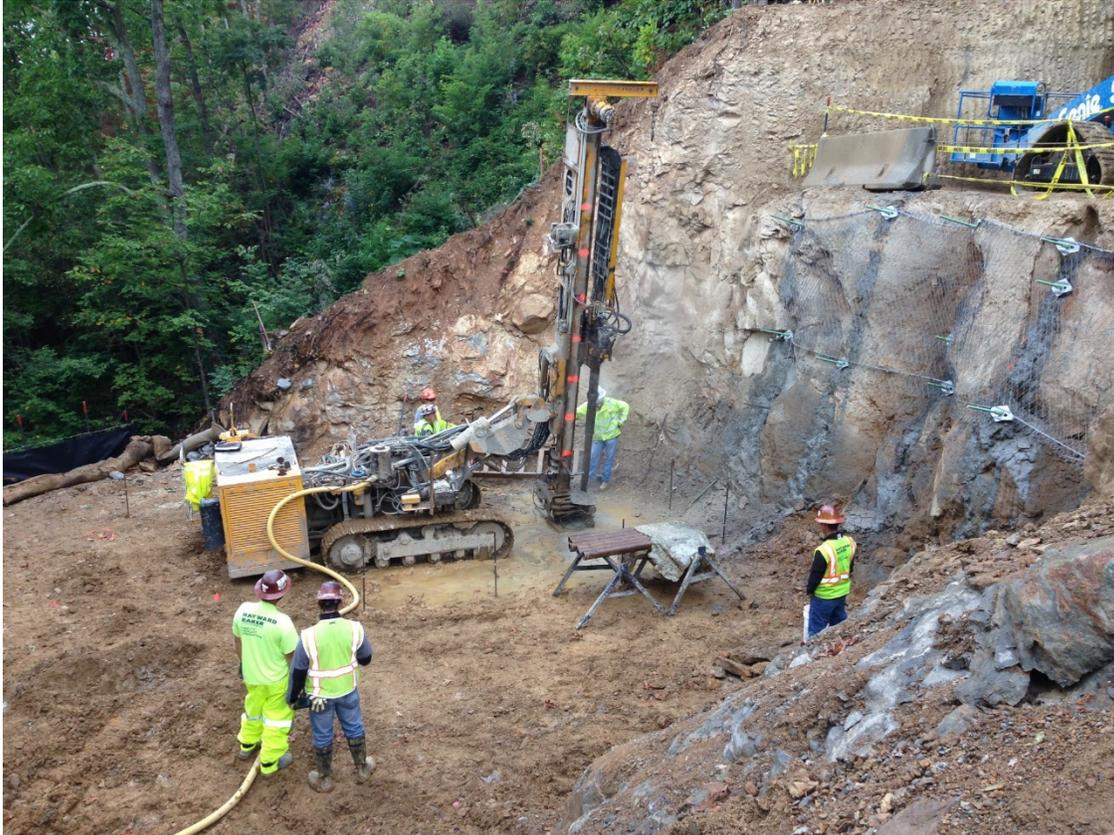
**Figure 6 – Bridge Abutment Micropile Installation**
