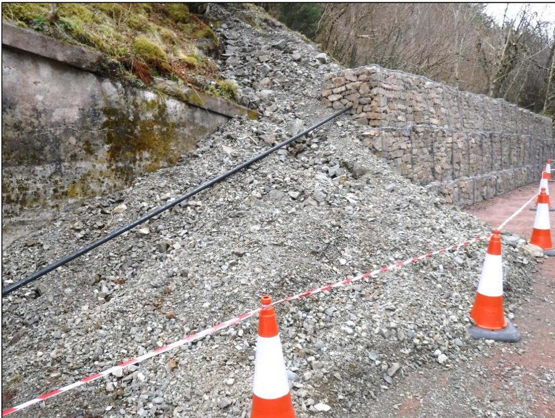
**Figure 10: View of the northern end of the embankment showing the overspill of material arising from the second phase of the debris flow impact**
