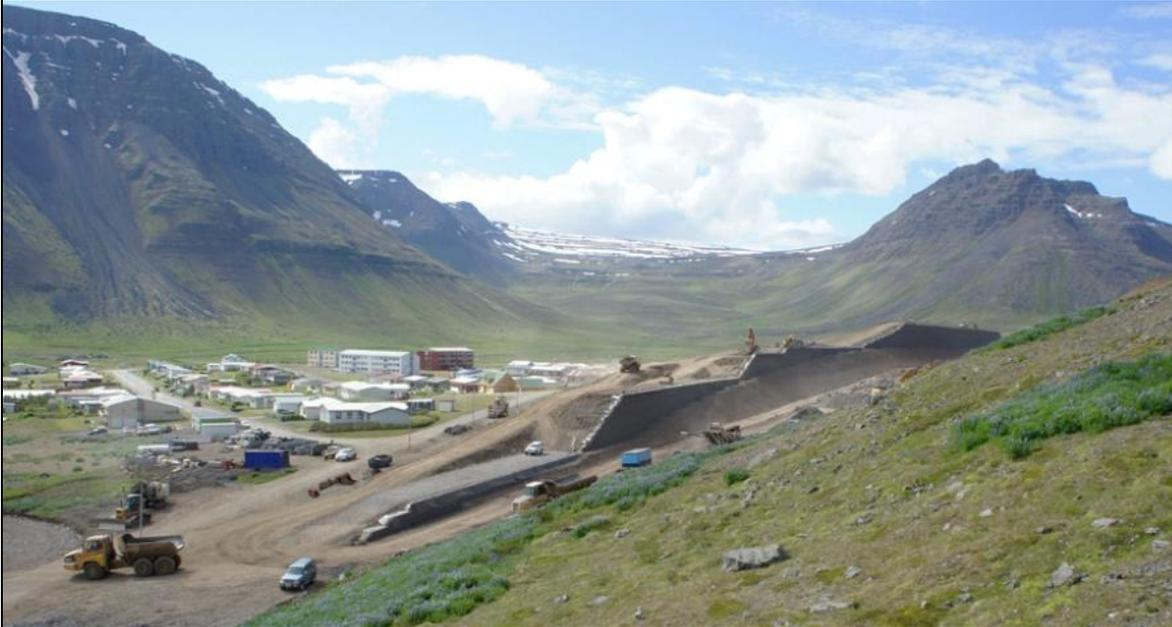
**Figure 6: 22m high x 750m long reinforced soil embankment construction, Iceland.**
