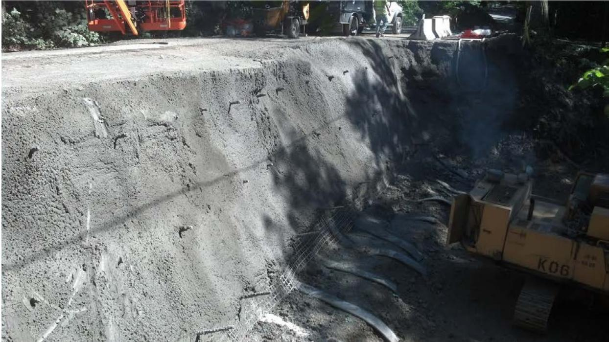
**Figure 8: Soil nail wall in progress**
