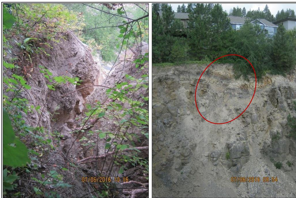
**Figure 5 – Tension fracture, west side of Fossil Cut on the brow of the slope (left). Head scarp on the west side of Fossil Cut and offset of Latah bedding (right).**
