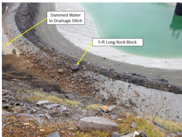
**Figure 3 – Rockfall debris accumulating in drainage ditch, perimeter roadway, and concrete liner. Note ponded water in ditch dammed by debris on far left side of photo.**
