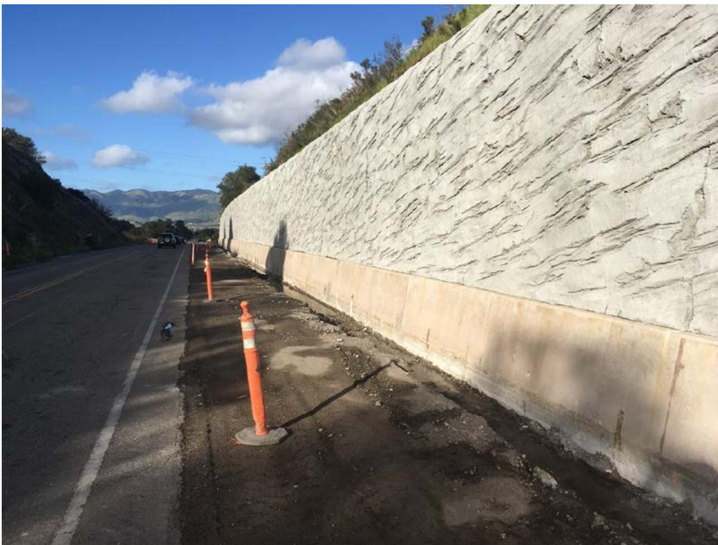
**Figure 9. Constructed Rock Dowel Wall with Architectural Treatment (facing north)**
