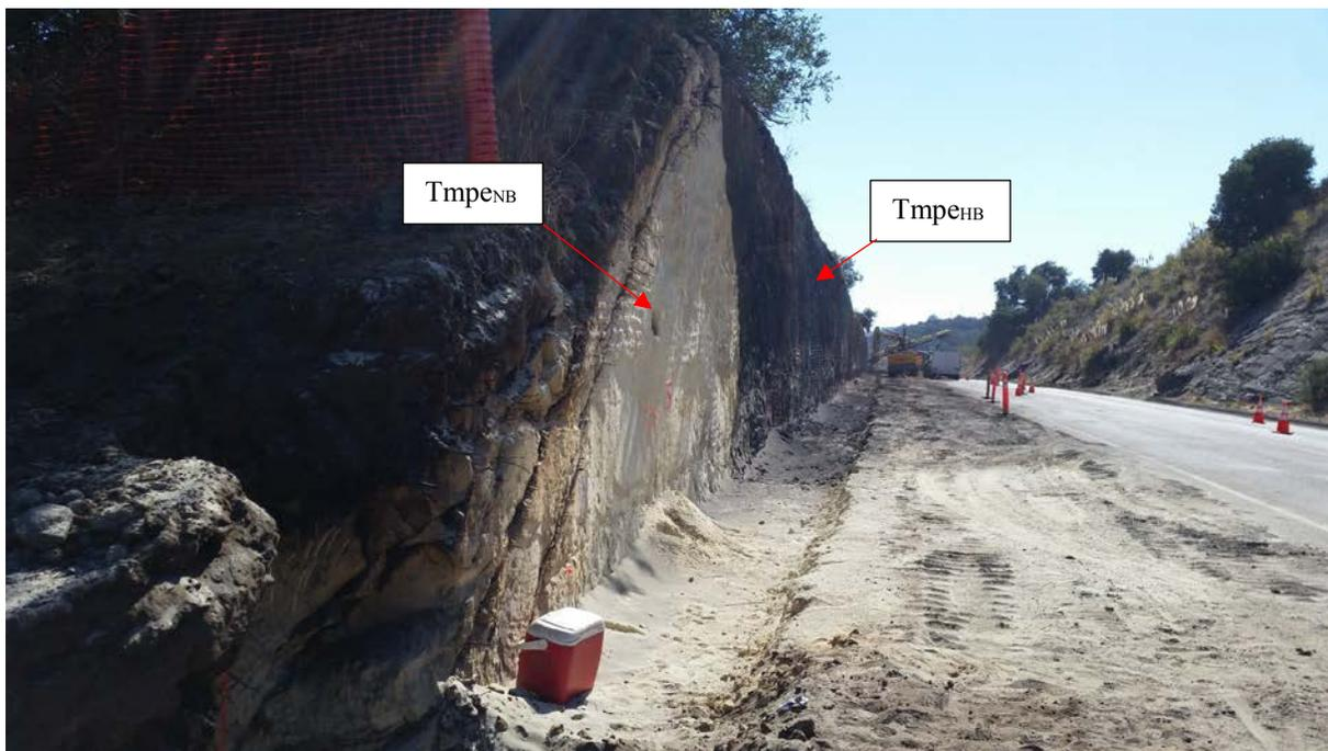
**Figure 8. Excavation of The Wall Alignment (Facing South). Note Non-Bituminous Sandstone in Foreground. Heavily-Bituminous Sandstone in Background.**
