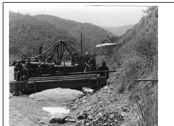
Figure 4 – I-40 Horizontal Drain Installation
