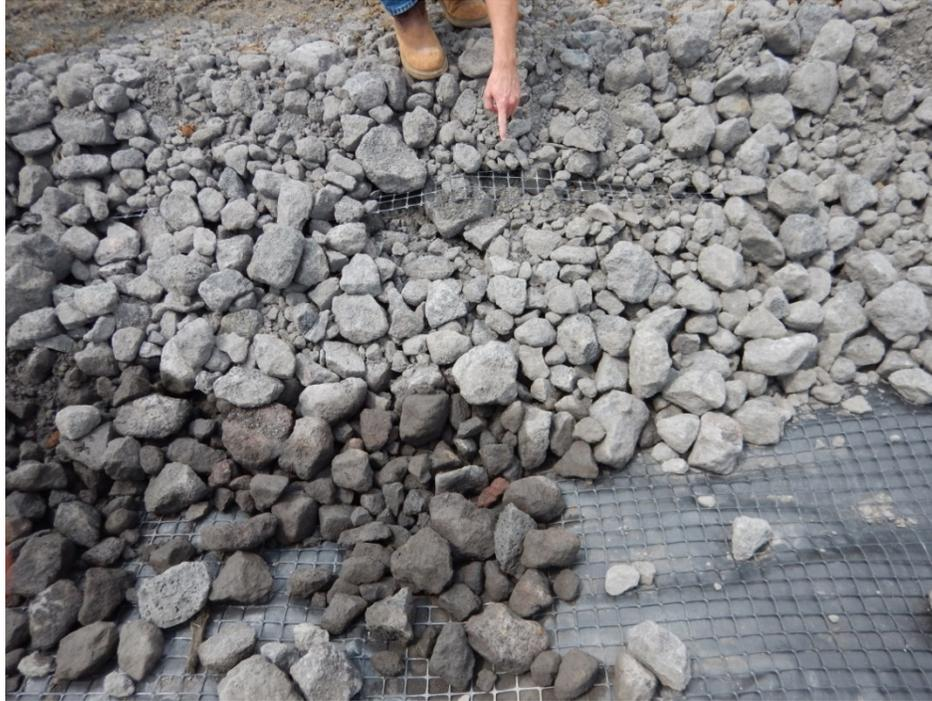
**Figure 9 - Installation of reinforced section including geotextile, two layers of geogrid, and crushed rock (select topping) material.**
