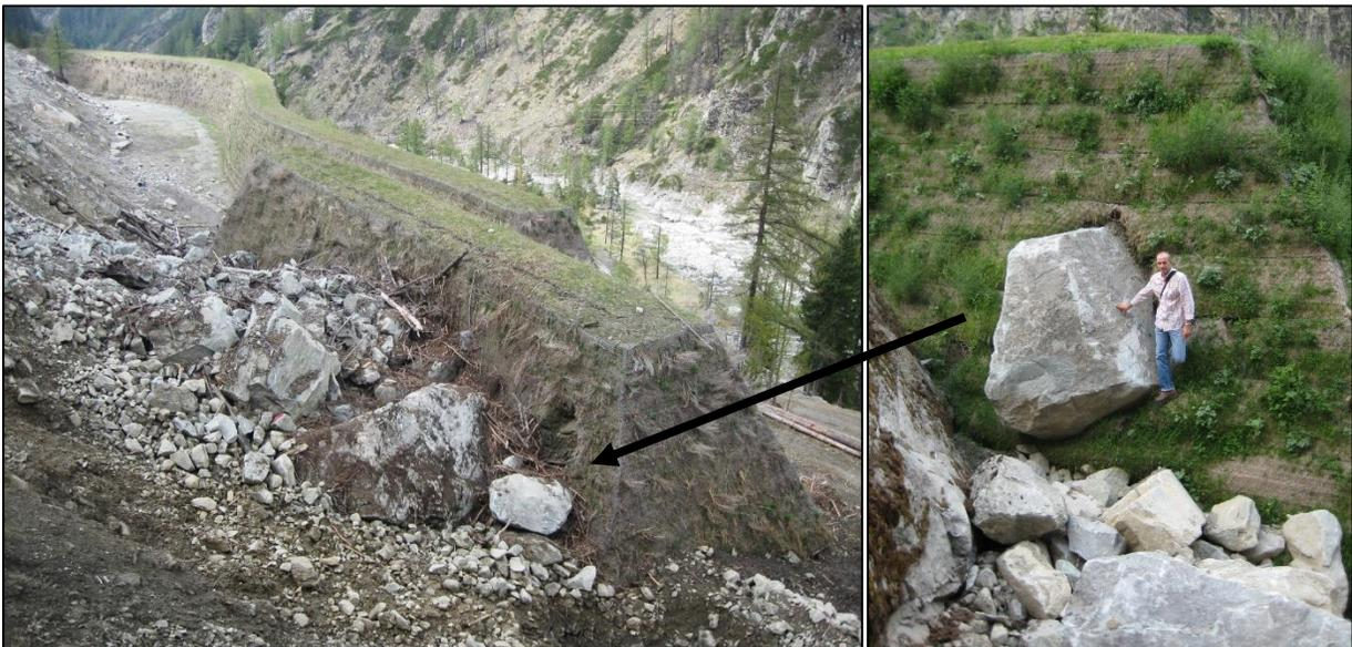
**Figure 7a and 7b: avalanche and rockfall debris accumulated behind a 12m embankment.**
