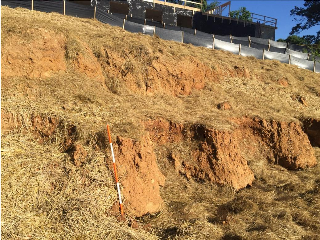
Photo 2: July 11, 2016 - Looking uphill with the house construction in the background and the DSW in for ground. Scale rod with 1-foot increments placed at Caisson 1.
