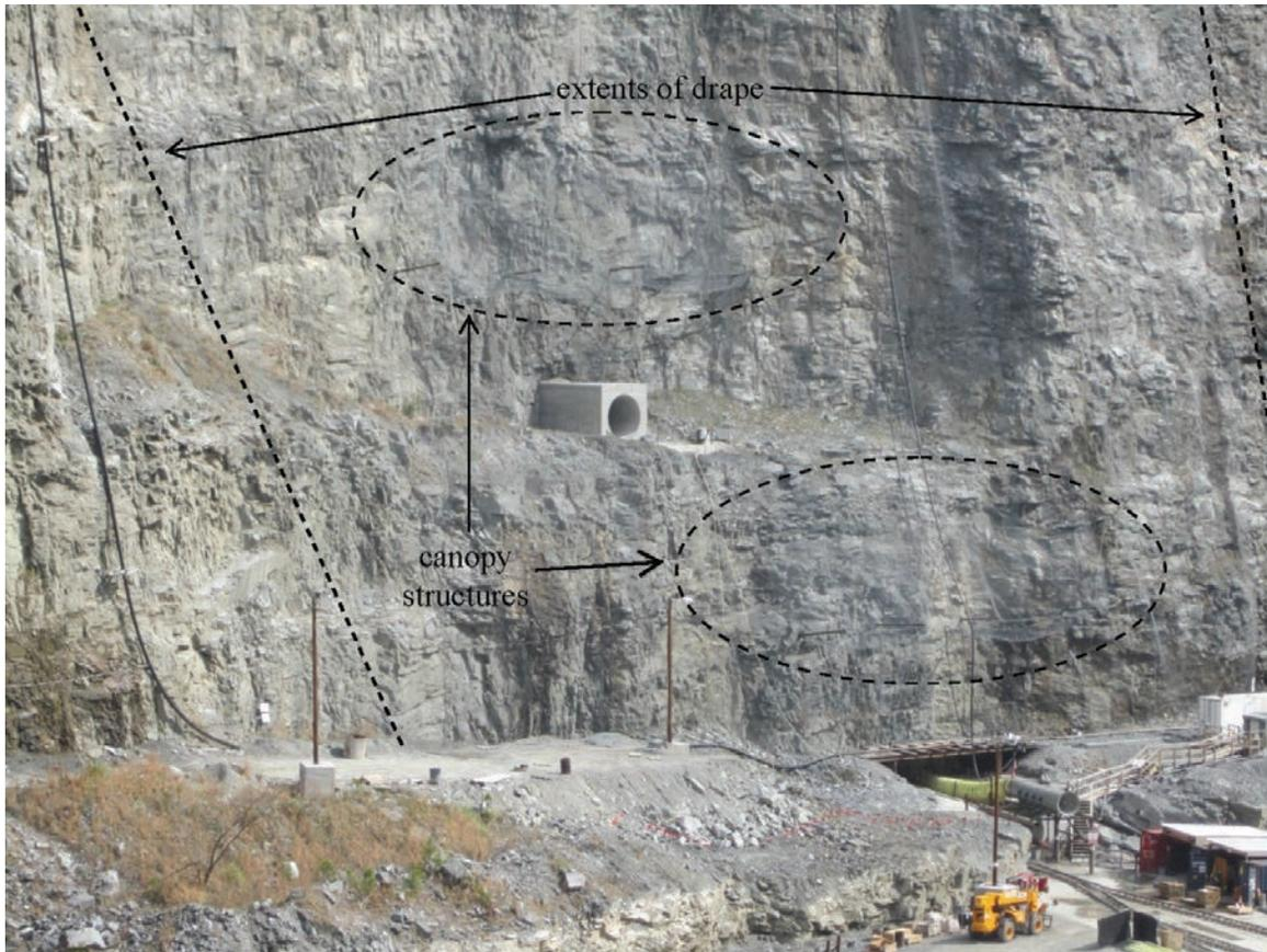
Figure 5. General area of tunnel portal stabilization area and the two canopies.
