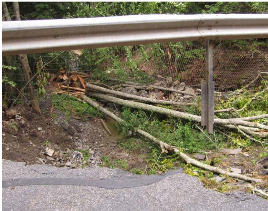
**Figure 4: Ponded water was present in the debris at the base of the slide. The existing stream entered the debris from the right of this photograph and continued downslope behind the tree stumps.**
