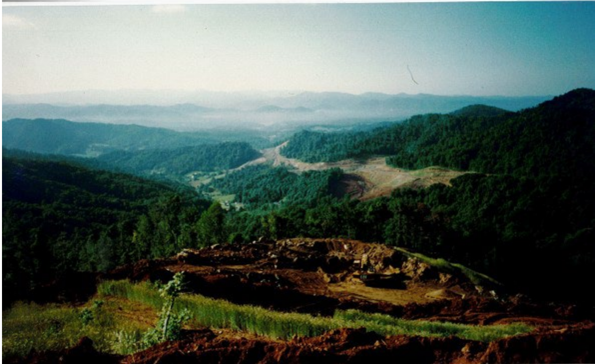
Top lift of Buckner Gap cut construction, looking South toward Asheville.
