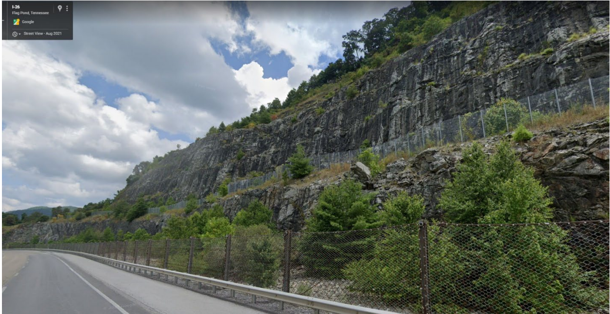
The Tennessee section of I-26 was completed 4 years before NC. Notable difference is the use of benched slopes and stacked rockfall fences.
