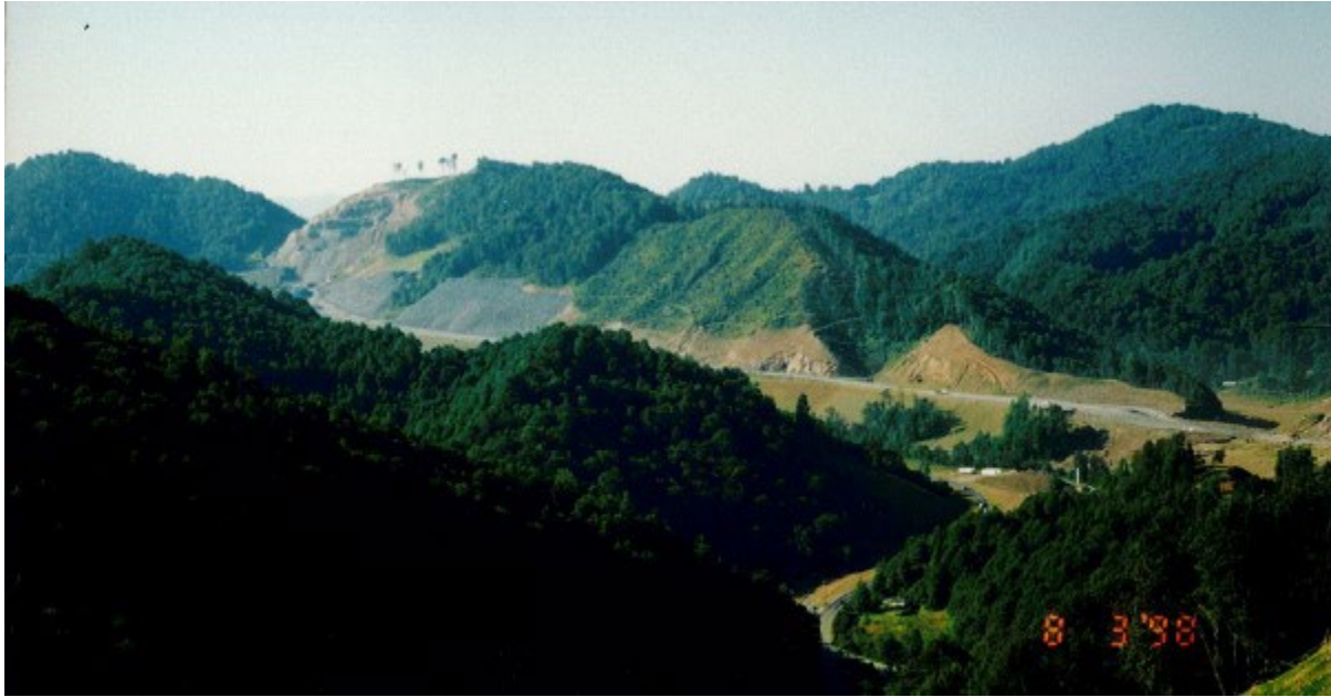
Looking toward Buckner Gap from the north. Cleared gap in distance. Large rock buttresses visible for soil slope support between rock cuts.
