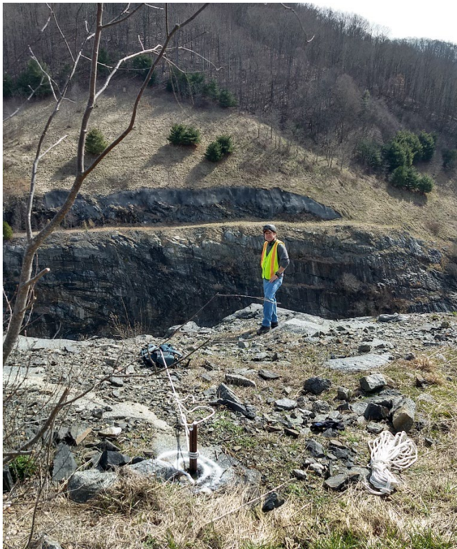
During construction holes were drilled across the benches to provide future rope access points, such as this Lidar study in 2020.
