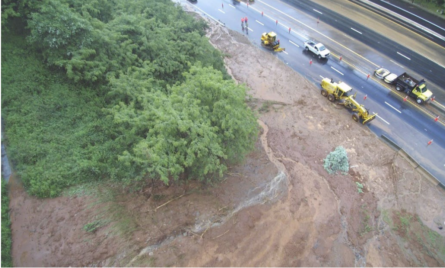
Slide runout with groundwater, mud, and weathered rock.
