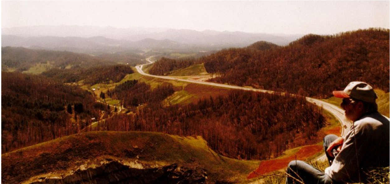
Russell Glass looks over final paving of I-26, Madison Co.
