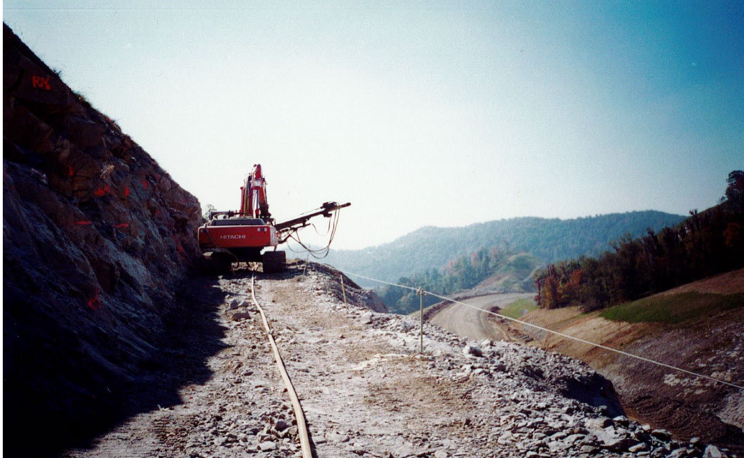
Buckner Gap, east face. Anchor and shotcrete stabilization.
