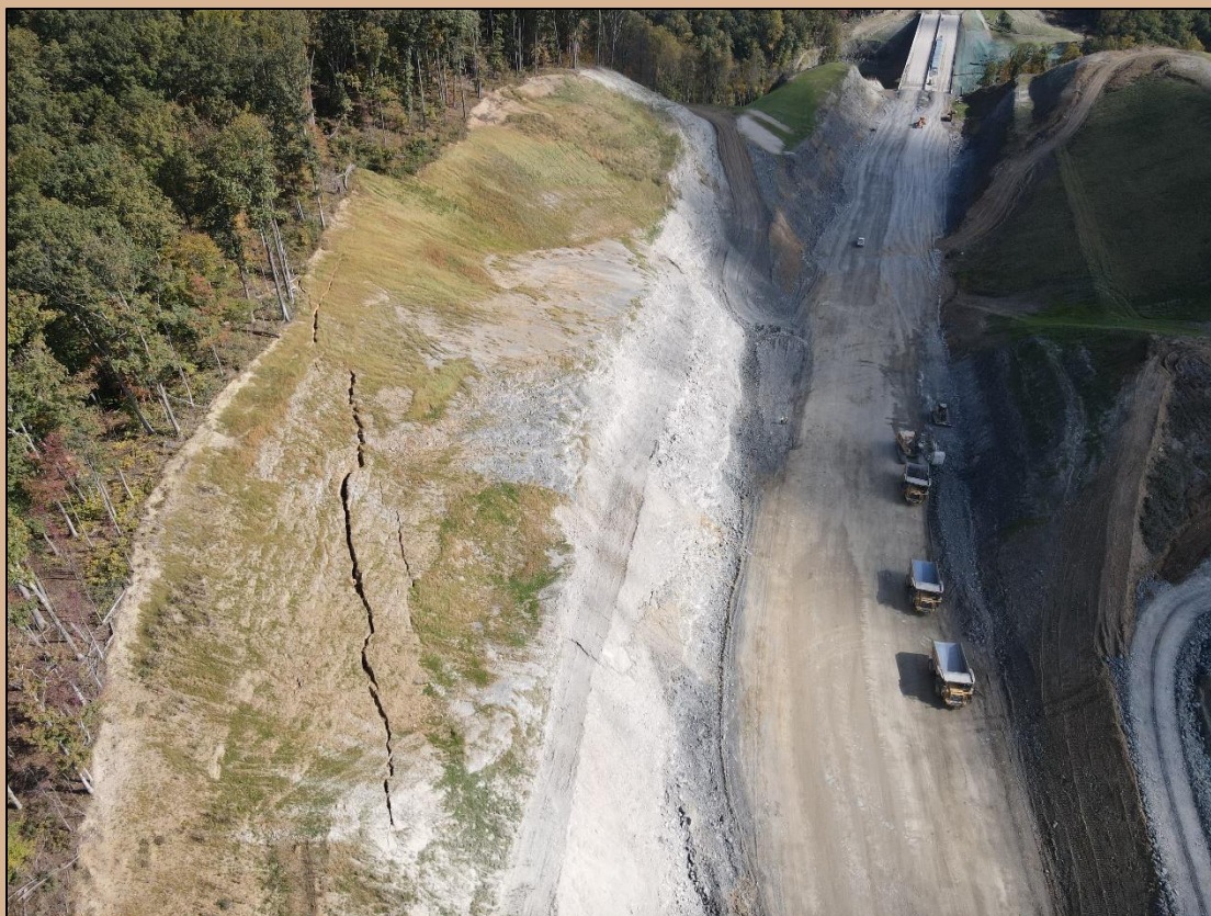
Figure 53. An aerial view of the slump blocks partway through the construction process at Cut 29. Photo provided by John Lasko.
