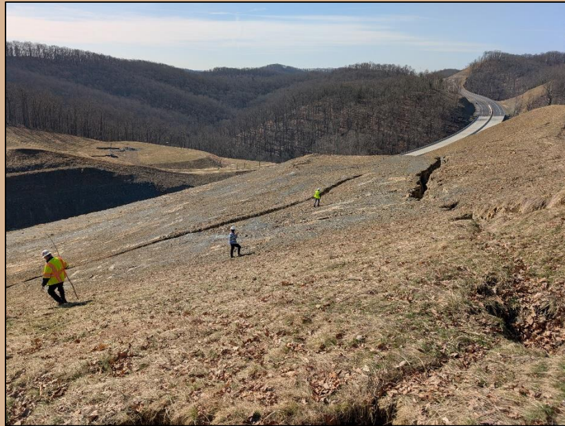
Figure 58. View of the latest cracks at Cut 29 looking downhill from the "Big G."
