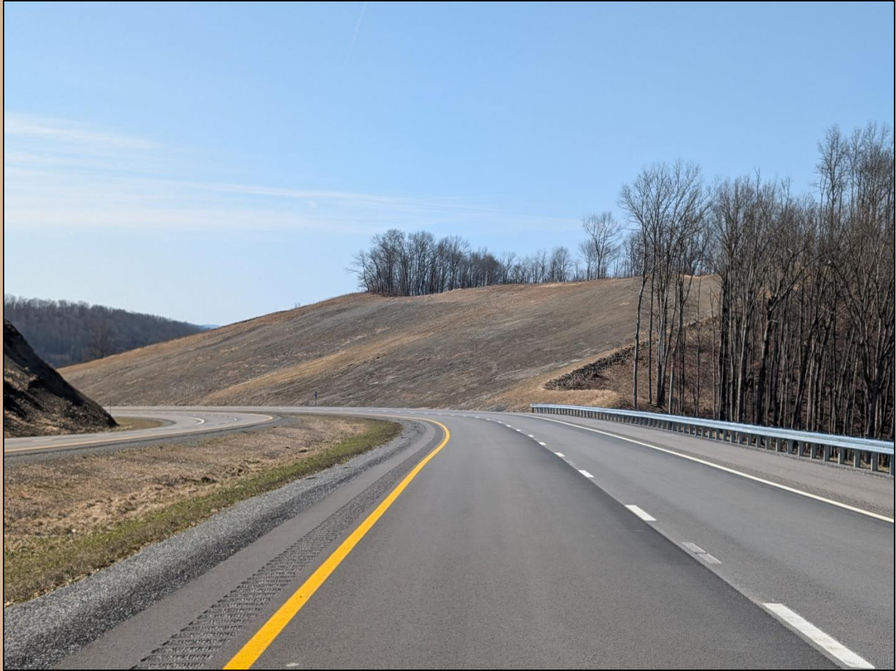
Figure 61. A view of a large bedding failure near the end of the unopened section of Corridor H.
