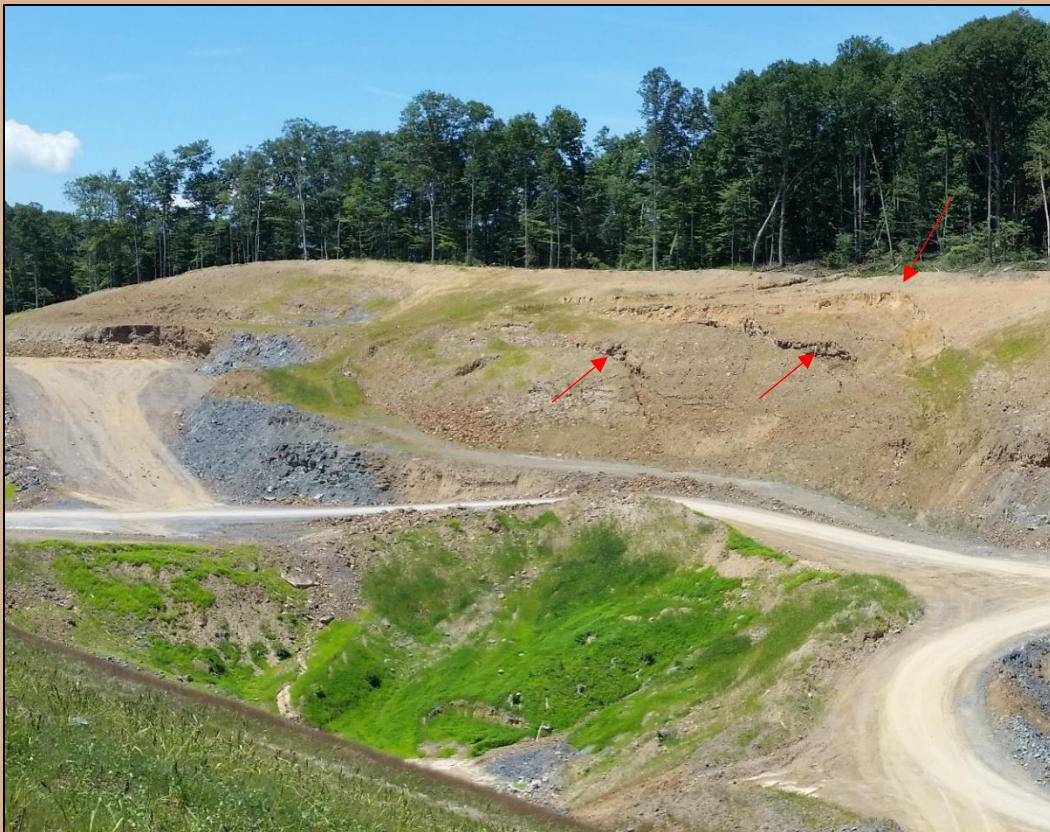
Figure 52. Cracks forming at the top of the large slump blocks (indicated by red arrows) during the early construction phase of Cut 29. Photo provided by John Lasko.
