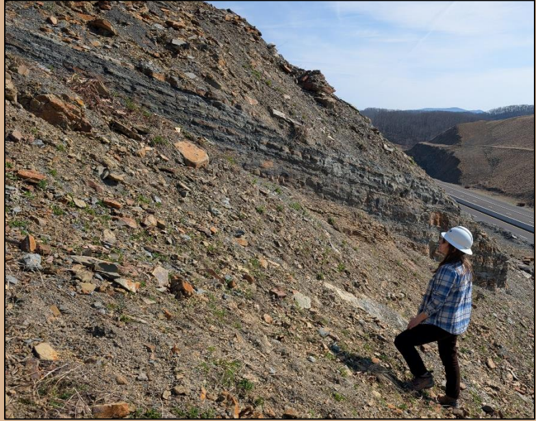
Figure 51. Steeply dipping strata (to the southeast) at Cut 29 with the finished roadway in the background.
