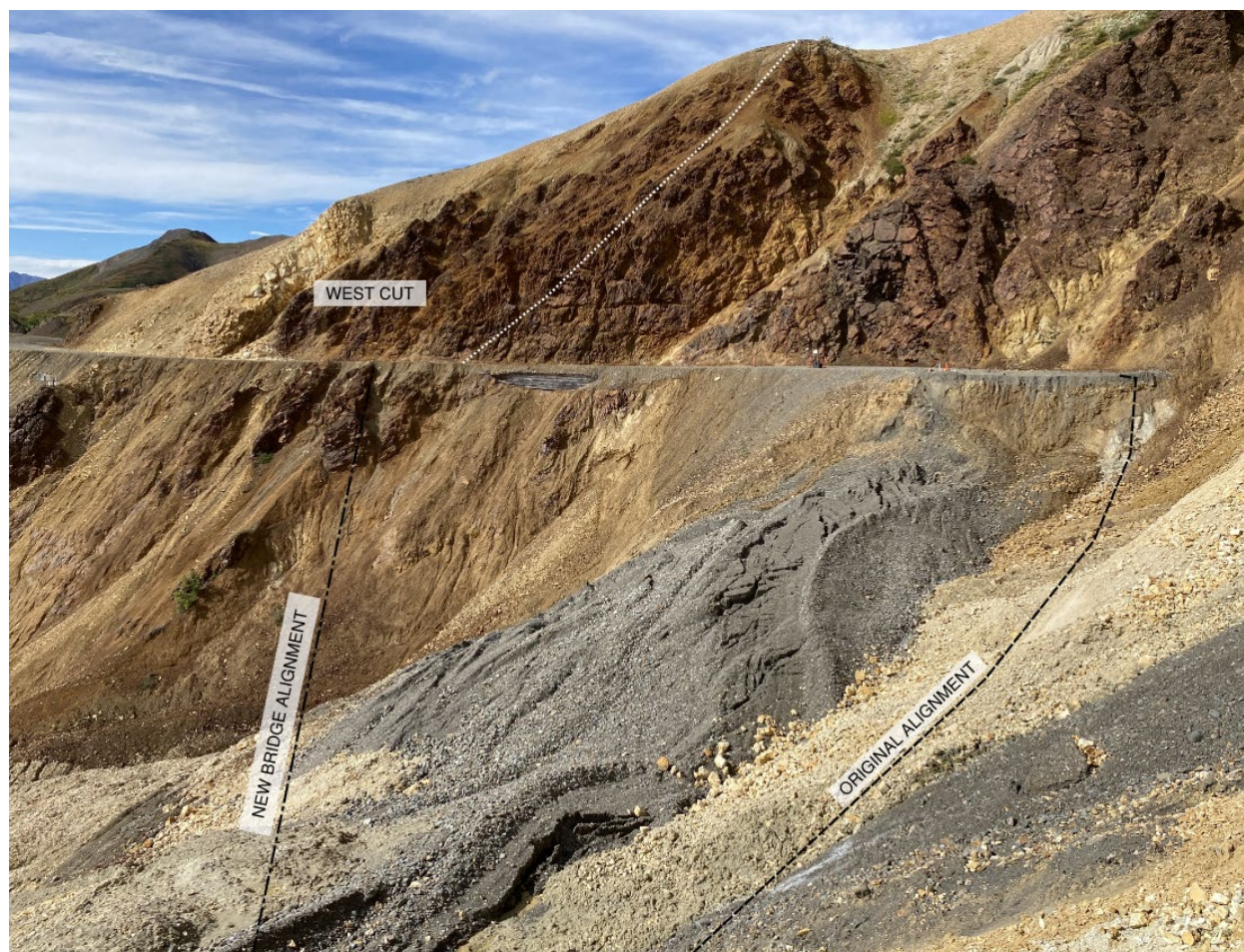
Figure 2 - Pre-Construction Photograph of West Cut (August 20, 2022) Looking from Approximately Abutment 1 Location towards Abutment 2 and West Cut.
