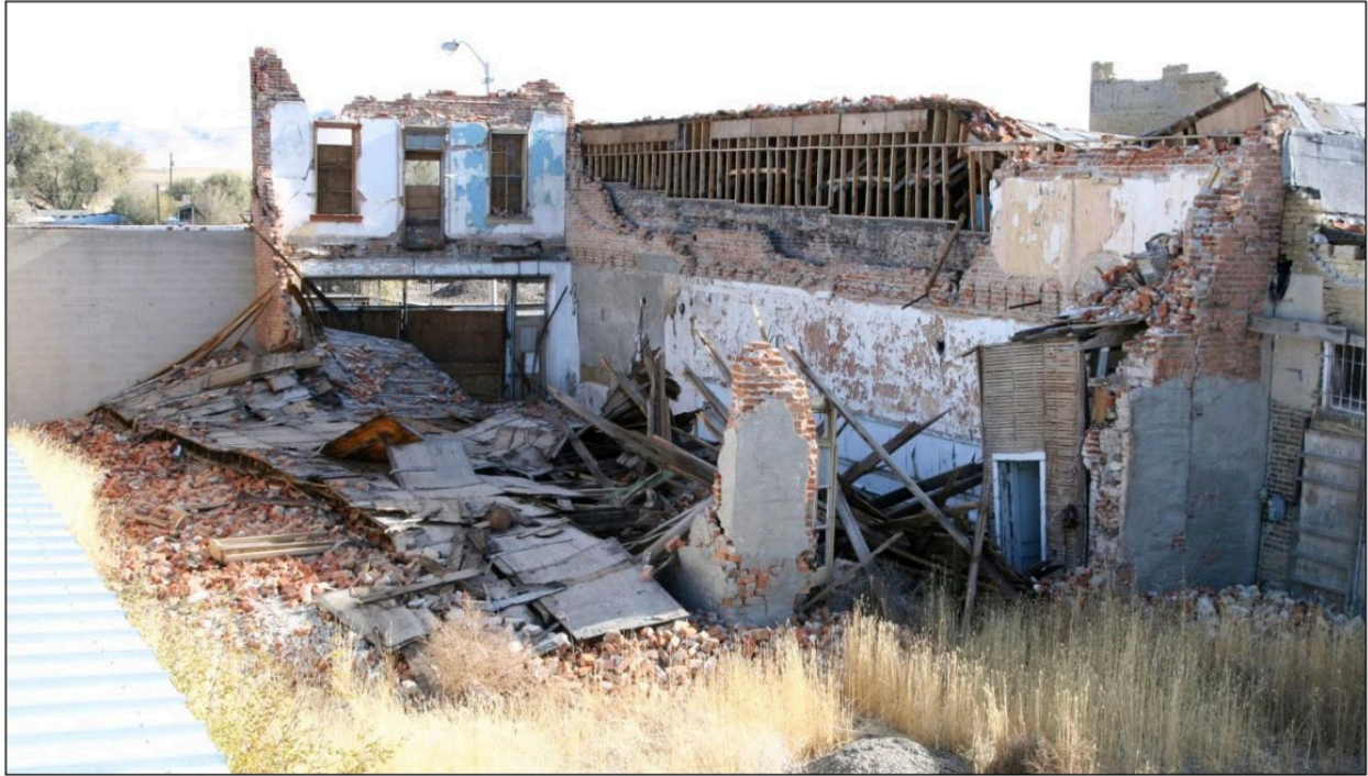
Figure 3. Unreinforced masonry building that collapsed during the magnitude 6.0 earthquake in Wells, Nevada on 21 February 2008, photo by C. dePolo (1).
