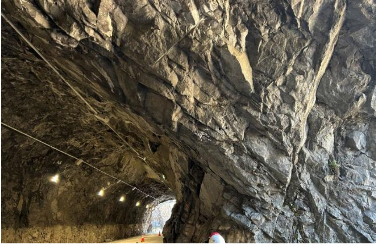
Figure 2. View of exposed rock within the Elephant Butte Tunnel
