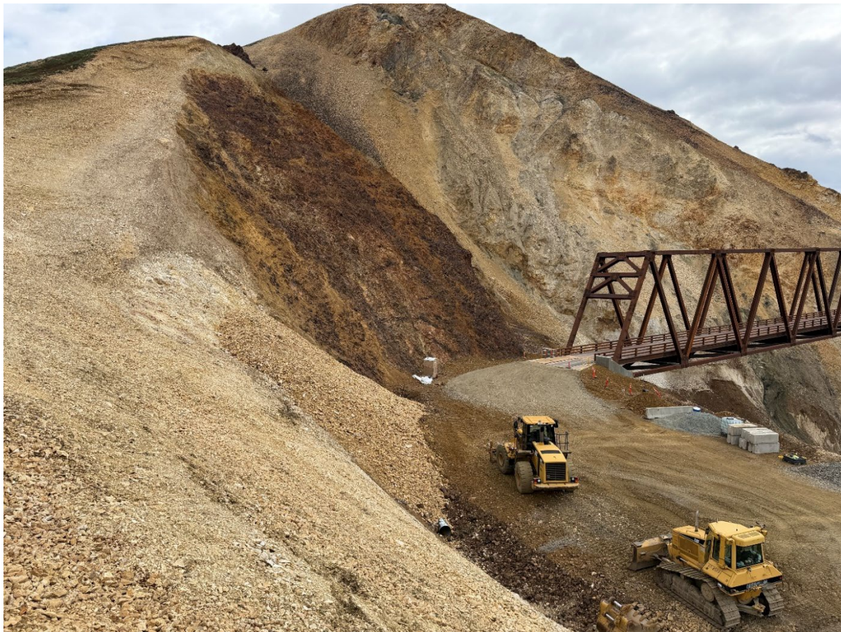
Figure 13 - Photograph of Completed West Cut (June 16, 2026).
