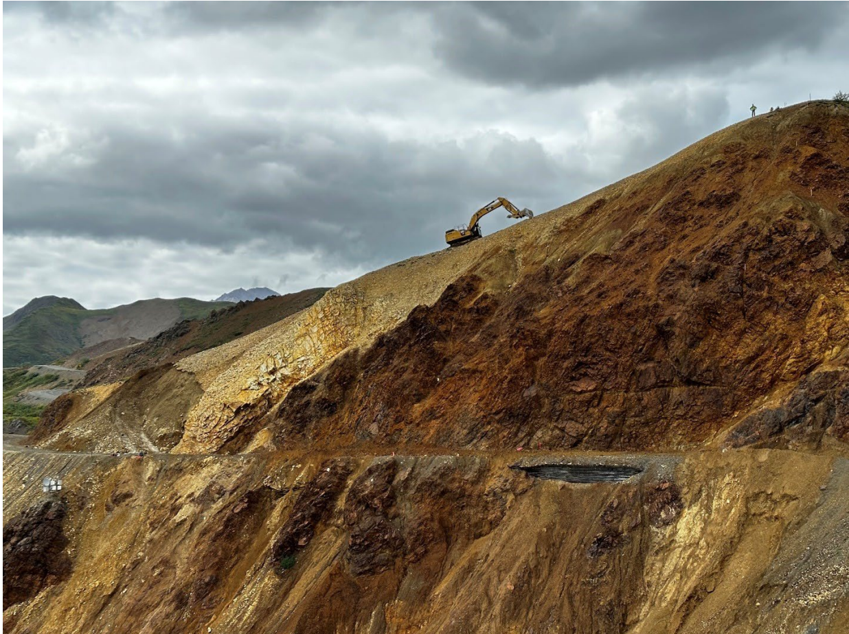
Figure 9 - Photograph of the Pioneer Access to the Top of the West Cut (August 23, 2023).
