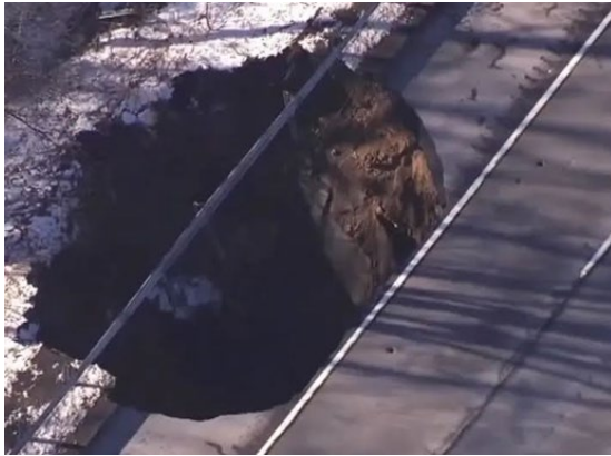
Photo of Mine Subsidence Location 1
