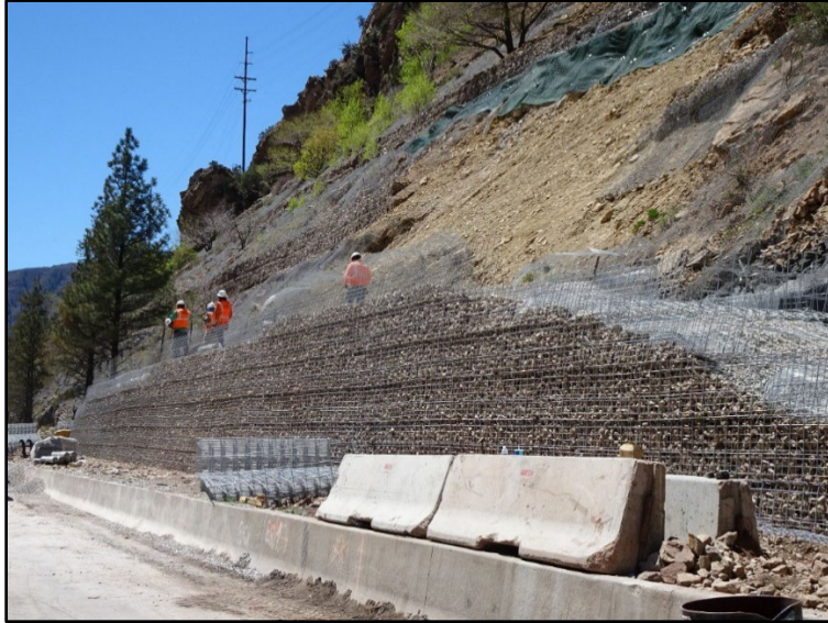
Figure 7 – I -70 near Glenwood Springs, CO. Construction of the double-sided wire vertical faced rockfall containment wall. Soil nail wall is located behind and out of view.
