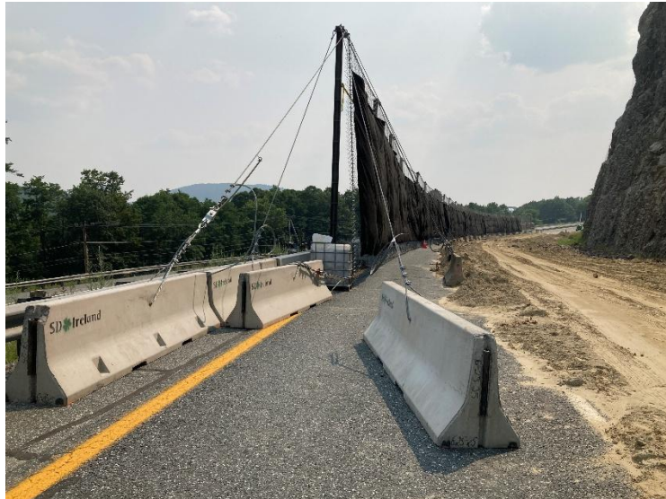
Figure 7 - Temporary rock fall barrier arrangement and sand cushion (Scarptec, 2025)
