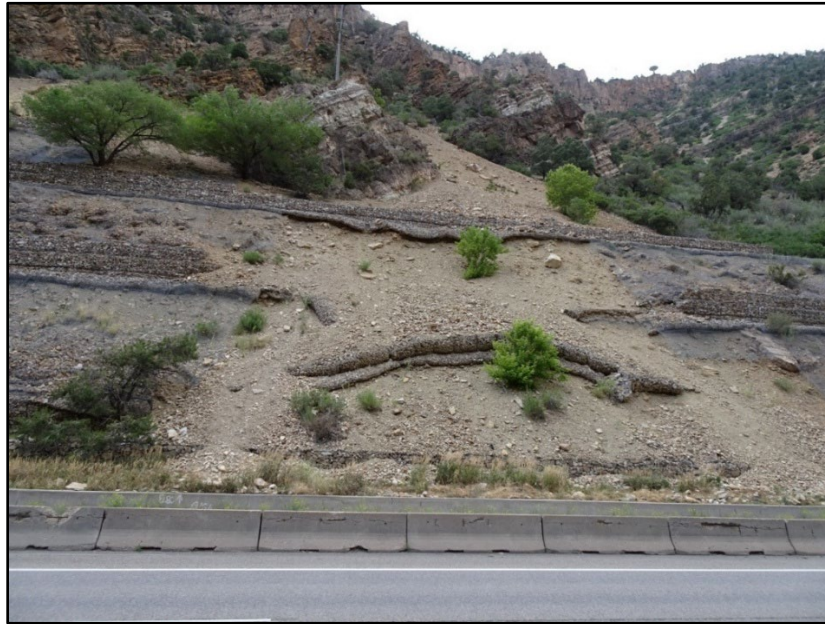
Figure 3 – I -70 near Glenwood Springs, CO with tiered gabion system to stabilize the cut slope.
