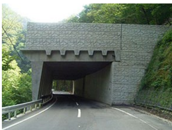
Figure 4 - Example of a Prestressed Concrete (PC) Rock Shed
