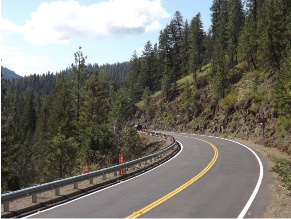
Figure 8 – Completed Repair and Reopened Roadway, Looking Southward
