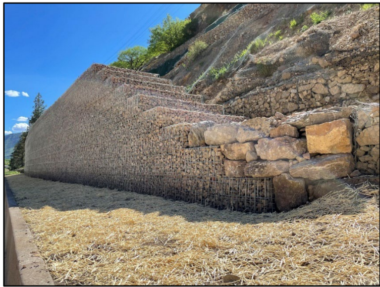
Figure 8 – I -70 near Glenwood Springs, CO. Final construction of the double-sided wire vertical faced rockfall containment wall.
