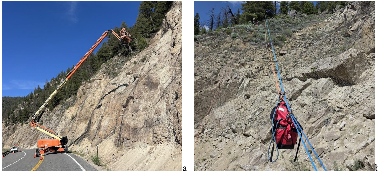
Figure 9 – Boom Lift Proving Insufficient (a) and Rope Haul System Implementation with a 130 lb. Battery (b)
