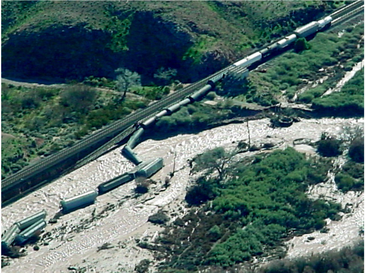
Figure 14. Flood in Meadow Valley Wash, Clark County, January 2005 (photo courtesy of Gale Fraser, Clark County Regional Flood Control District).
