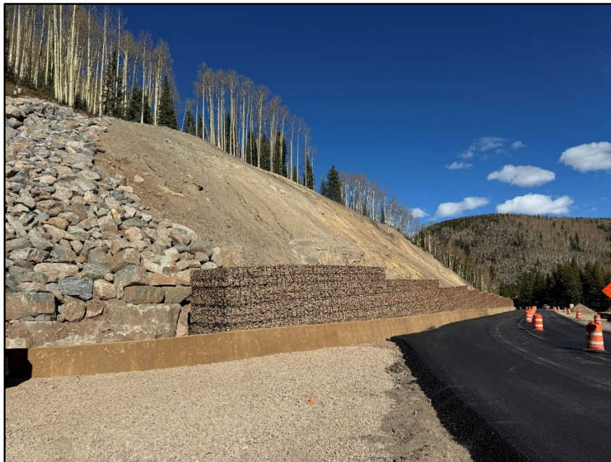
Figure 18. US 550 completed rockfall containment system.
