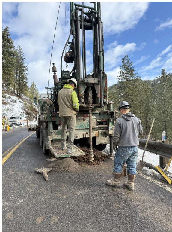
Figure 4 – Hollow-Stem Auger Drilling During the Field Investigation
