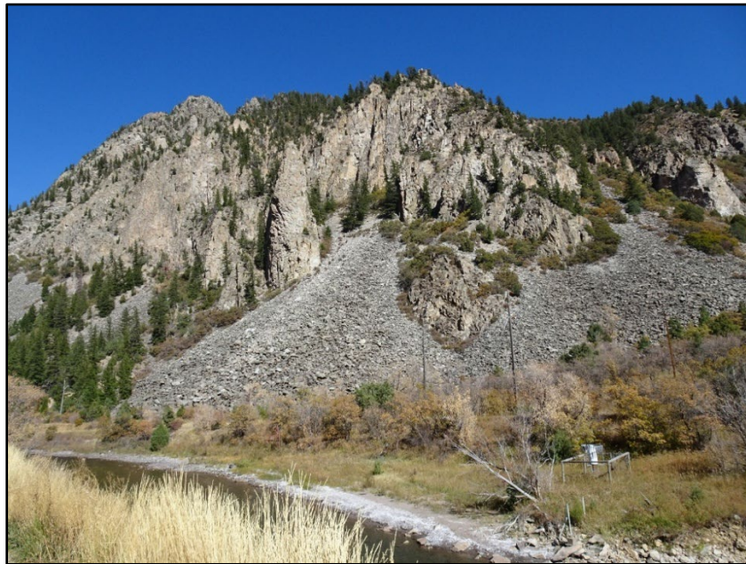
Figure 11 - CO 133 is an example of a talus slope that was located across the river valley that was in a natural slope condition at the angle of repose.
