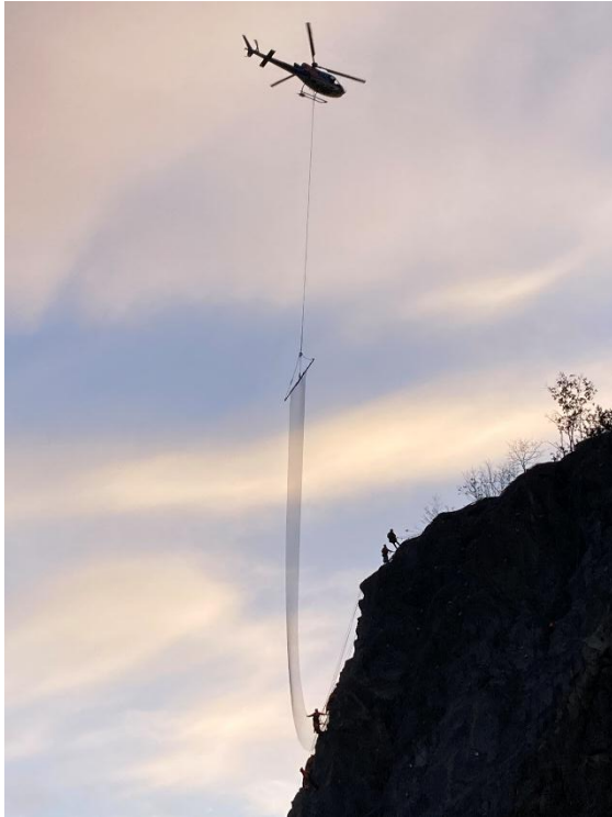
Figure 10 - Pinned mesh installation using helicopter (Scarptec 2025)
