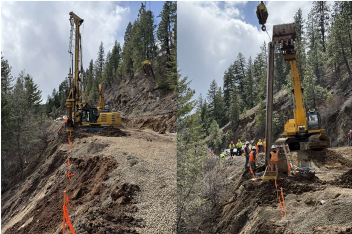
Figure 7 – Pile Installation
