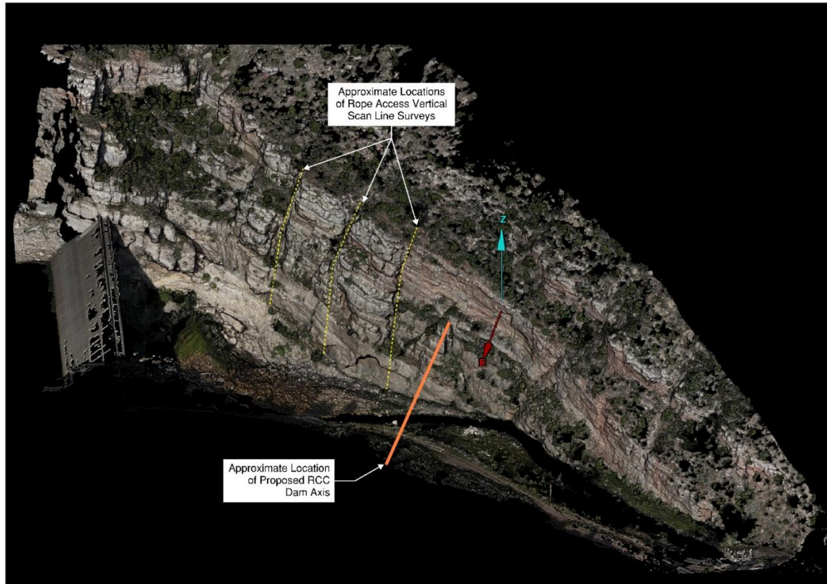
Figure 8. LaPrele Dam Left Abutment Rock-Wall Scan and Rope-Access Scanline Locations (6)
