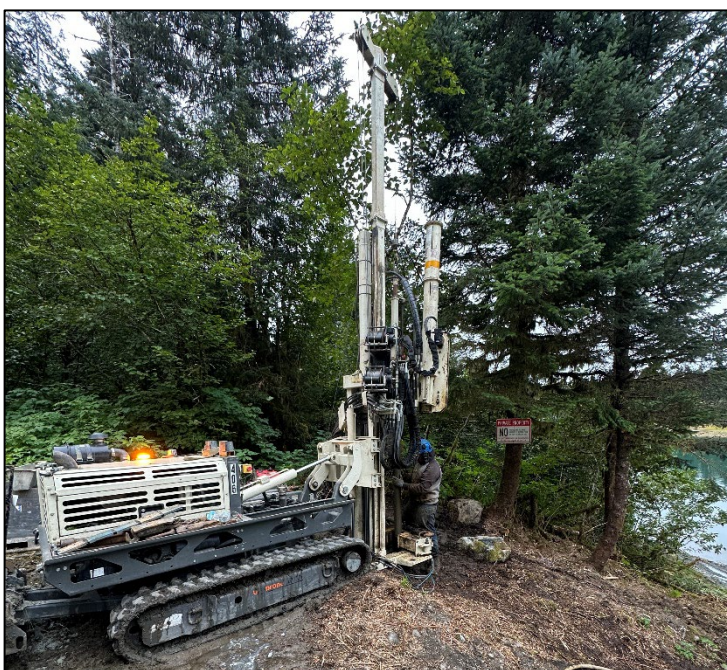
Figure 4: Drill rig advancing a boring at the north abutment
