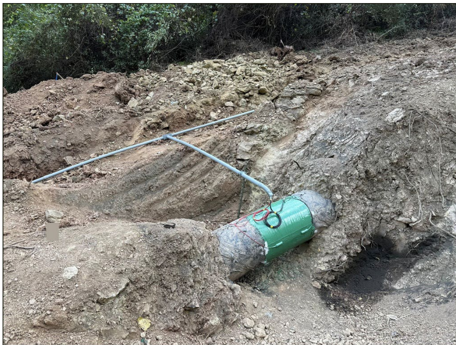
Figure 4: Excavated section of pipeline for the purpose of installing strain gauges.
