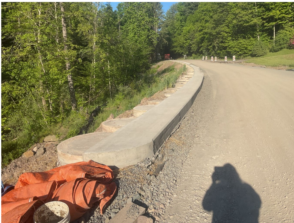
Photo 6: Completed Tangent Caisson Wall at Site 2
