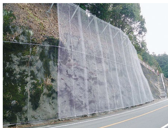
Figure 2 - Standard-Type Rockfall net
