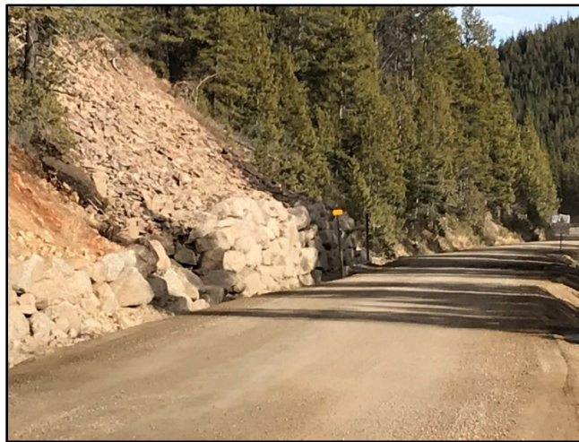
Figure 2 – Talus Slopes in Colorado where a small rockery wall is stabilizing the natural slope.
