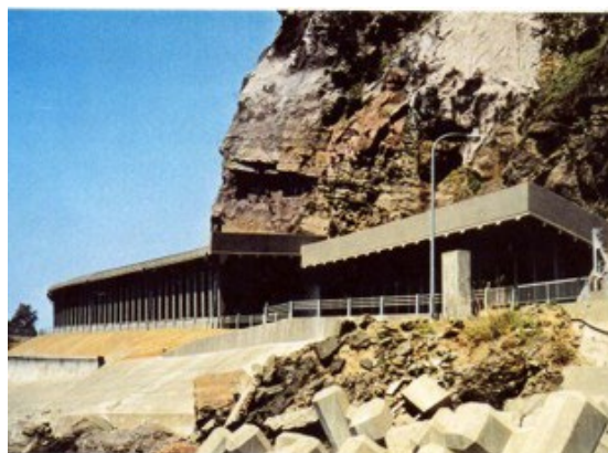
(a) Before the rockfall
