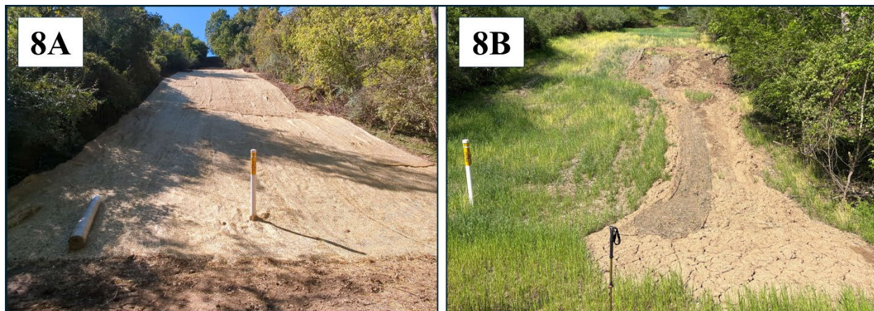
Figure 8A: Photo looking upslope at the recently regraded ROW located within the landslide complex. The slope was regraded after installation of strain gauges in 2025. Figure 8B: Looking upslope at the debris flow, which occurred after the slope regrading of Figure 8A.
