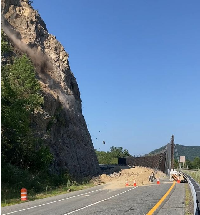
Figure 8 - Hand scaling operations (Scarptec 2025)
