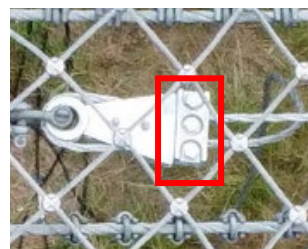
Figure 8 - Friction-Slip Energy Dissipation Device
