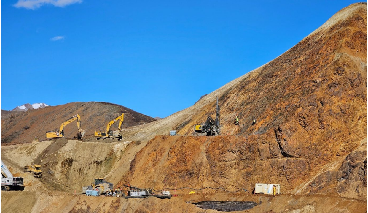
Figure 10 - Photograph of West Cut Excavation (May 31, 2024).
