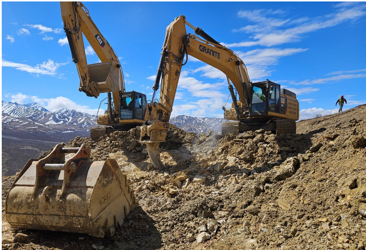
Figure 11 – Photograph of Frozen Colluvium Excavation (May 30, 2024).
