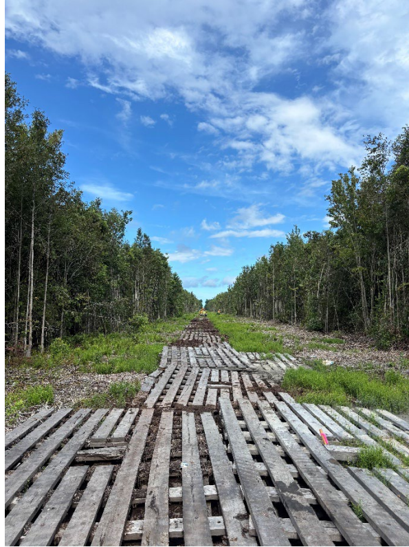
Fig. 7 – Timber mats to access the borings in Maple Swamp
