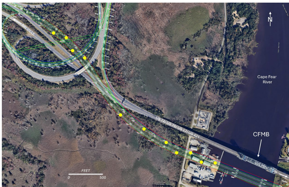
Fig. 9 – Map View Showing the MWD Boring Locations (Yellow Circle) on the West Side of the Cape Fear River. CFMB = Cape Fear Memorial Bridge.
