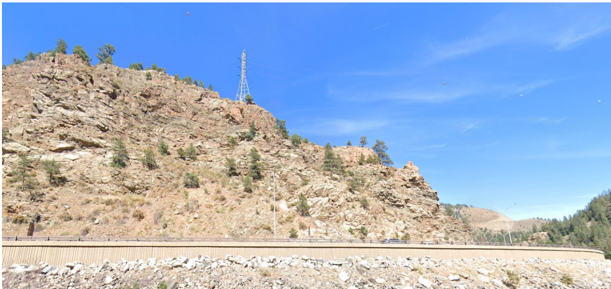
Figure 3 – Photo of the West Cut Showing the Curved Roadway, Flat Bench, Variable Jointing and Foliation, and Electrical Tower
