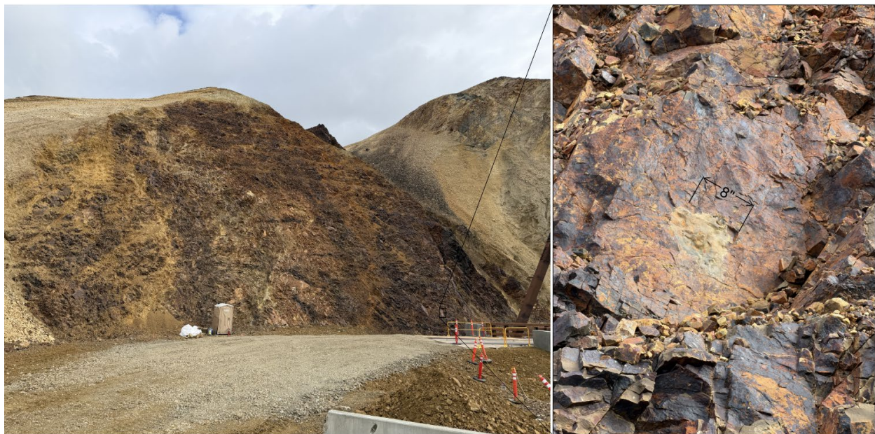
Figure 8 - Photograph of Completed West Cut and Close-Up of a Completed Rock Bolt Location (June 16, 2026).
