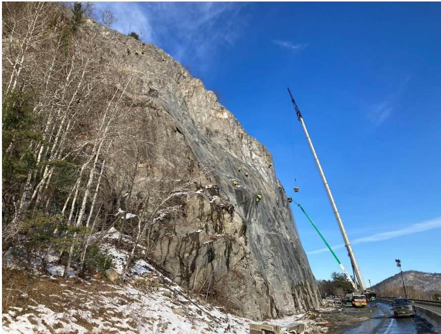
Figure 11 - Installation of draped mesh using a crane and telehandlers (Scarptec 2025)
