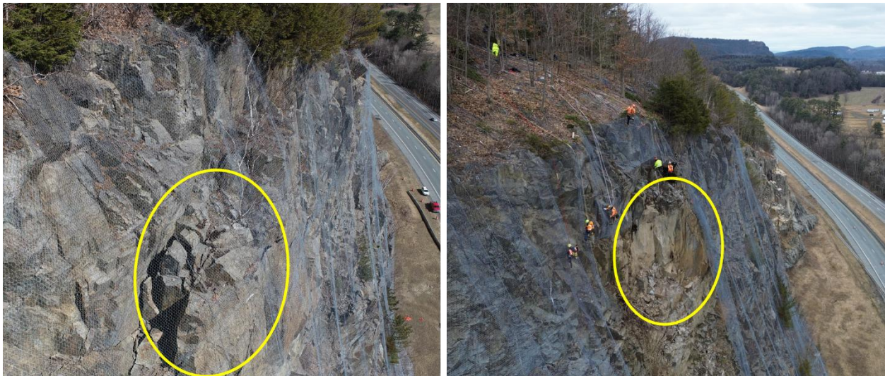
Figure 5 – Drone images of rock fall source area prior to rock fall (left) on April 5, 2022, and scar following rock fall (right) March 5, 2024 (VTrans)
