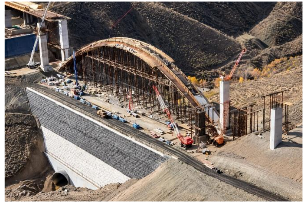
Figure 16. Photo from Durski (ASPIRE The Concrete Bridge Magazine, Winter 2010) of the partly completed arch forms with the MSE/RSS walls in place during construction. (NDOT)
