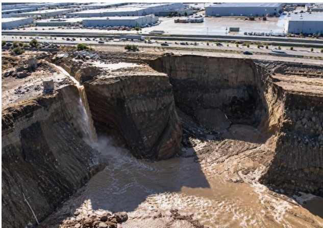
Figure 7. (left) Closer view of the eroded pit wall at the moment of breach. (right) Sparks Marina in Google Satellite View.
