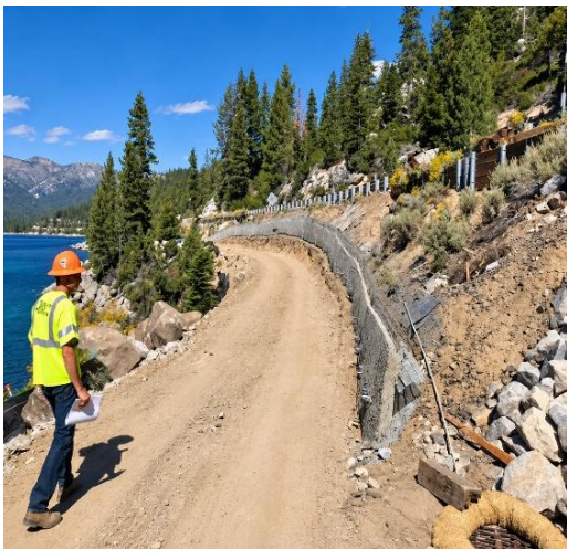
Figure 31. A soil nail wall holds the active highway alignment above the new trail bed.
