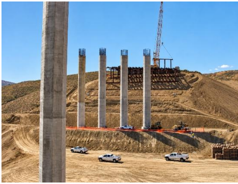
Figure 13. Bridge piers and falsework framing under construction, prior to placement of the arch spans. (NDOT)
