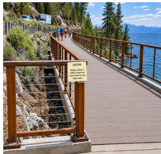
Figure 32. The finished trail: a cantilevered steel-surfaced boardwalk carries walkers and cyclists along the cliff face above Lake Tahoe's east shore.
