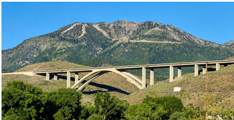
Figure 10. View of the Galena Creek Bridge on I-580 from Pleasant Valley below. Mt. Rose in the background.
