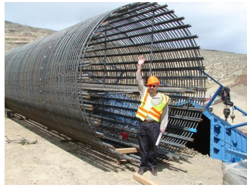
Figure 14. Bridge pier reinforcement cage. (NDOT)
