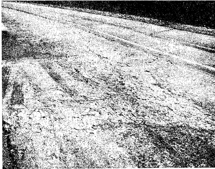
Fig. 1. Failure of concrete pavement which began after 14 years of service under moderate traffic.
