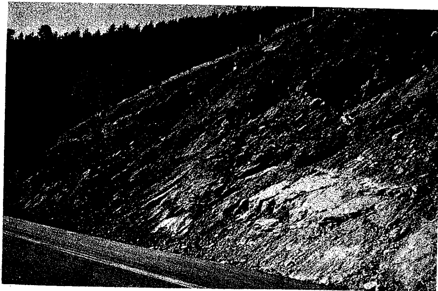
Plate 12. Upturned sedimentary rocks west of Dayton, Wyoming. Example of a bedding plane rock slide.
