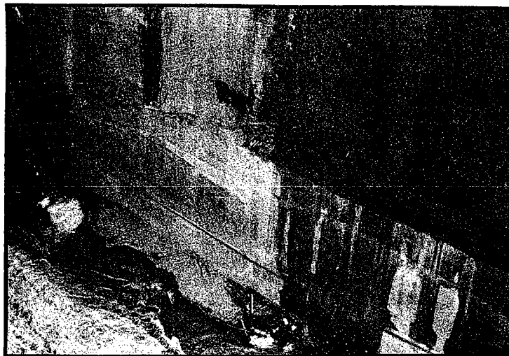
Figure 40 The Completed Concrete Filling Of The Undermined Tunnel Section
