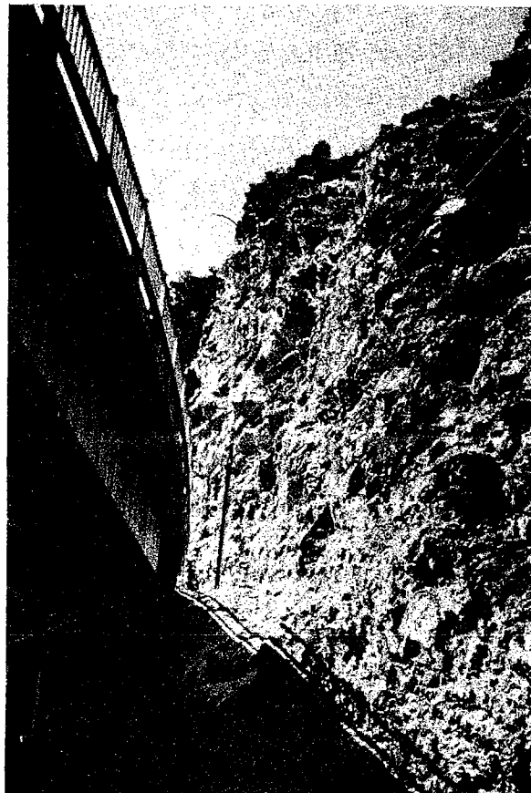
Plate 16. Rock cut east of Idaho Springs, Colorado, on opposite side of canyon from Plate 15, showing up-dip side of the same rock formation. This slope is nearly vertical whereas slope in Plate 15 is following the foliation plane.
