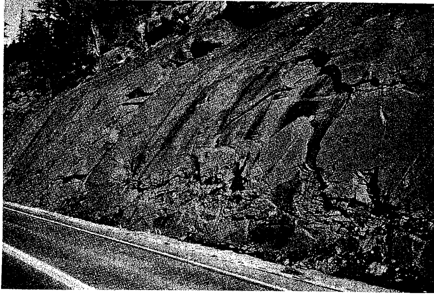
Plate 22. Example of a sandstone being over-shot during cut excavation. Over-shooting may create residual stress zones in the rock which could cause spalling as these stresses are relieved.
