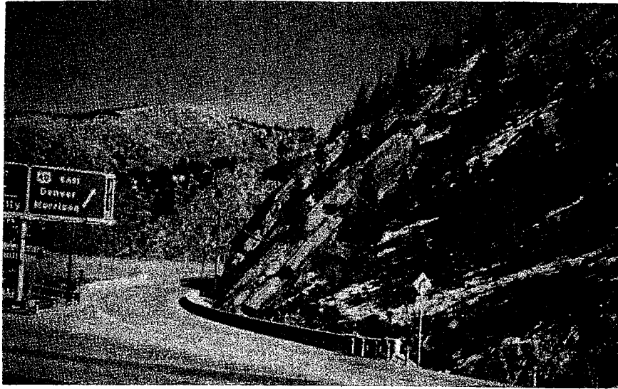
Plate 15. Rock cut east of Idaho Springs, Colorado. Showing rock-slide area as described in Plate 11. Road is on down-dip side of the foliation planes in the rock.
