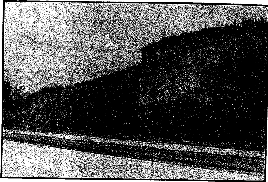
Figure 47 Backslope In Loess-Like Material And Sand On I-70 West Of Kansas City
