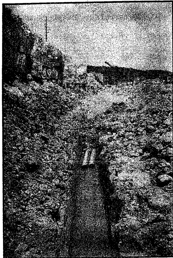
Figure 12 Right The Installation Of An Underdrain At The Bottom Of The Cut Section Shown in Figure 11
