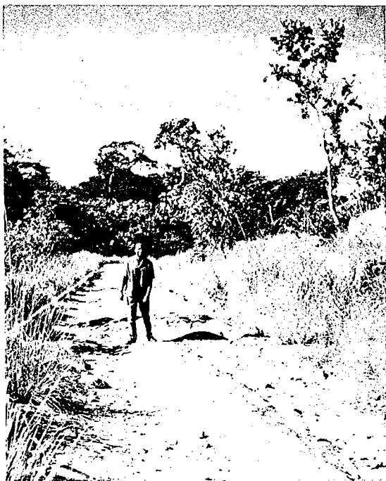
Figure 5. A section of road developed in weathered clayey and bouldery soil of the Crystalline rocks.
