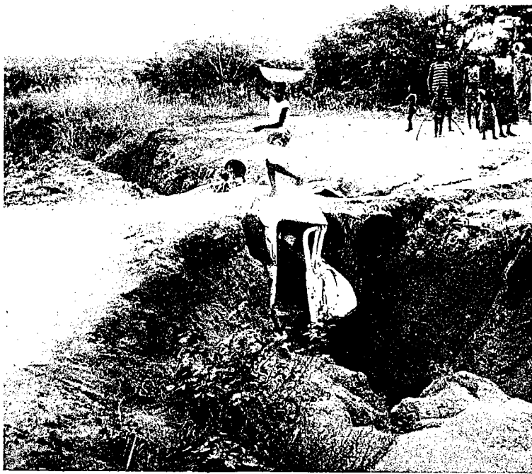
Figure 10. Examples of side-drain erosion: A, near Bakwa-Mpuka on northern alignment; B, on the Sandstone and Siltstone unit of another section on the northern alignment; and C, truck-body culvert in badly eroded side drain on southern alignment.
