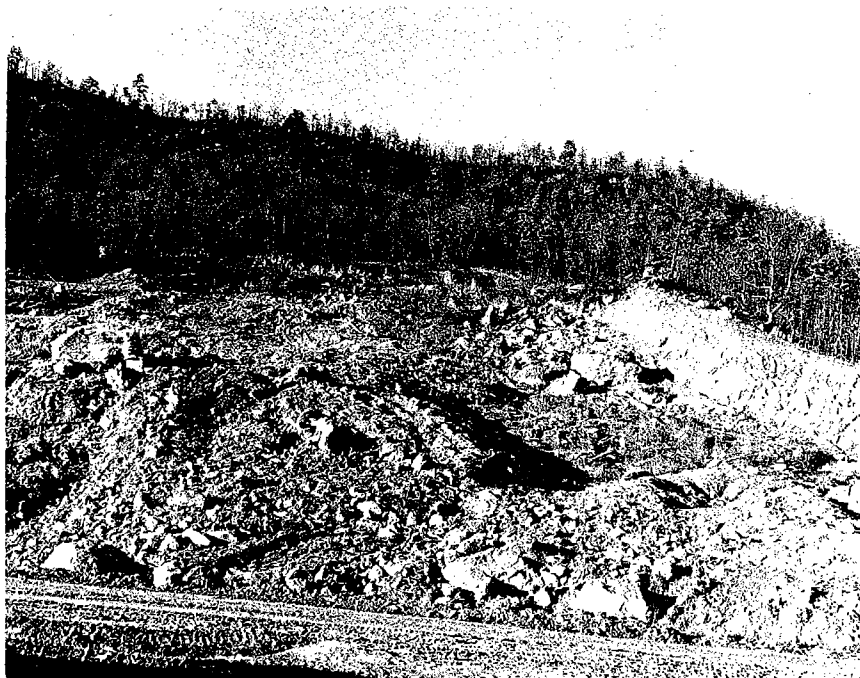
FIGURE 5. MASSIVE COLLUVIAL CUT SLIDE ALONG INTERSTATE -40 NEAR ROCKWOOD IN ROANE COUNTY.
