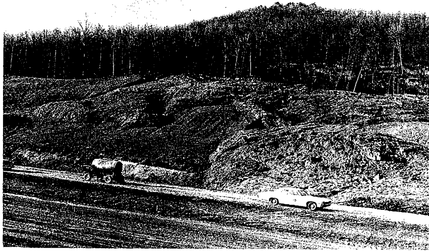
FIGURE 4. COLLUVIAL SLIDE ALONG I-40 NEAR CRAB ORCHARD IN CUMBERLAND COUNTY.
