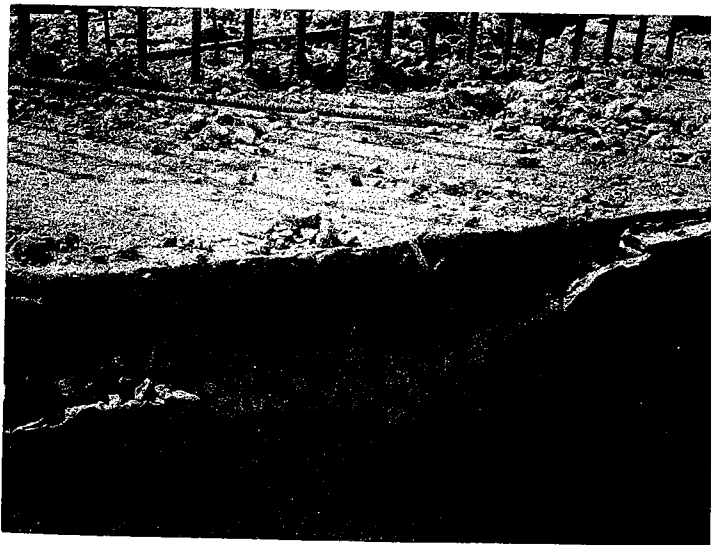
Fig. 9 View of retaining wall foundation before removal showing distress cracks. Scale is indicated by pocket knife.
