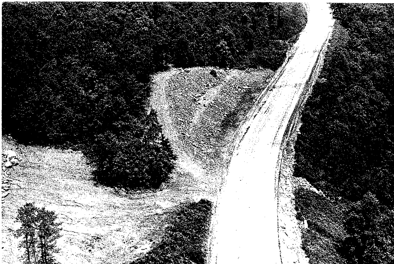
FIGURE 9. BUTTRESS BEING USED TO CONTROL SLIDE ALONG THE EAST-BOUND LANE OF I-40 AT ROCKWOOD.
