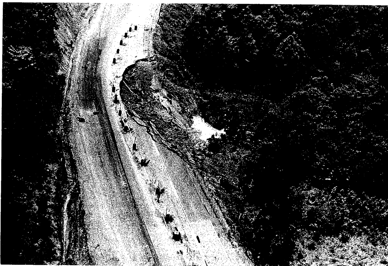
FIGURE 6. EMBANKMENT FAILURE ALONG STATE ROUTE 30 JUST EAST OF DAYTON IN RHEA COUNTY.
