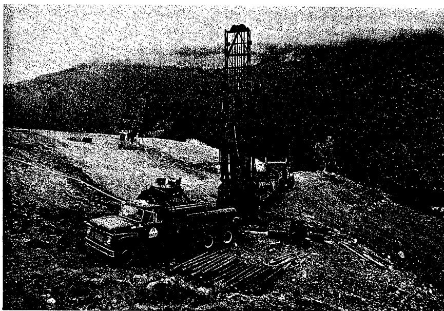
Fig. 8. Becker Hammer Drill set up on the drainage well site. Cyclone separator is partially visible behind pipe truck.
