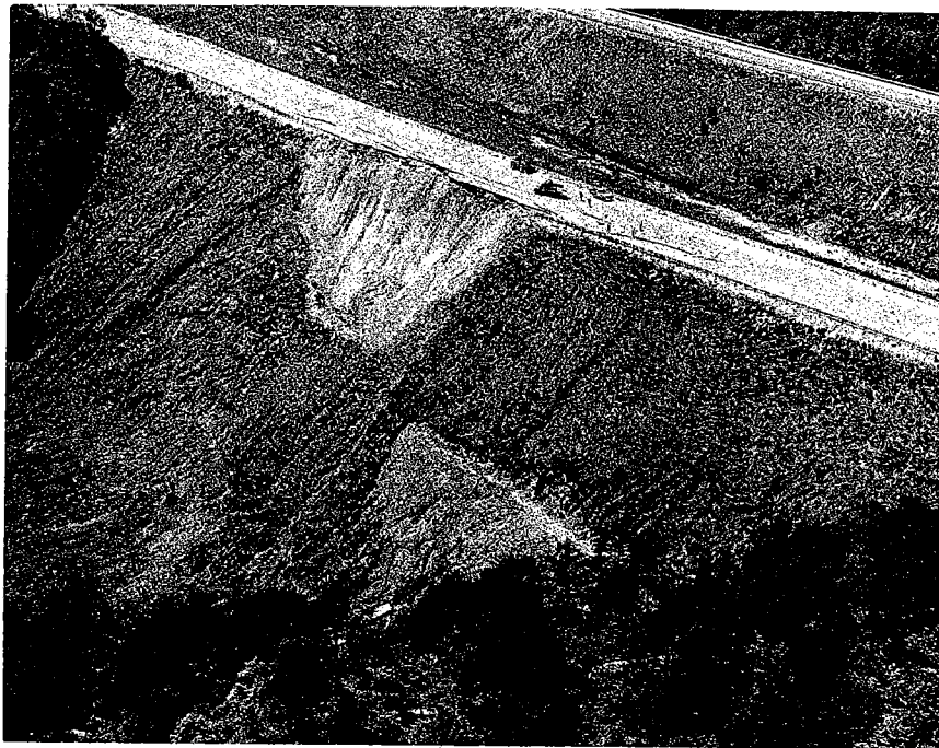
FIGURE 15. AERIAL VIEW OF AN EMBANKMENT FAILURE THAT OCCURRED ALONG THE NORTH-BOUND LANE OF I-75 IN APRIL, 1972 .
