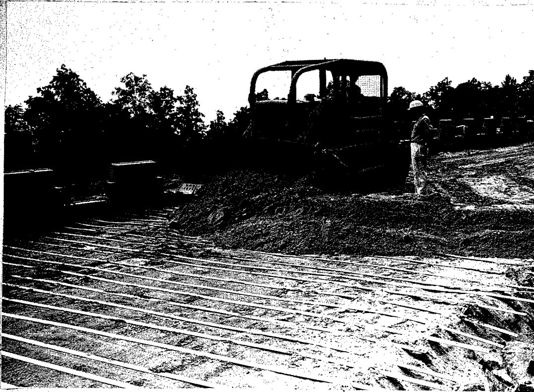
FIGURE 13. THE SAND IS SPREAD AND COMPACTED IN 8-INCH TO 10-INCH LAYERS.
