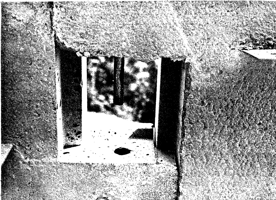
FIGURE 10. CLOSE-UP OF THE INTERLOCKING FEATURES OF THE PANELS.
