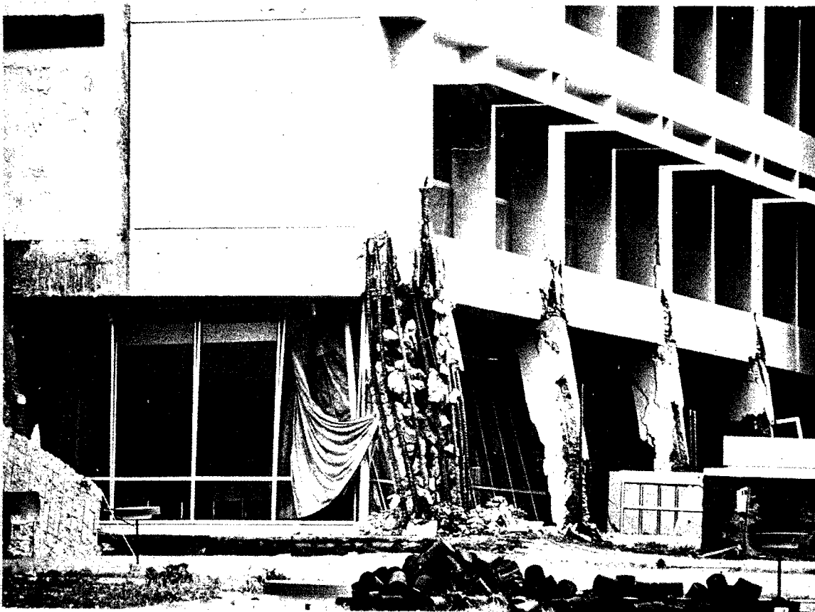
Fig. 9 Damaged columns in New Olive View Hospital caused by San Fernando Earthquake of 1971 (Photo by author).
