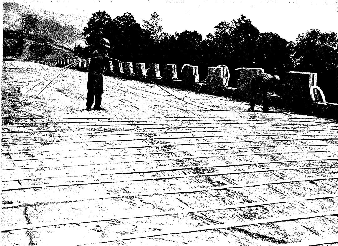
FIGURE 12. THE REINFORCING STRIPS ARE 1' TO 3' APART HORIZONTALLY AND 1\frac{1}{2} ' TO 3' VERTICALLY.
