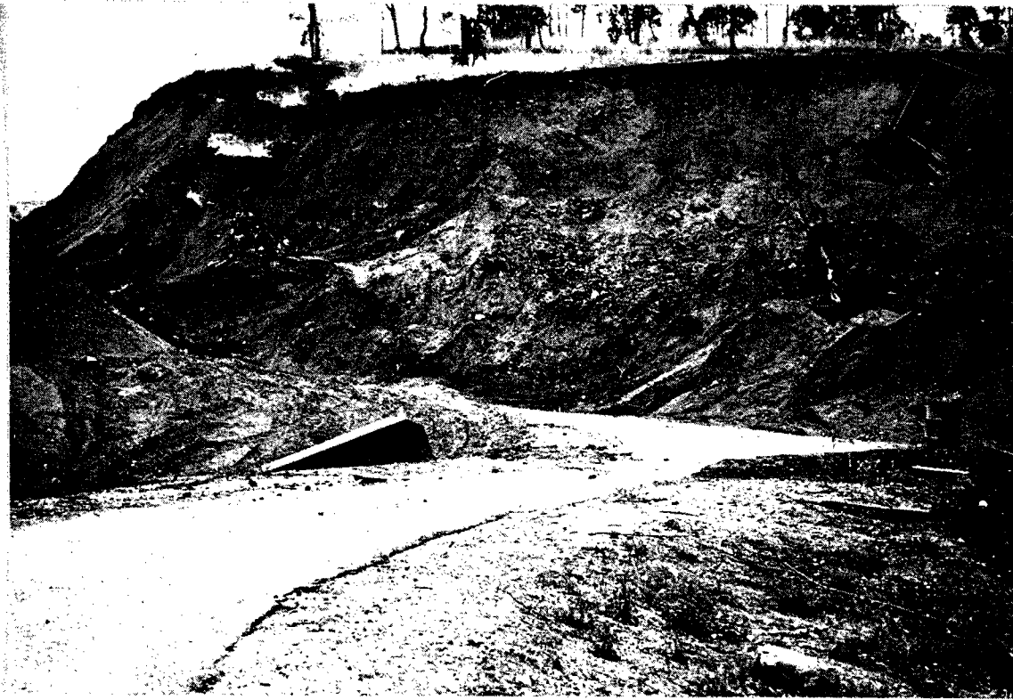
Fig. 10a Earthquake-triggered land slide blocking road following San Fernando Earthquake of 1971 (By author).
