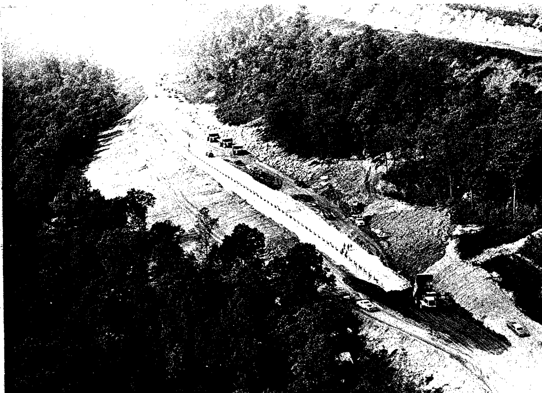
FIGURE 18. THE OUTER TRENCH SLOPE WAS FILLED IN AGAINST THE BASE OF THE WALL ON A 5:1 SLOPE RATIO.
