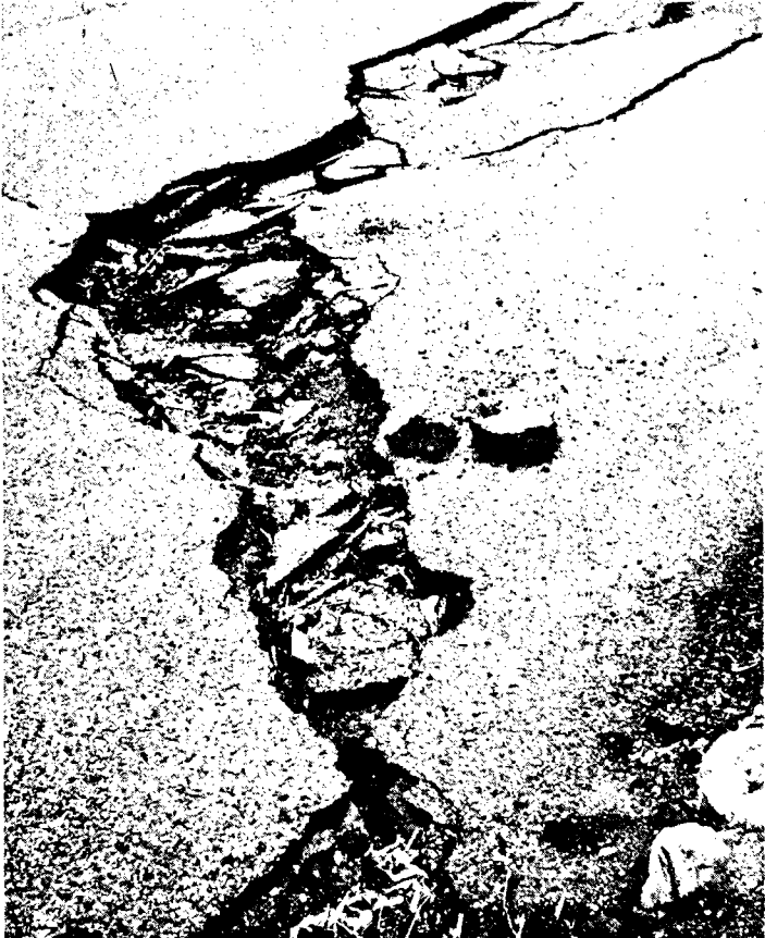
Fig. 10 b Pavement cracked by San Fernando Quake of 1971 (by author)
