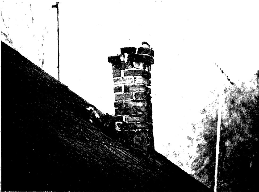
Fig. 13b Old chimney in Newry S. C. (7 m E. of epicenter) that broke from disrepair months before the earthquake and remained unchanged during the earthquake.
