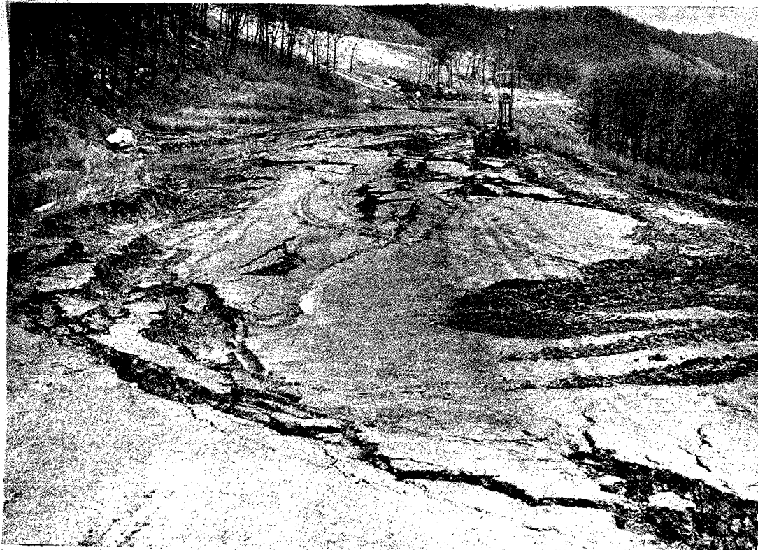
FIGURE 1. GROUND VIEW OF SLIDE CENTERED AT STATION 2038+00 OF THE EAST-BOUND LANE.
