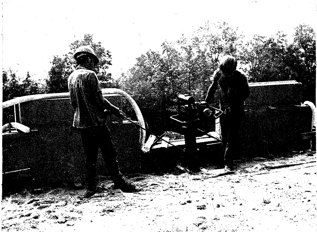
FIGURE 16. COMPACTION NEAR THE WALL WAS ACHIEVED WITH A GASOLINE POWERED HAND TAMPER.
