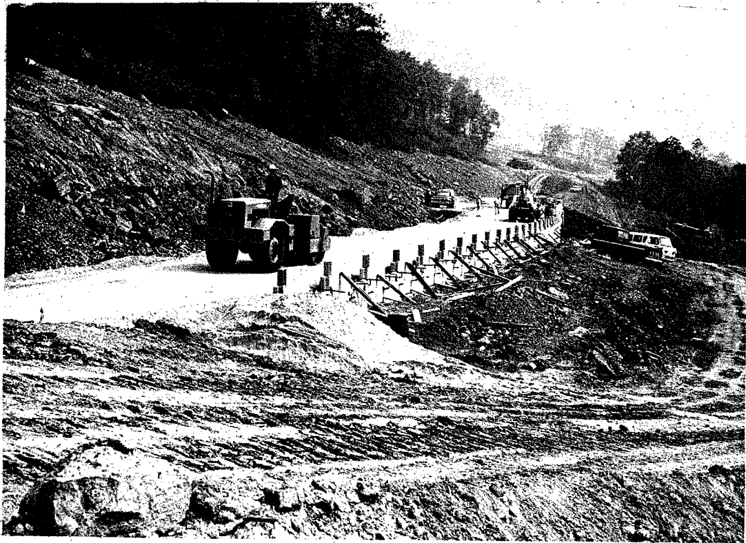
FIGURE 15. COMPACTION WAS ACCOMPLISHED WITH A VIBRATORY ROLLER TO AT LEAST 95% OF THE MAXIMUM LABORATORY DENSITY.
