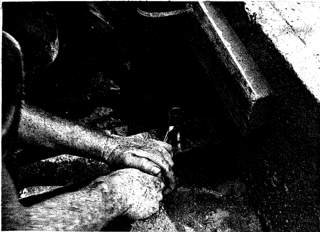
FIGURE 11. THE REINFORCING STRIPS ARE ATTACHED TO THE PANELS WITH TWO 1/2 " X 1" BOLTS.
