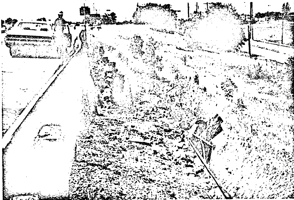
Figure 2. Wood pile and guard rail retaining structure.
