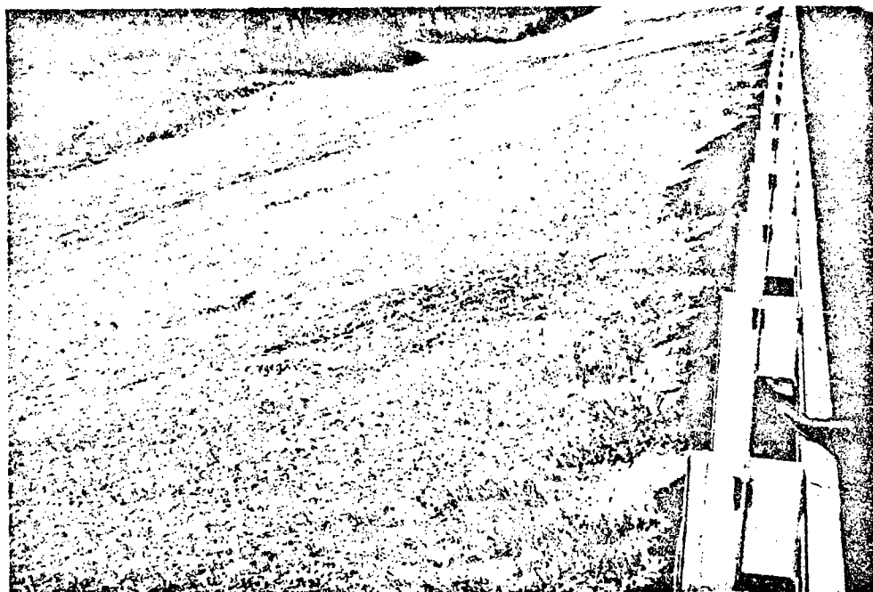
Figure 3. Addition of berms to flatten slopes.
