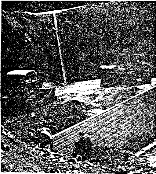
Photo 4. Erection of facing elements and backfill operations.
