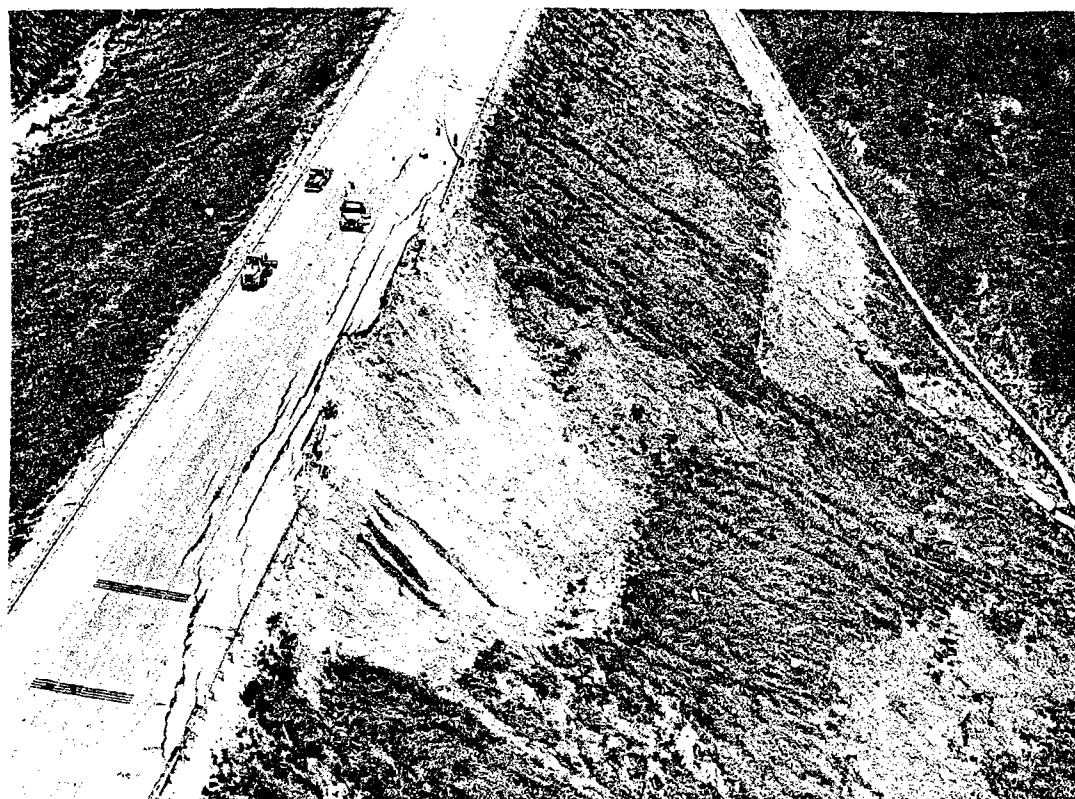
Figure 12. Aerial View of a massive Fill Failure along I-75 in Campbell County.
