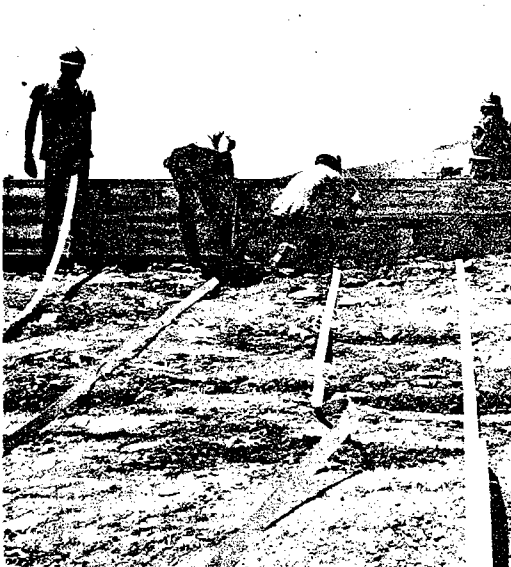
Photo 6. Attaching reinforcing elements to 13 inch face "skins".
