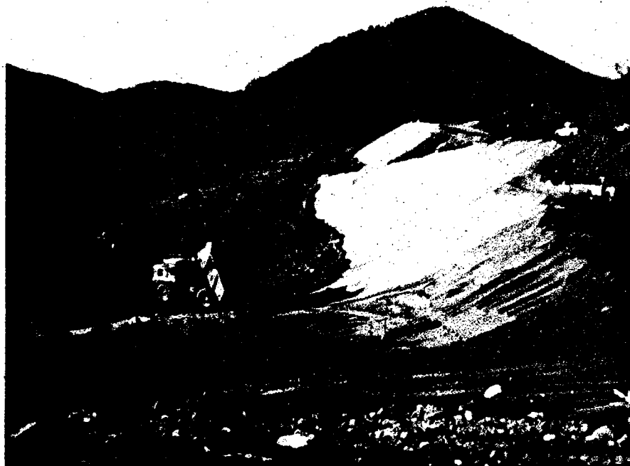
Figure 15. Embankment material being placed over sand and stone blanket. Lighter material is stone; the darker, sand.
