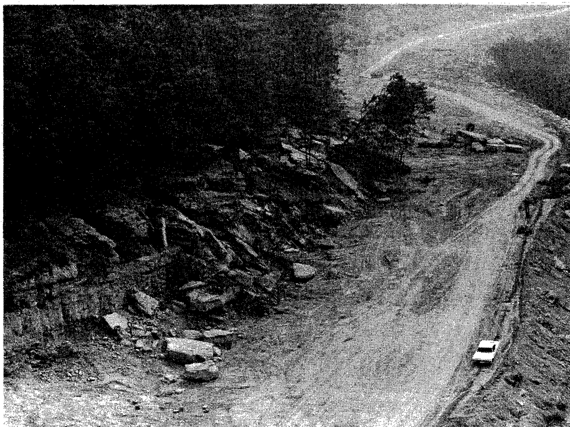
Figure 6. The strata in this cut which failed during construction are inclined approximately 22 degrees toward the roadway.
