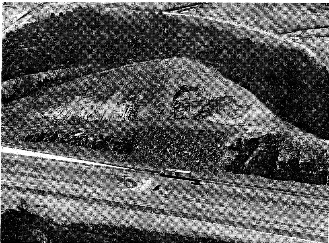
Figure 23. Removal and restraint with a rock buttress were the corrective measures utilized (see Figure 22).
