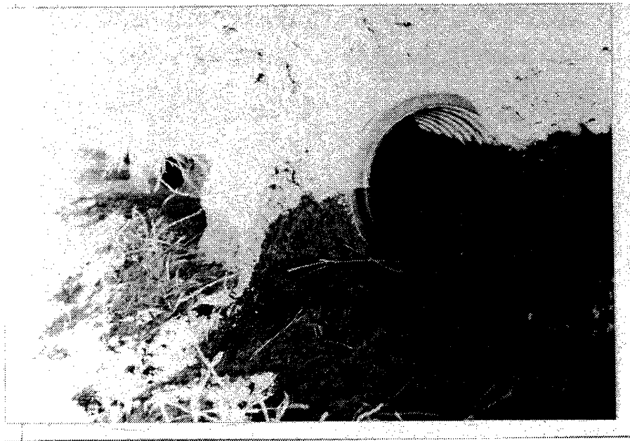
Figure 12. Corrugated polyethylene tubing is installed with a pit-run gravel envelope in a trench. This is a Case 2 installation.
