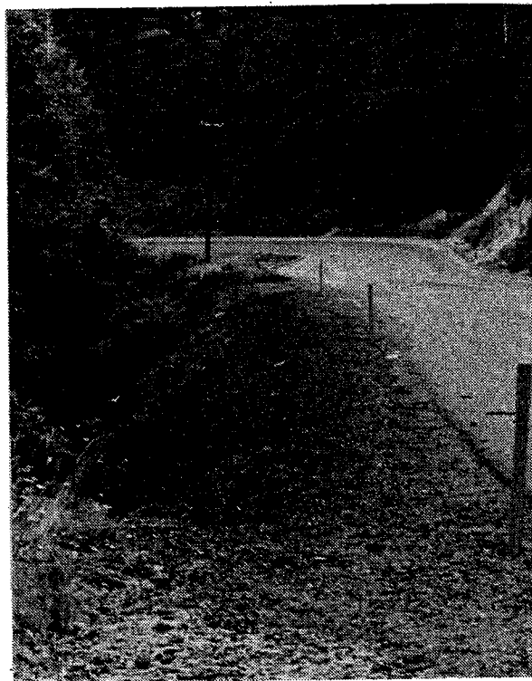
Figure 3 - Sawdust Fill - crack typical on fills with steep side slope
