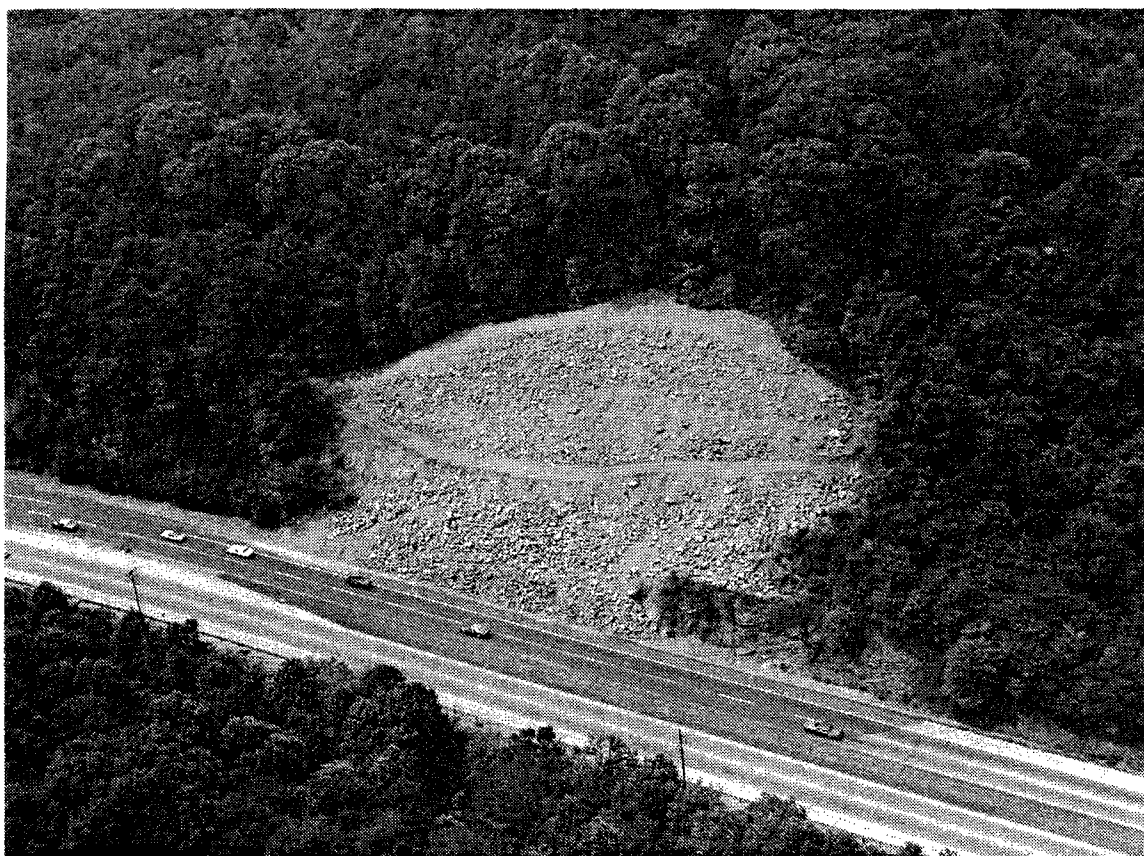
Figure 20. Partial removal and a revetment-like buttress were utilized in the repair of the mud flow shown in Figures 11 and 12.
