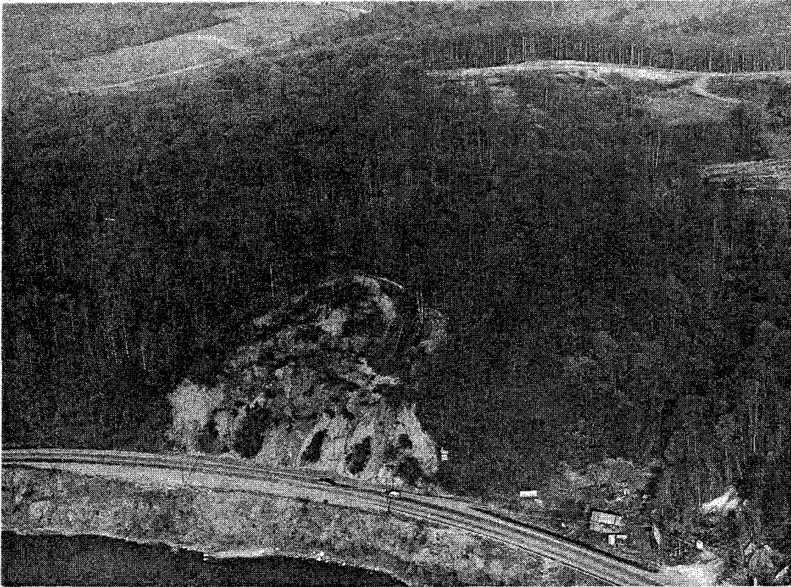
Figure 25. This failure, a translational-slump-flow, developed along relict bedding that dipped directly toward the roadway.
