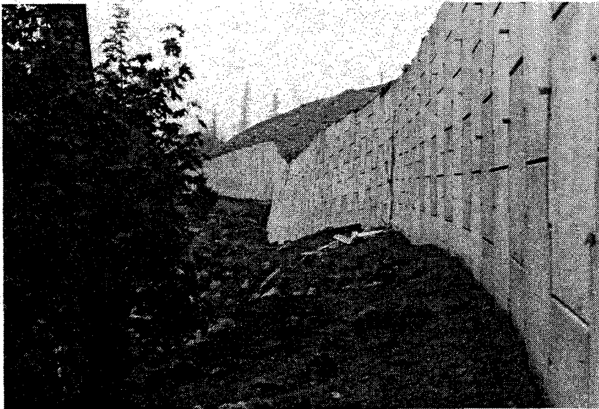
Photo 2 RE Wall Movement Caused by Landslide
