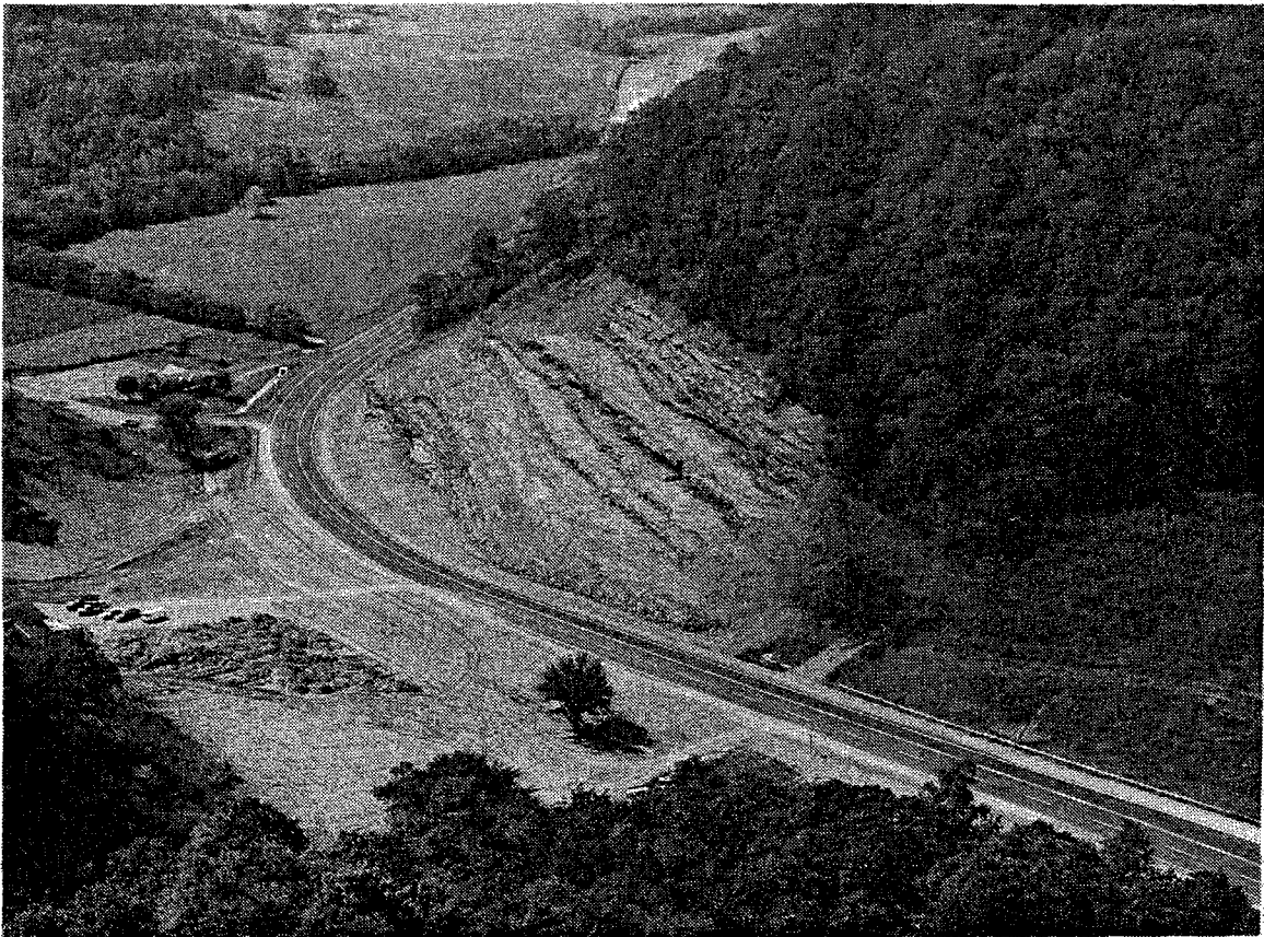
Figure 17. Total removal was the measure used to correct the mud flow shown in Figures 9 and 10.
