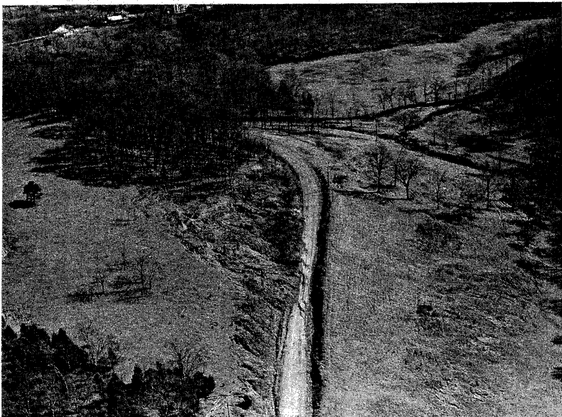
Figure 8. This failure began as a rotational slide but had deteriorated to a slump-flow by the time this photograph was taken.
