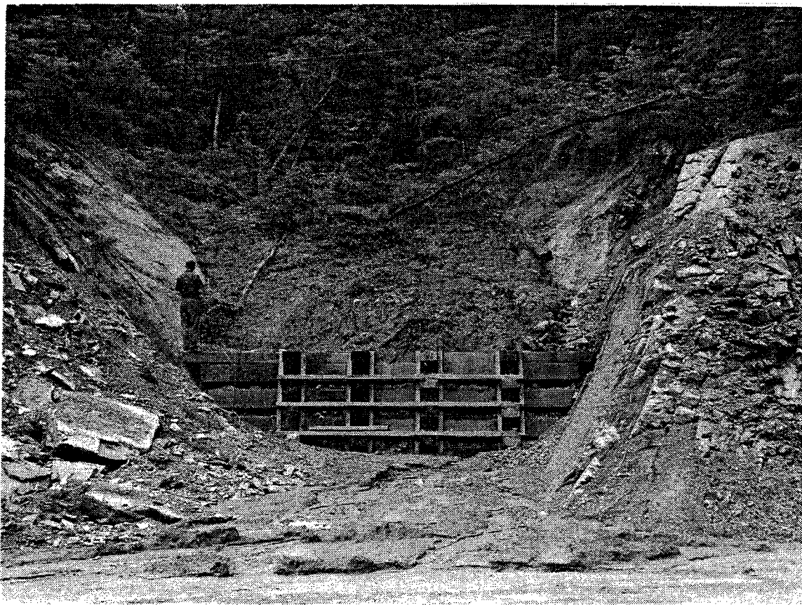
Figure 44. A small timber structure used to control a translational slide that developed in a plunging syncline along a rural road in Hamilton County.
