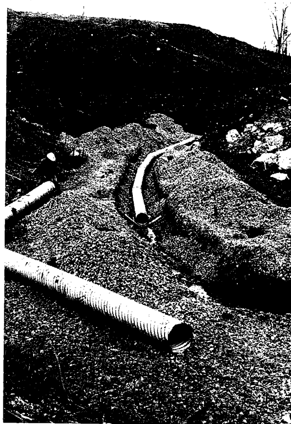
Figure 14. French drains reinforced with perforated underdrain pipe are used effectively to drain karst areas with numerous springs. Illustrated above is the installation of a French drain which will provide drainage for one of eleven springs located beneath a fill section of I-640 in Knox County.
