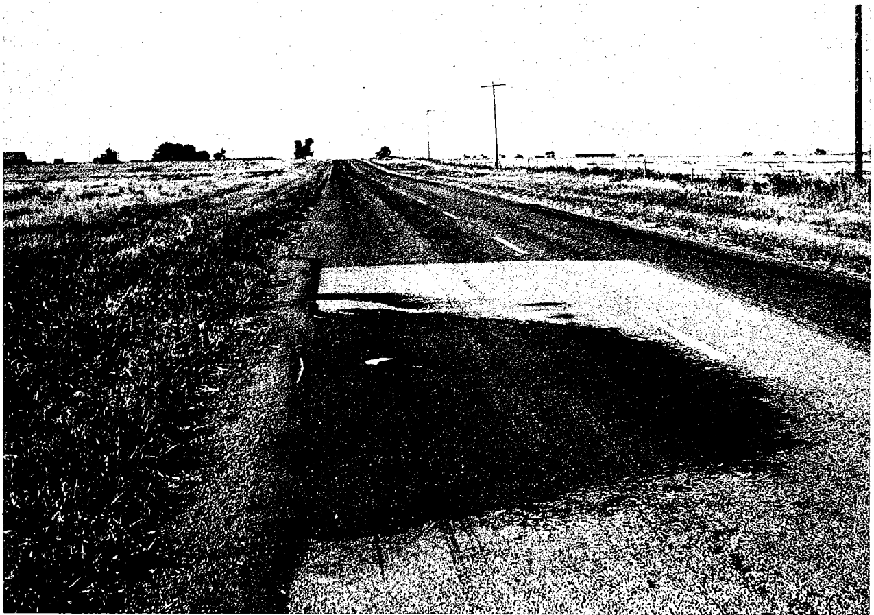
Figure 8. View south along FM 1033 in Childress County showing collapse depression. The depression affects most of the northbound lane and extends into the borrow ditch. Different shades of road patches at this site attest to the history of subsidence.
