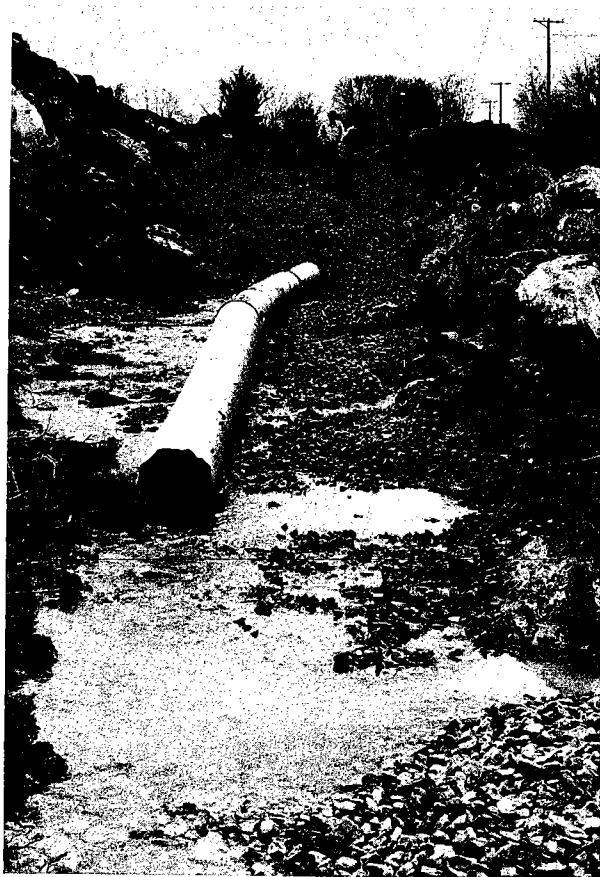
Figure 13. Perforated pipe reinforced French drains have been used with great success in draining springs along a part of I-640 in east Knox County.
