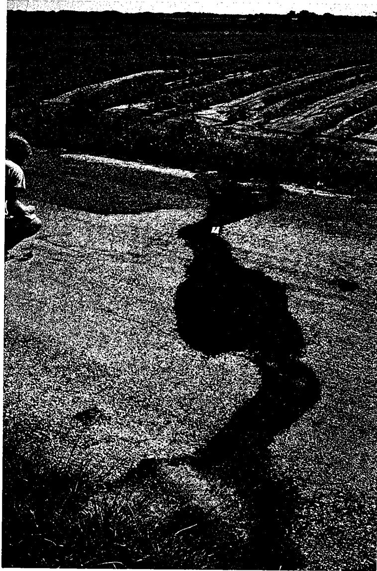
Figure 10. Fault trending northeast across FM 2639 in Hall County. Left side of fault is depressed approximately 3 to 4 cm (1.5 to 1.8 inches) relative to the right side. Fault extends into the cultivated field.
