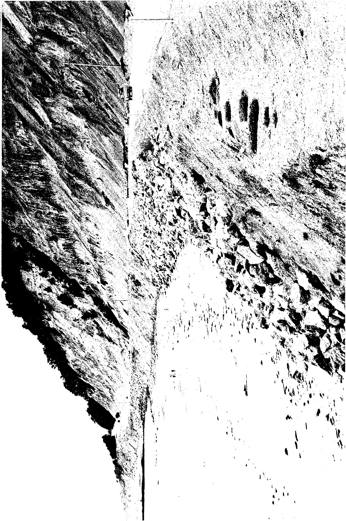
Figure 13. View upcoast of riprap emplaced in 1983 to save 1800 feet of Highway One from wave attack.
