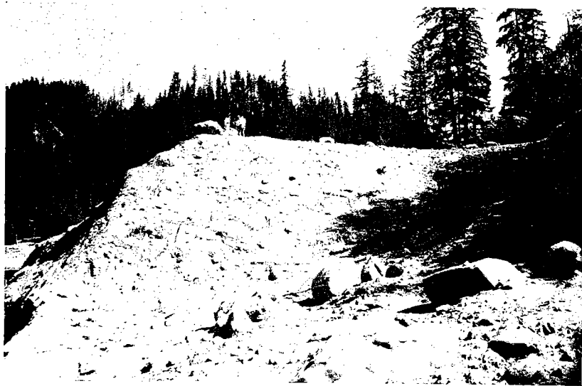
Figure 8. Large boulders deposited on a bridge abutment by mudflows southeast of Mount St. Helens.
