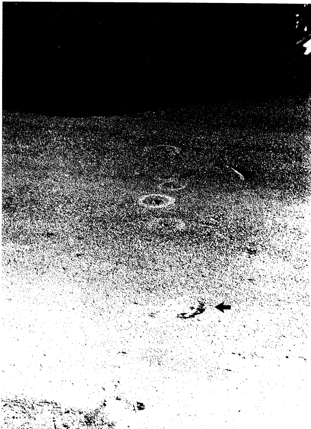
Figure 11. Impact marks on Highway One at northern end of Waddell Bluffs where large rock bounded onto roadway. Rock was present on shoulder and weighed approximately 350-400 lbs.
