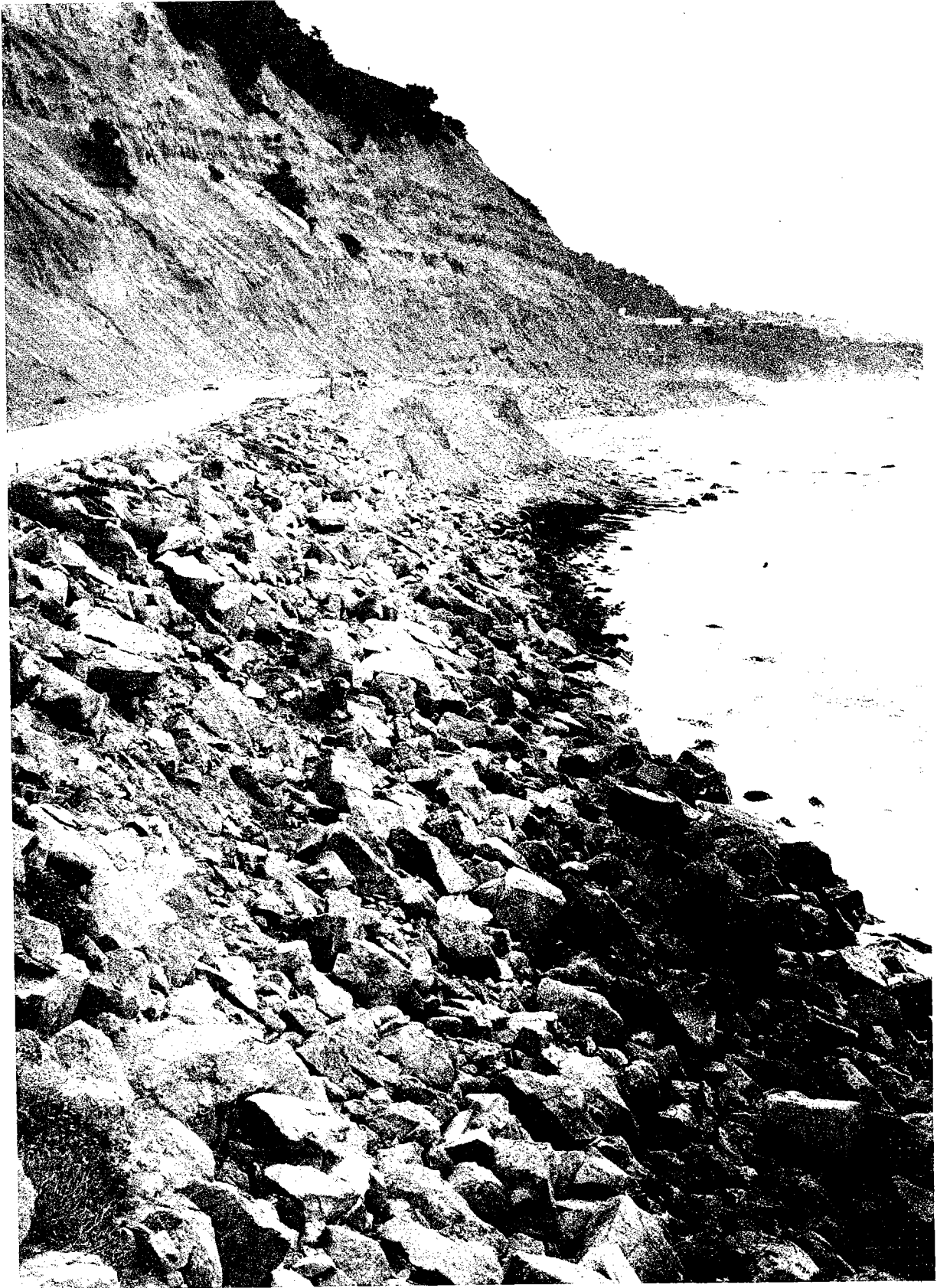
Figure 12. Initial riprap emplaced in 1947 to protect eroded area downcoast from natural groin. Some settlement has occurred. View downcoast.
