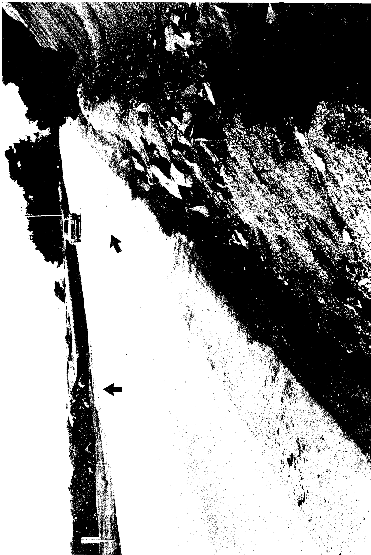
Figure 10. Debris trench at north end of bluffs. Almost no trench exists and rock is reaching traveled roadway. Note tracks crossing road (arrow) and recently dumped rocks on shoulder (arrow).
