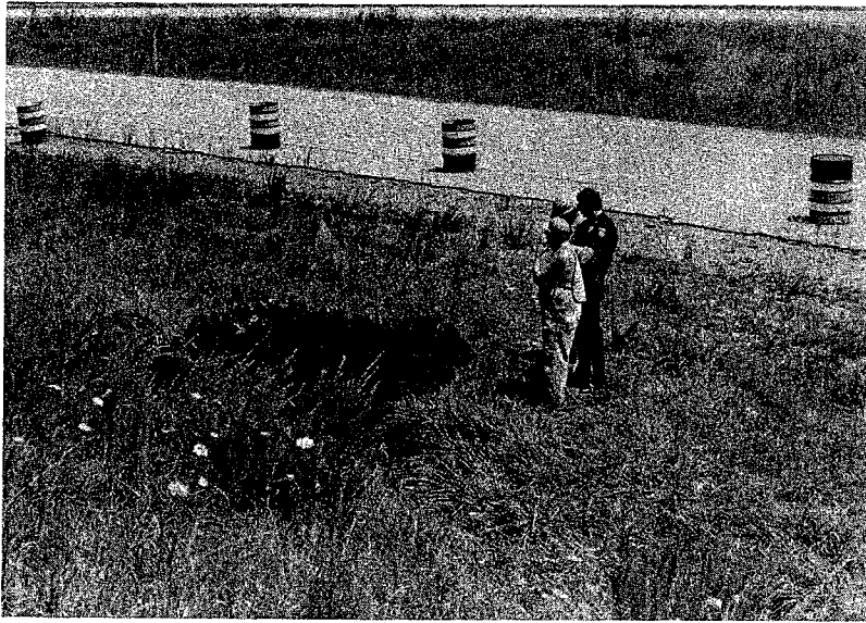
Figure 5. An unpaved ditchline resulted in this collapse along S. R. 73 in Maryville, Tennessee.
