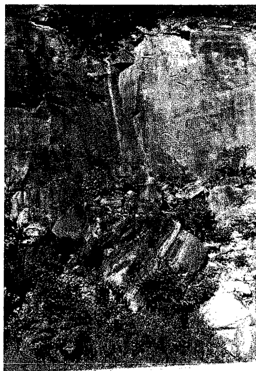
Figure 5: Shallow wedge failure at Mingo Junction cut. Notice the large rock blocks in the foreground.
