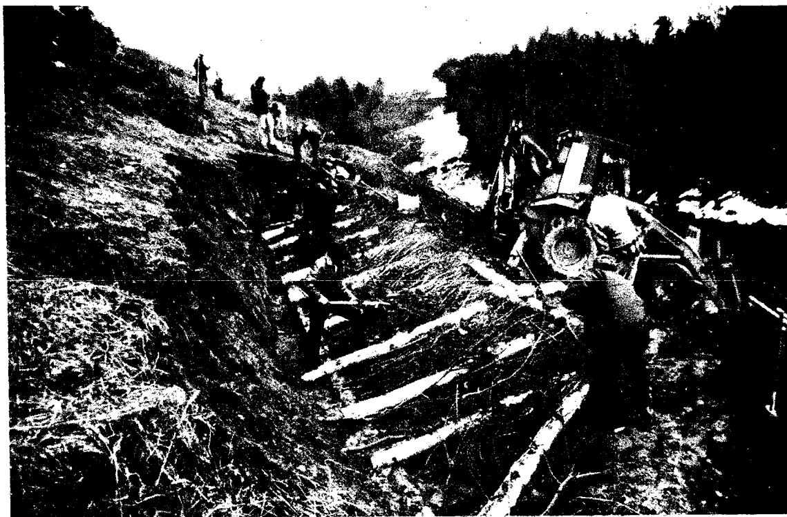
Photo 4. Close-up of live cribwall construction
