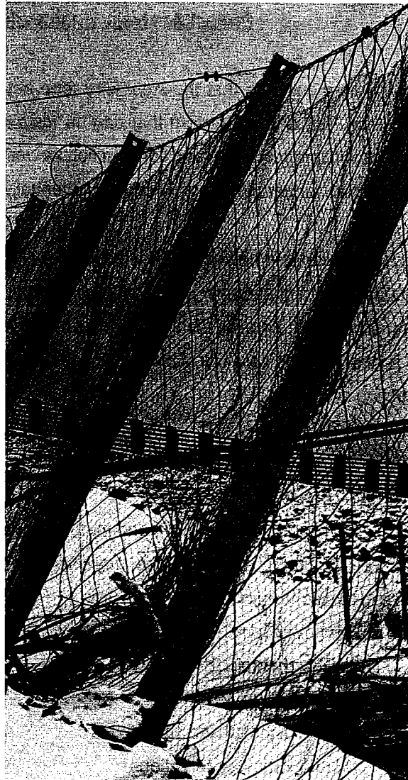
Picture 4 - Rockfall fence system with breaking devices
