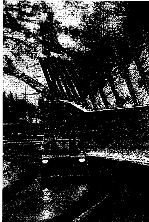
Figure 2 - Wire rope net support structure
