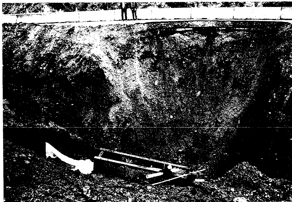
Figure 11. Caving Of The Roadway At The South Receiving Pit
