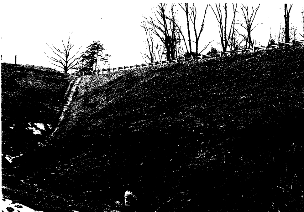
Photo 3. Area 1: slump failure - live cribwall construction; January 1987
