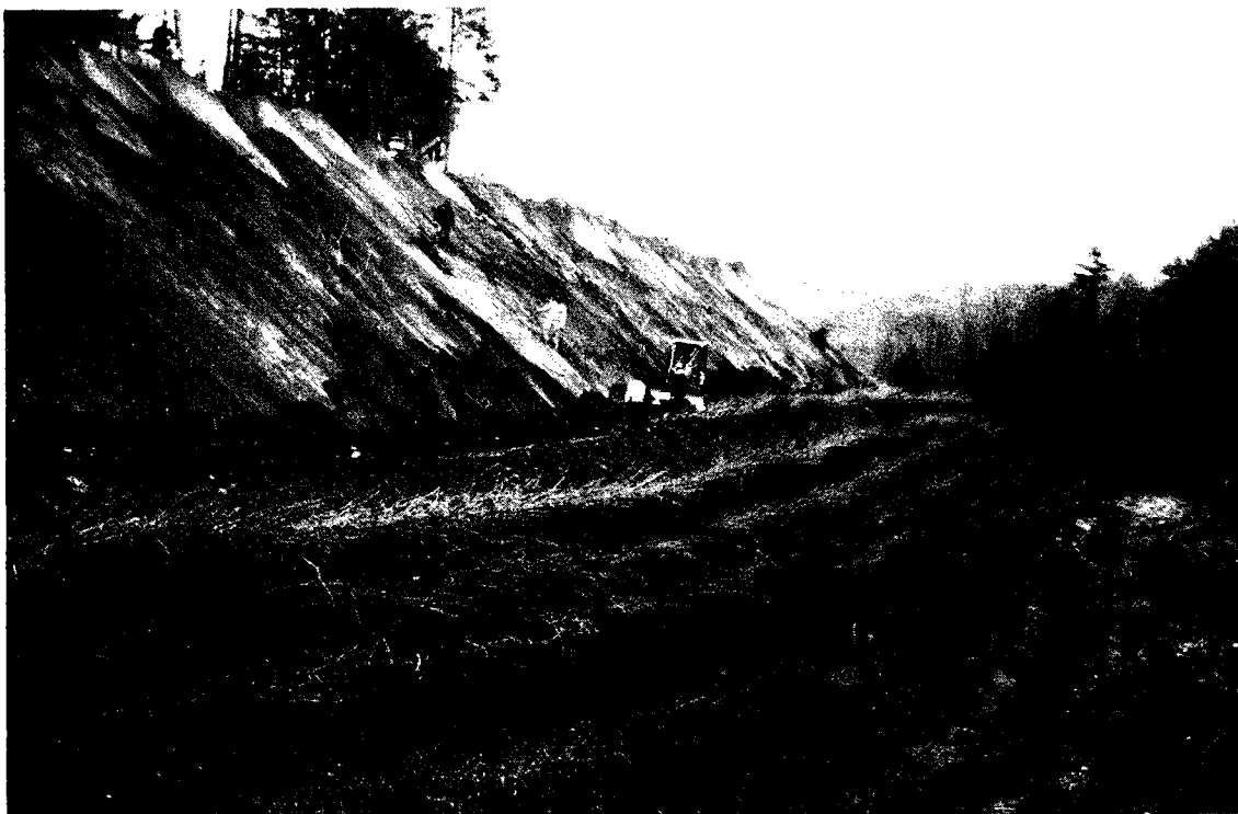
Photo 8. Area 2: February 1987, during fill brushlayer construction
