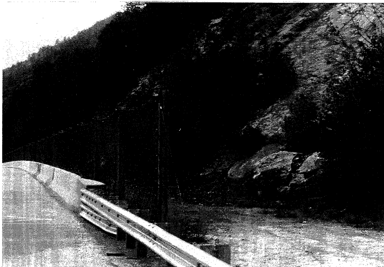
Tennessee DOT - I-40 Rockfall Catchment Barrier
