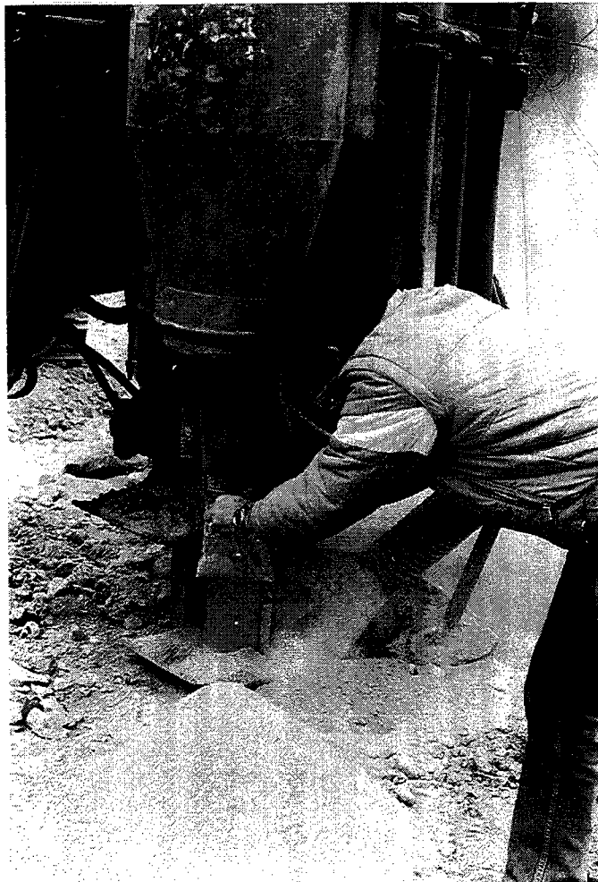
Fig.2 Sampling production drill cuttings for acid/base testing during construction.
