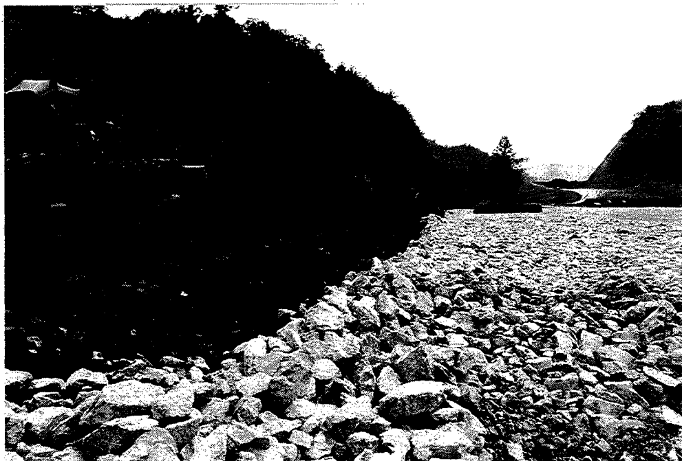
Fig.3 Construction of the clay liner encapsulation method showing limestone drainage pad and early stages of clay liner construction.
