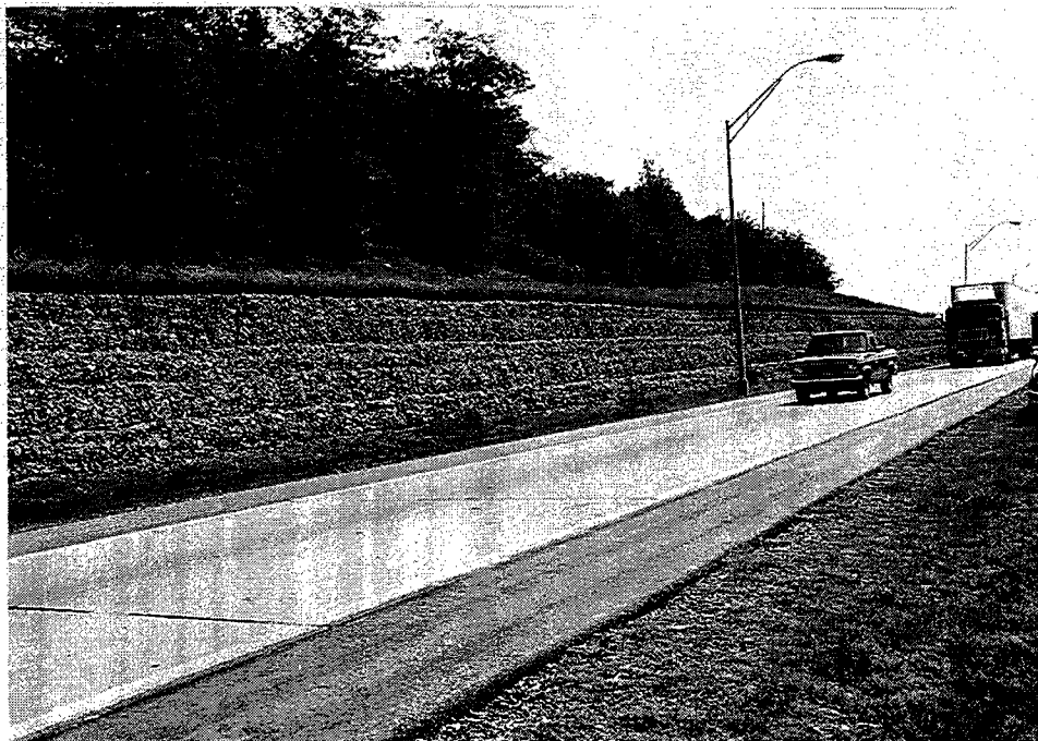
Figure 6 A. -- Gabion wall at exit 10 on I-540 in Fort Smith.
