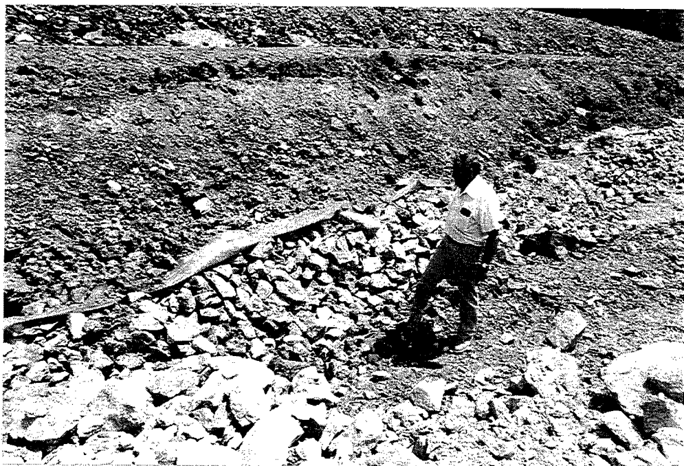
Fig.4 Side view of clay liner encapsulation during construction showing rock drainage pad, filter cloth and compacted clay liner.
