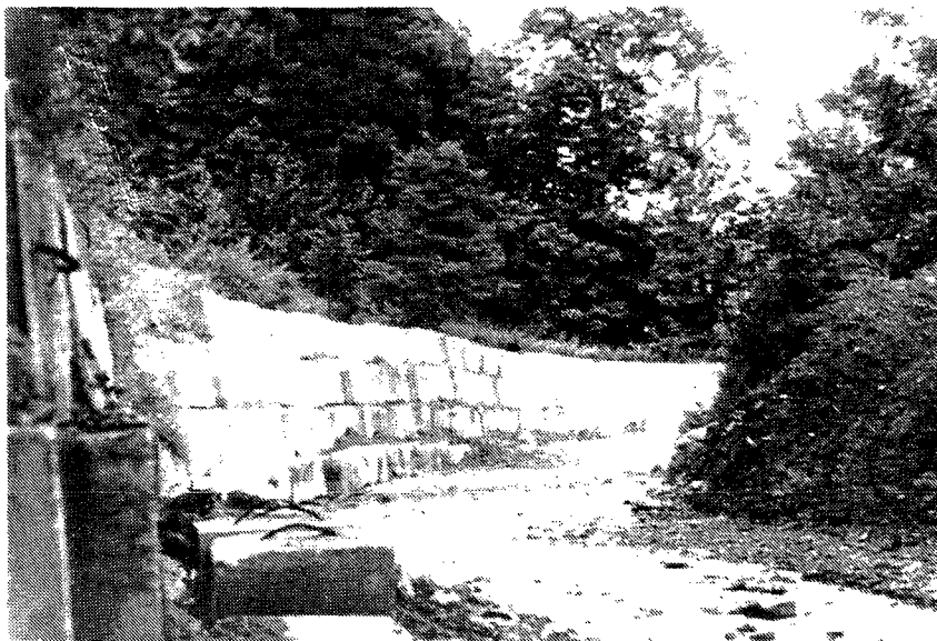
Figure 14: Concrete-block gravity retaining wall at the base of the slope at the Clough Pike site.
