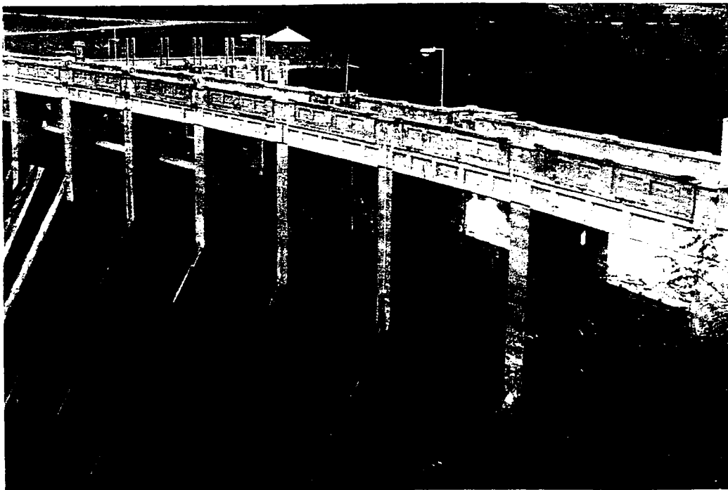
PHOTO 4 - DAM CREST WITH FLASHBOARDS
