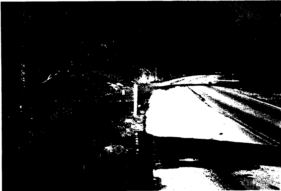
Figure 6: Sediment choked drainage ditch, which has forced water to drain over Chagrin River Road.
